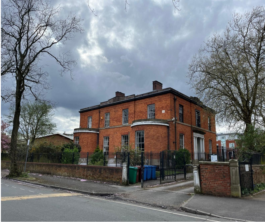
Figure 4.5: Court Nursing Home (grade II)
