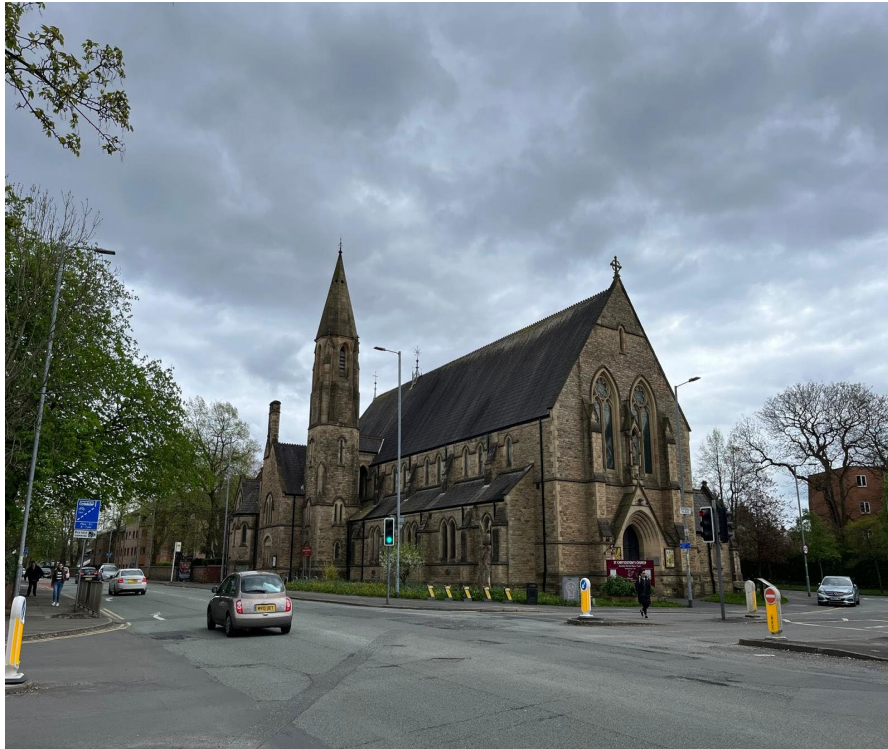
Figure 4.10: Church of St Chrysostom (grade II)
