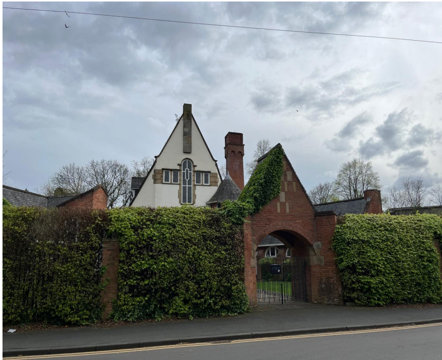
Figure 4.9: Former First Church of Christ, Scientist (grade I) and Arched Gateway (grade II)
