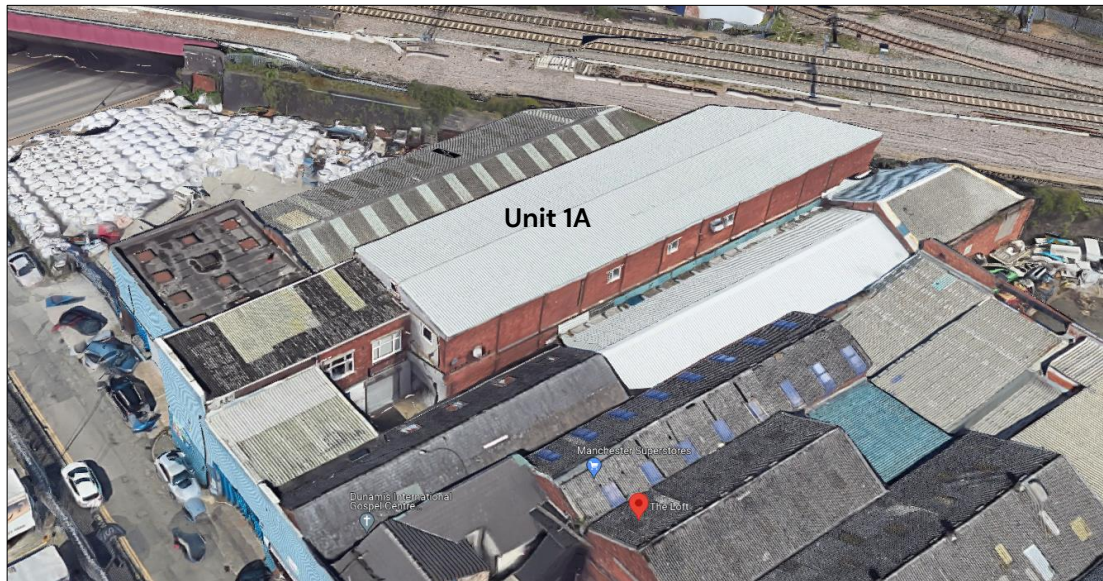
Figure 2.1: View of Unit 1A looking North East
