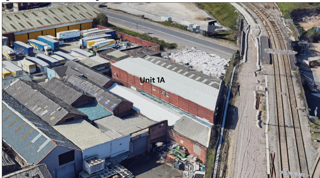
Figure 2.2: View of Unit 1A looking North West
