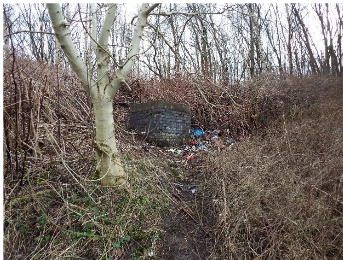
Blue brick stack/ manhole cover
