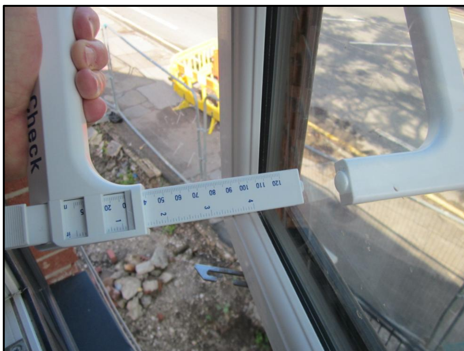
Photograph 5. Measured thickness of the sealed unit glazing, plot 10 - front bedroom
