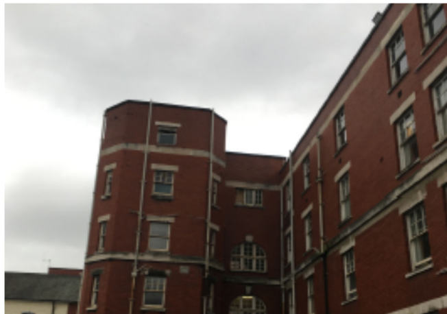
Figure 1.9: The rear service core to Cobbett House with contrasting brickwork and window details above the ashlar string course.
