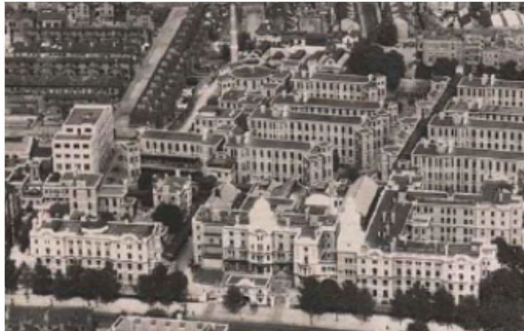
Figure 1.3: Post WWII damage, the left link between the central and northern ranges is missing, the scale of the complex extends well back to the rear of Cobbett House.
