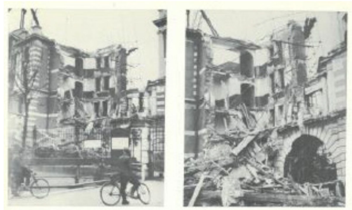
Figure 1.12: Images of the front, northern tower collapsing following WWII bomb damage (Brockbank, 1952).
