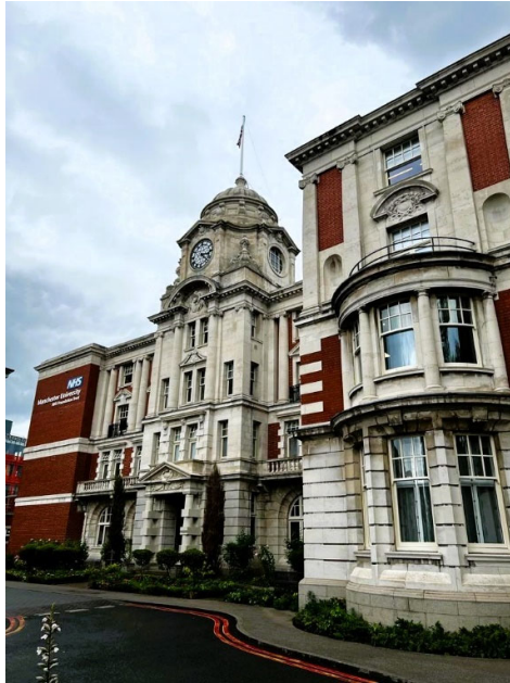
Figure 1.10: Facade of Cobbett House North at present indicate the extension after the WWII bombing.
