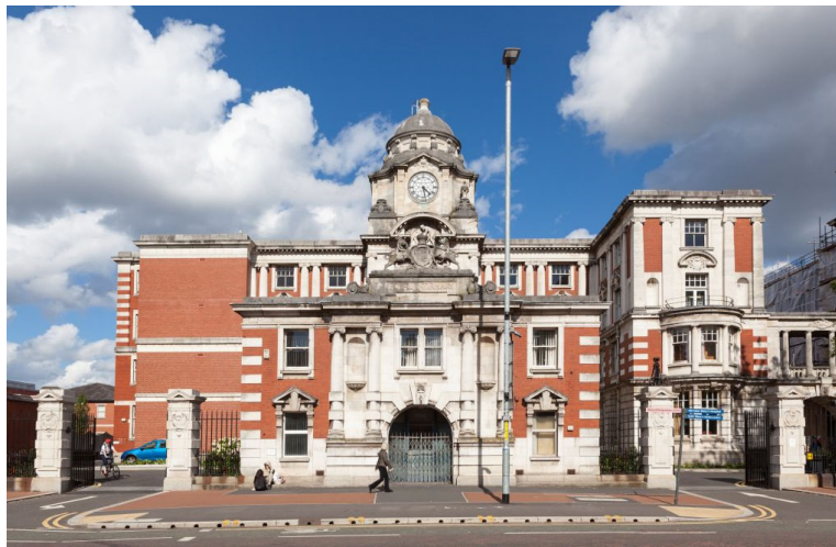
Figure 1.14: The left-hand bay removed following WWII.
