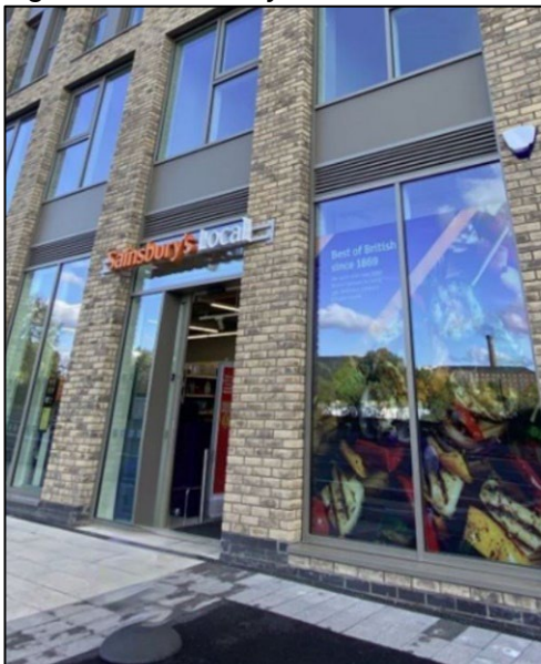
Figure 1: Sainsbury's Local Old Mill Street.
