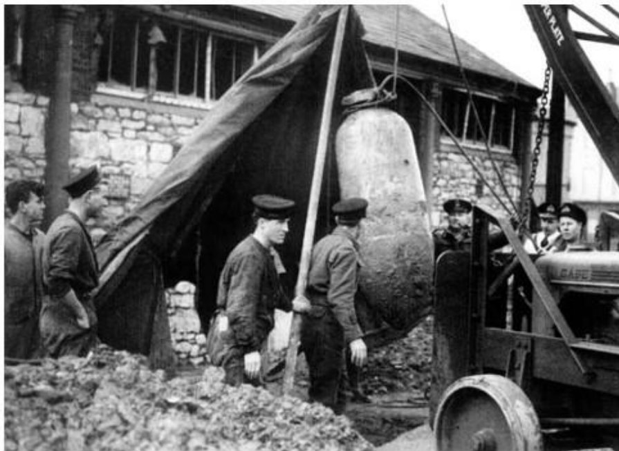
Removal of an UXB
