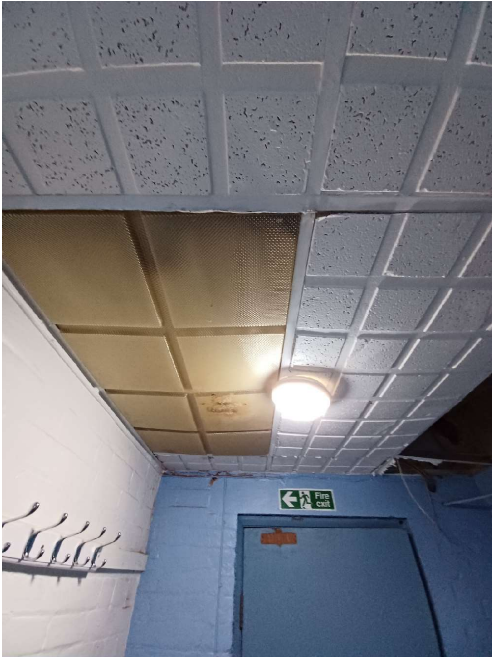
Replace all ceilings and Lighting
