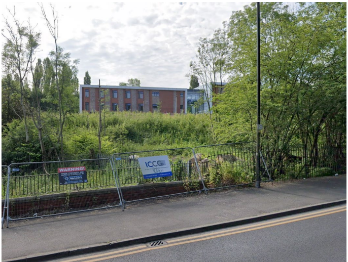
2 View from Delaunays Road towards the Crumpsall HC
