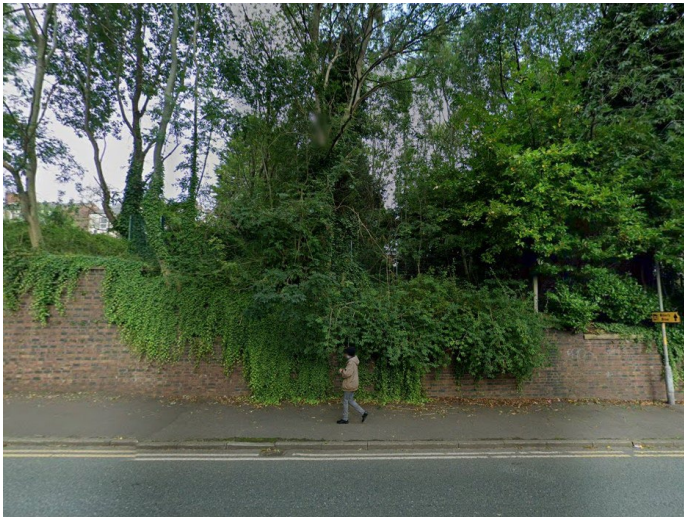
3 View of Delaunays Road retaining wall
