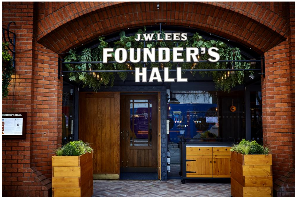
Photograph 6 – As-built internally illuminated individual letters fascia sign to main entrance.
