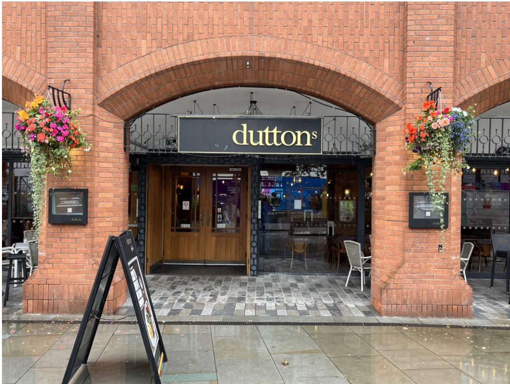
Photograph 2 – Existing internally illuminated fascia sign (nr2) above main entrance and 2 nr internally illuminated menu boxes to brickwork columns to both sides of main entrance all now removed.
