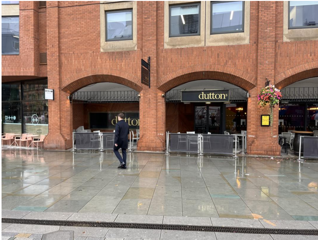
Photograph 1 – Existing internally illuminated fascia sign (nr 1) above fire exit entrance and projecting sign (nr 1) all now removed.
