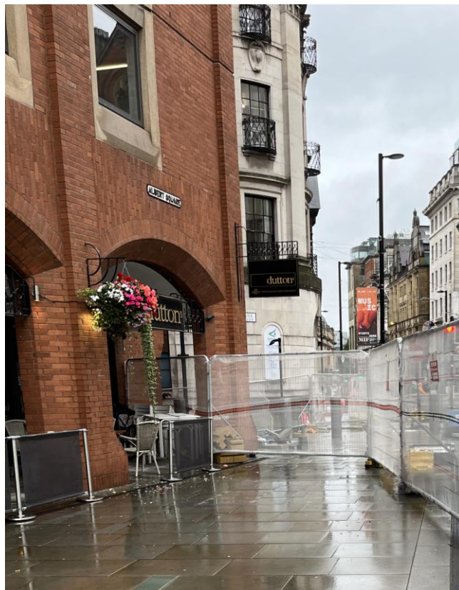
Photograph 3 – Existing internally illuminated fascia sign (nr 3) and projecting sign (nr 2) all now removed.
