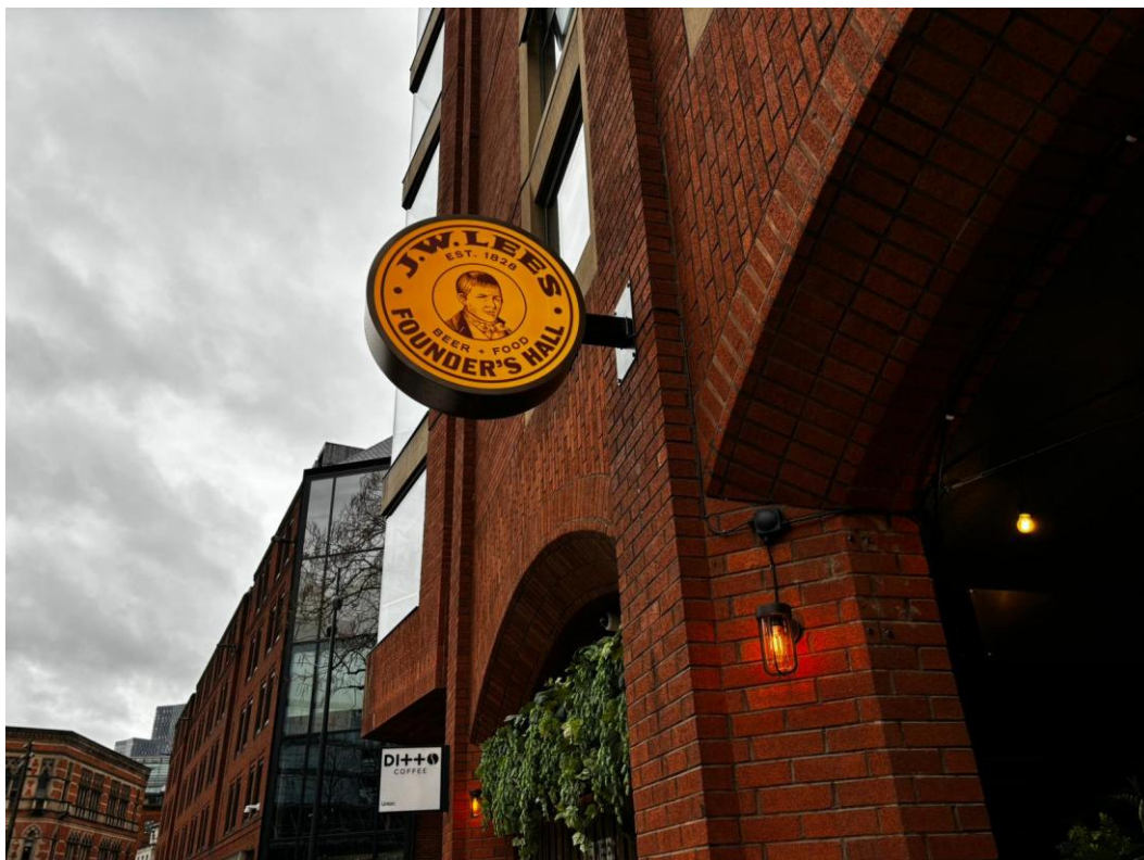
Photograph 5 – As-built internally illuminated projecting sign (nr 1).
