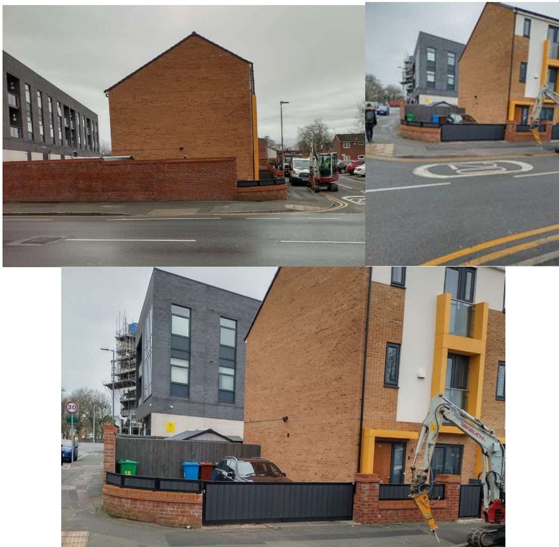
Fig.1 – View of the application site from Brunswick Street and Beamish Close
