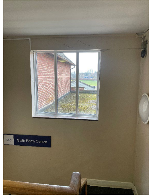
Figure 105: Window to west elevation, lighting stairwell.
