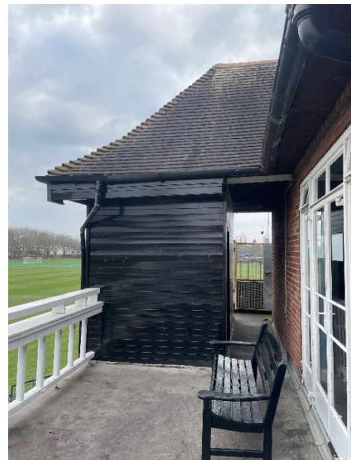
Figure 125: View of the first floor terrace, orientated west. Timber with the projecting bay for the scores to be hung out at the end.
