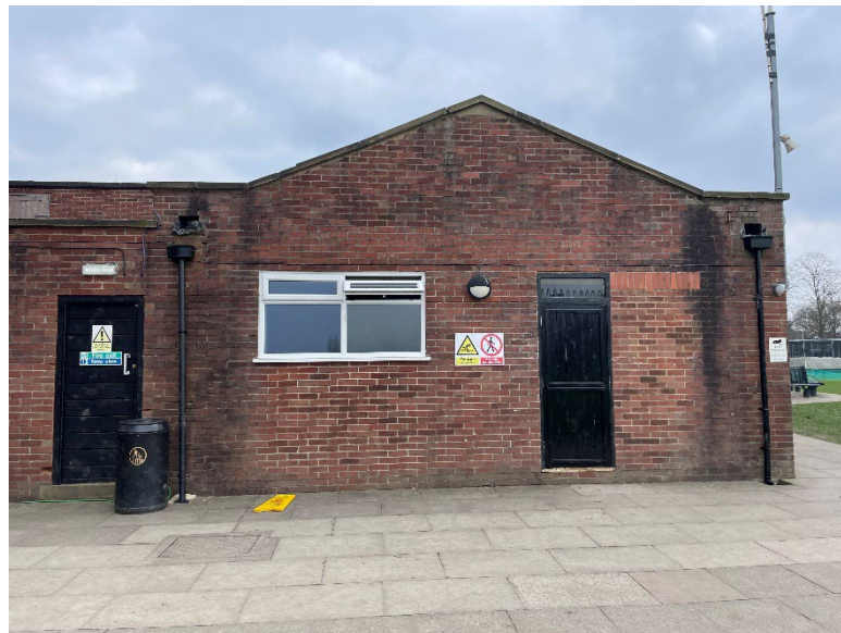
Figure 35: View of the east elevation. Brown brick in stretcher bond. Single pitched roof, modern replacement upvc windows. Two utilitarian timber panelled doors feature.
