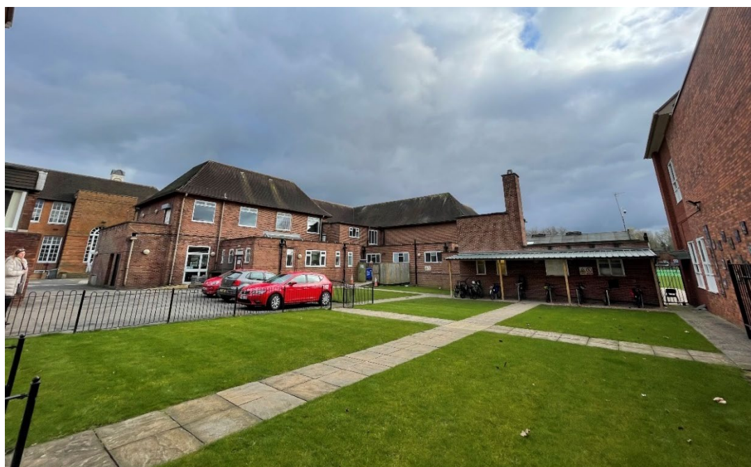
Figure 29: View of the north and west elevations of the pavilion illustrating the utilitarian appearance of the 'back' of the building. Original bellcast / sprocketed eaves and clay roof tiles feature to 2-storey elements. Note modern, replacement windows and doors. The block to the far right (west) comprises the toilet / plant room block. Later veranda fixed to north elevation.
