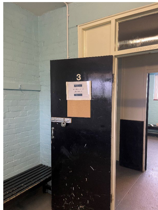
Figure 73: Changing room 2.3, south side (centre). Original door and architrave.
