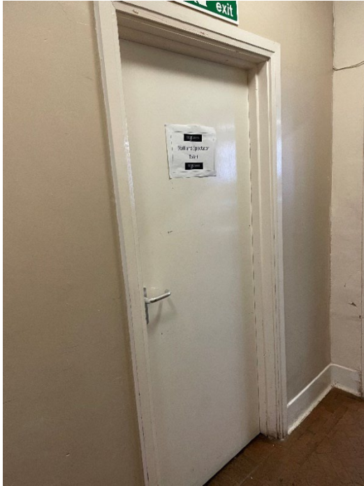
Figure 47: Room 8, toilet (inaccessible), west side of corridor.
