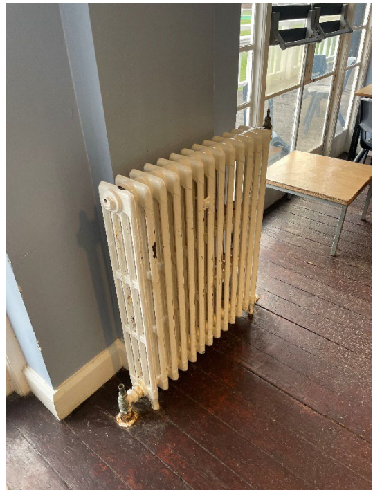
Figure 119: Example of original 1950s radiator. Original timber flooring.
