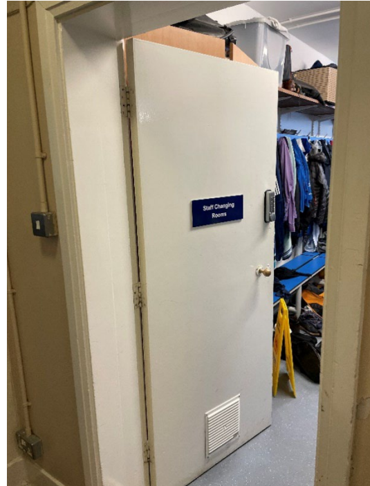
Figure 48: Room 5, Staff changing room. Original brass door handle. Utilitarian 1950s door and recessed architrave.
