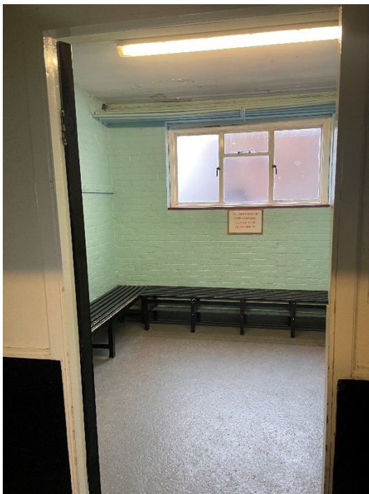
Figure 68: Changing room 2.2, north-east corner. Original tripartite window with brass latches. Brick walls overpainted blue.
