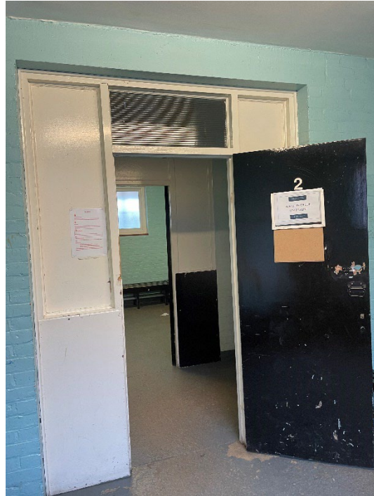
Figure 71: Changing room 2.2, north-east corner. Original 1950s door and architrave. Flanking windows boarded over. Ribbed glass to central light above.
