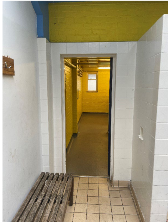
Figure 91: Shower room, Room 3 on GF plan (looking north into toilet area). Note, inbuilt soap dish in wall to right wall.
