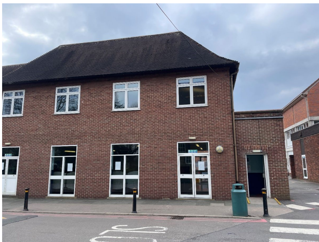
Figure 23: East elevation, north side. Brown brick in stretcher bond, original bellcast / sprocketed eaves and clay roof tiles. Replacement upvc windows / modern doors across the elevation. Single storey lean-to with flat roof to north.
