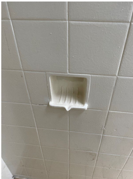
Figure 92: Detail of inbuilt soap dish.
