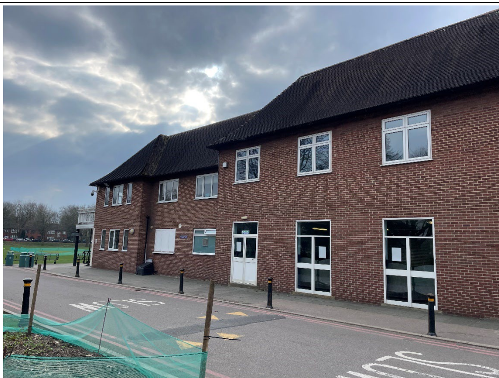
Figure 24: East elevation, south side. Brown brick in stretcher bond, hipped clay tile roof and replacement upvc windows / modern doors across the elevation. Recessed section and slight projecting bay to southern end.
