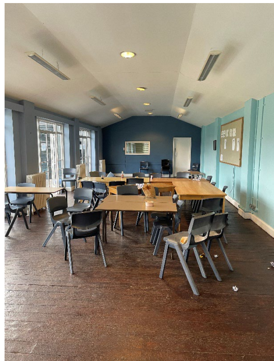
Figure 115: View of the linear room to the south aspect of the building. The doors to the left provide access out on to the terrace. Metal framed windows/doors, timber board flooring and radiators are original / 1950s.
