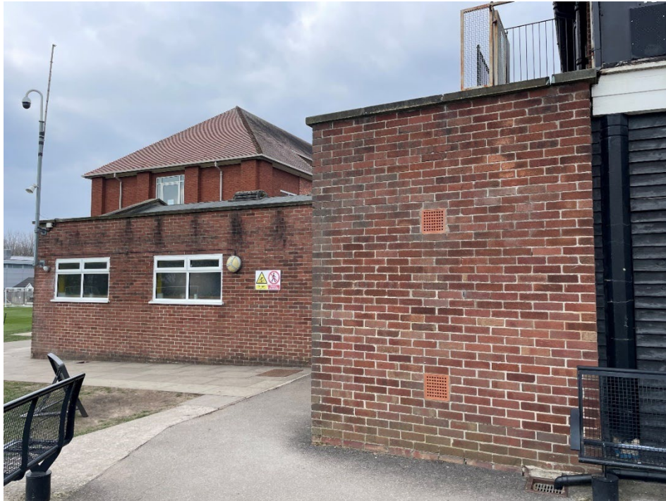
Figure 14: South elevation, single storey – western aspect. Section to the right of the image is illustrative of the external stair, single-storey building recessed to the left is the dining hall. Traditional mid-20 th century brown brick in stretcher bond. Windows to the left of the image are shown to have been replaced with upvc.
