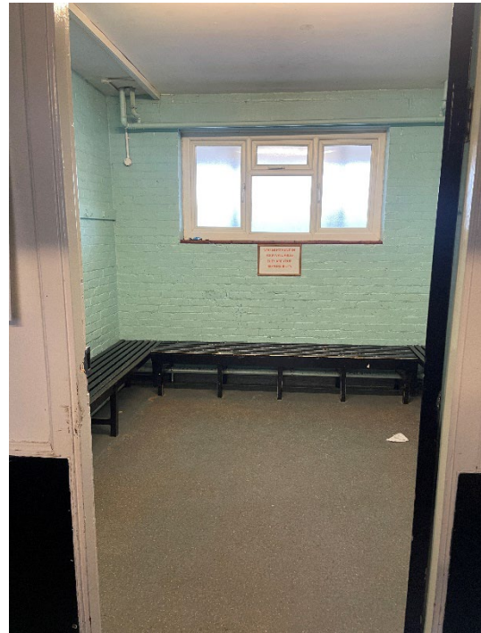
Figure 65: Changing room 2.1, south-east corner. uPVC replacement window to south elevation.
