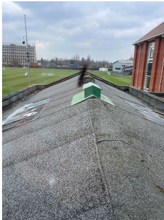
Figure 34: Asphalt roof covering over dining hall. View looking west from first floor window.
