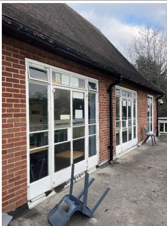
Figure 126: View of the first floor terrace, orientated south-west, allowing for view of 1950s metal framed windows to south elevation.
