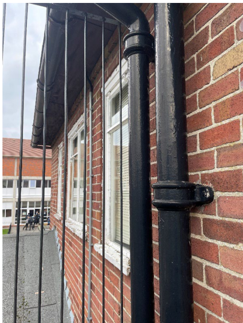
Figure 15: External rainwater goods detail (north / west elevation).
