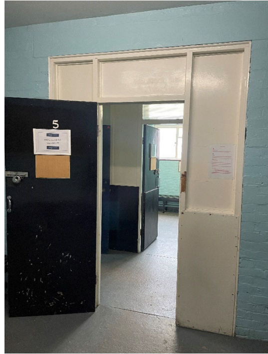
Figure 79: Changing room 2.5, south-west corner.
