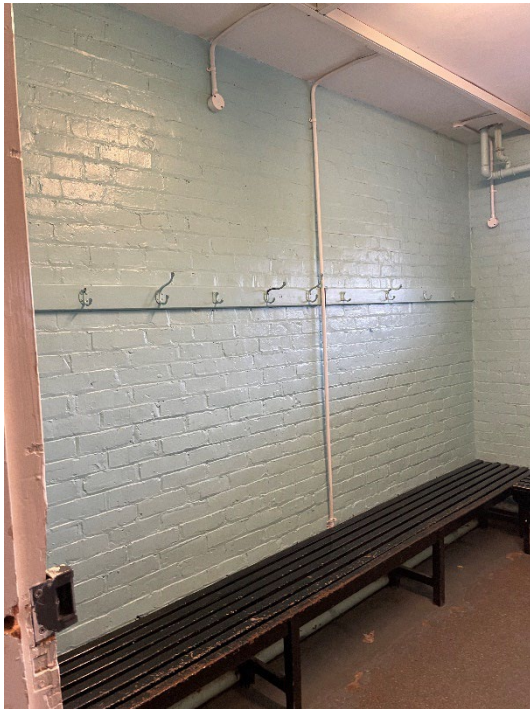
Figure 66: Changing room 2.1, south-east corner. Fixed bench seating to each side. Brick walls overpainted blue. Original fixed hooks.
