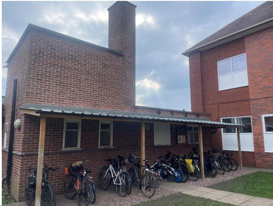
Figure 32: View of the north elevation of the pavilion (west side), brown brick in stretcher bond, featuring chimney. Original casement windows. Later veranda fixed to north elevation.
