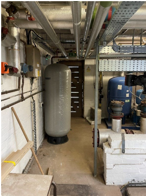
Figure 99: Room 14, north-west end of floorplate. Plant room, looking west to timber door (external).
