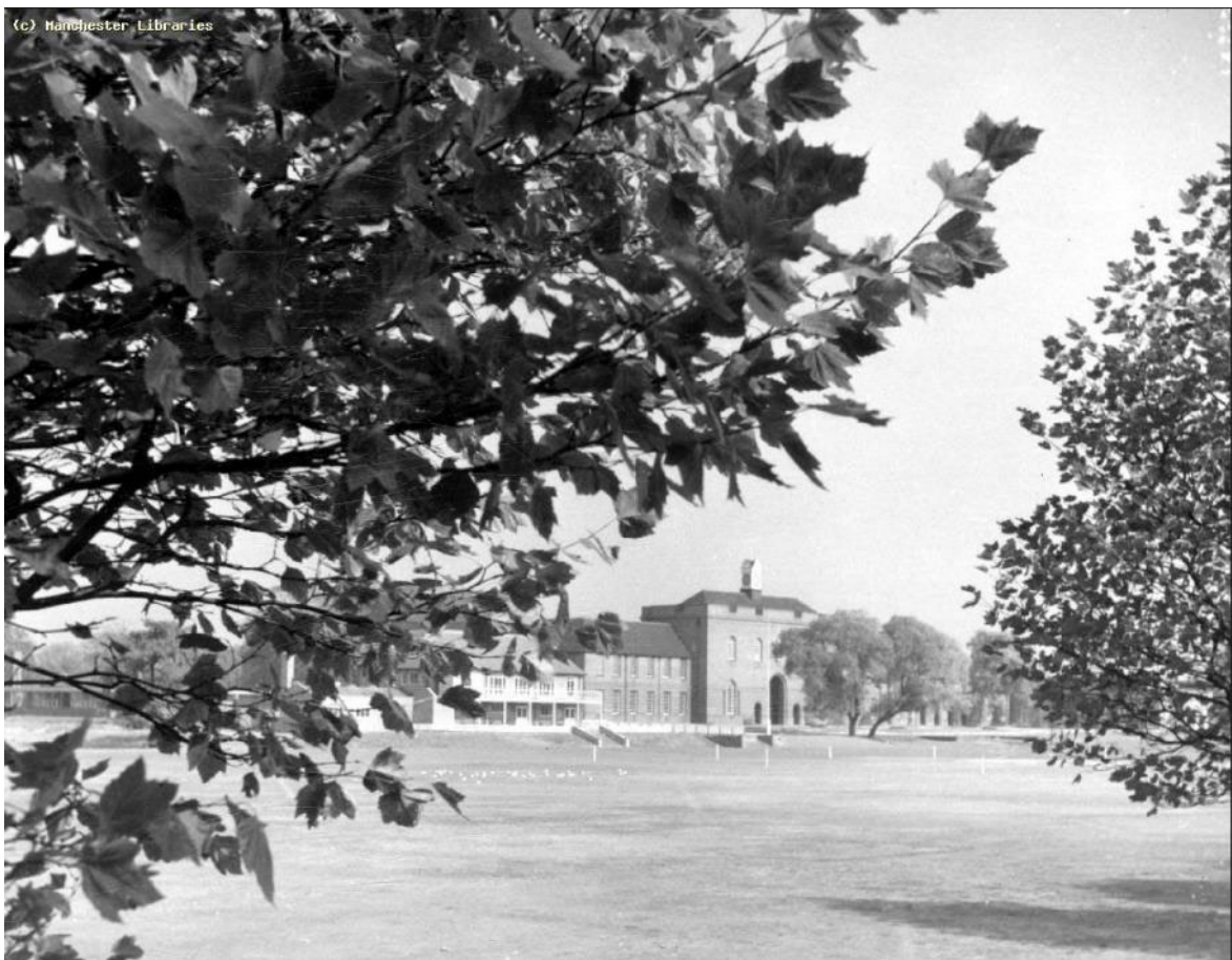
Figure 10b: The Pavilion in 1959. Source: Manchester Image Collection
