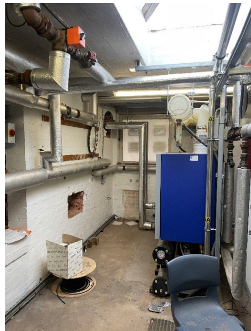
Figure 100: Room 14, north-west end of floorplate. Plant room, looking north.
