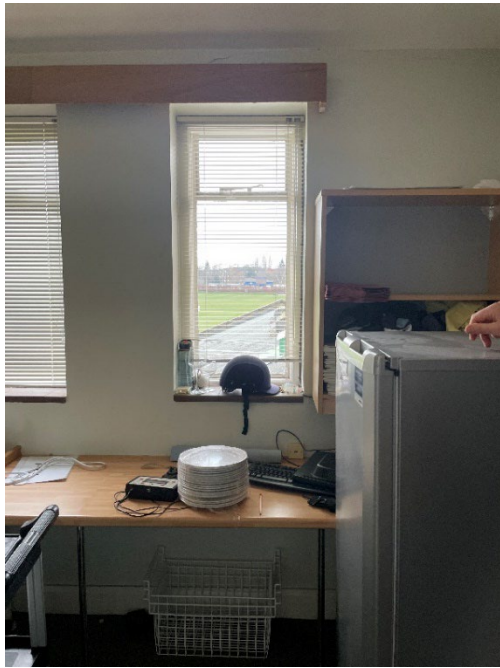
Figure 122: Room, west end of floorplate (looking west). 1950s windows with casement light above, original cills.
