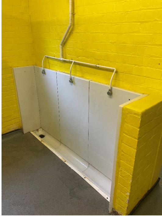
Figure 93: 1950s inbuilt urinal, south wall to NW toilet room.
