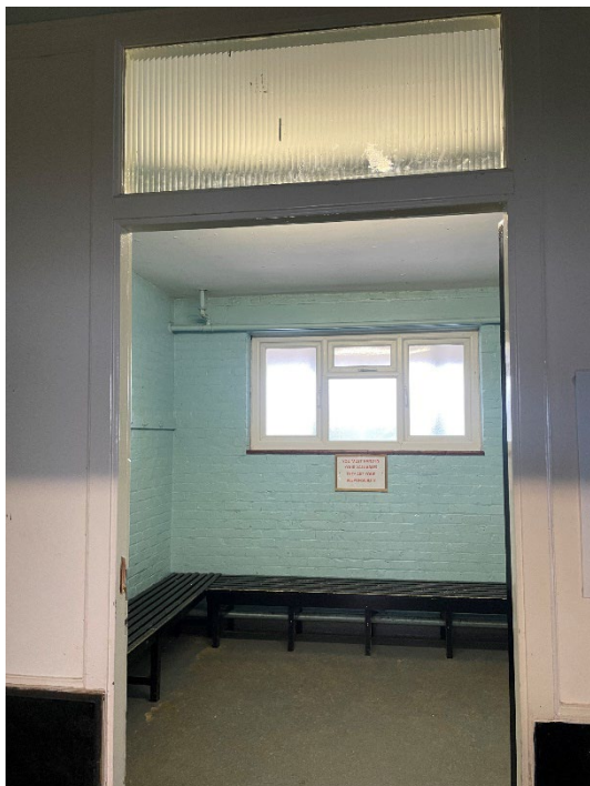
Figure 72: Changing room 2.3, south side (centre). Replacement window, Upvc. Brick walls overpainted blue.
