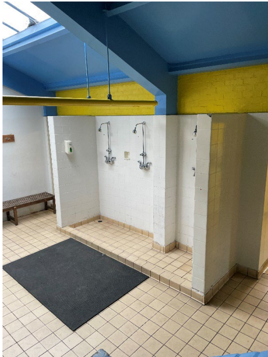
Figure 86: Shower room, Room 3 on GF plan (looking north-west). Open shower enclosure, partial height.
