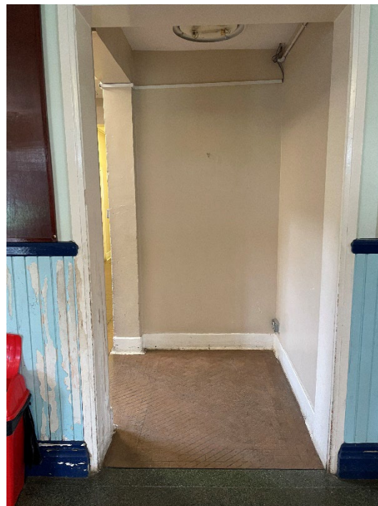
Figure 43 (left): Memorial plaque for T. F. Nutter, situated to NE corner of room 1. Figure 44 (right): Room 1, looking north into corridor. No doors. Original plain skirting and woodblock flooring.
