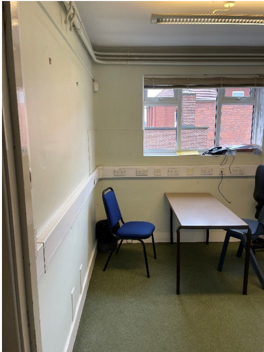
Figure 108: Room north of stairwell, first floor. Modern trunking and replacement window.
