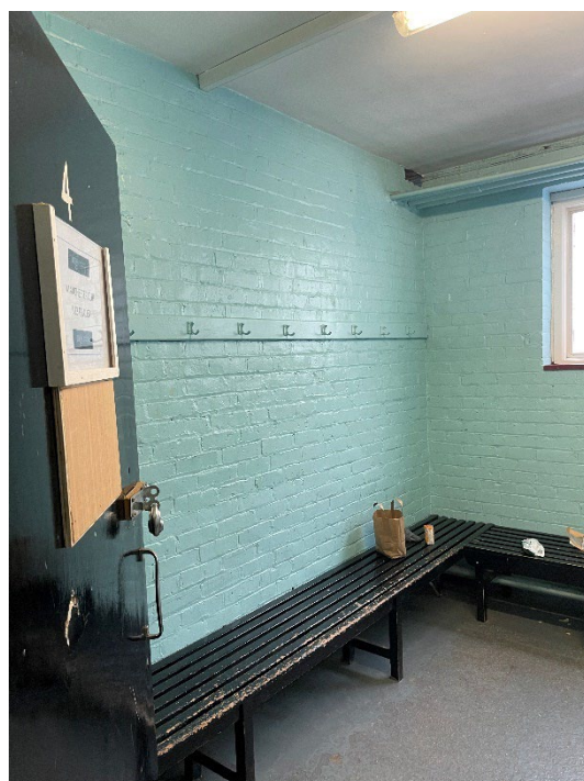
Figure 75: Changing room 2.4, north side (centre).
