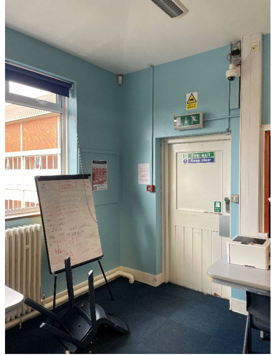
Figure 113: Large sixth form classroom, north aspect of the first floor plan. Original timber paneled door (glazing overcovered).
