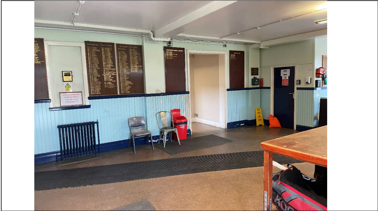
Figure 36: Room 1, looking north-east. Entrance hall with wooden honour boards, with gold lettering, featuring to each wall. Timber panelling to dado height, overpainted in light blue. Dark blue paint applied to original dado and moulded skirting. Original woodblock floor and green terrazzo to perimeter.
