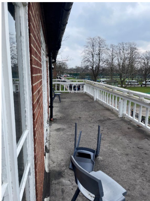
Figure 124: View of the first-floor terrace, orientated east.
