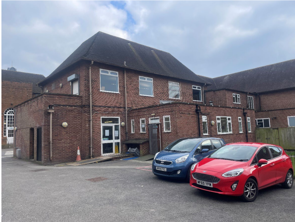
Figure 30: View of the north and west elevations of the pavilion. Note modern, replacement windows and doors. Original bellcast / sprocketed eaves and clay roof tiles feature to 2-storey elements.
