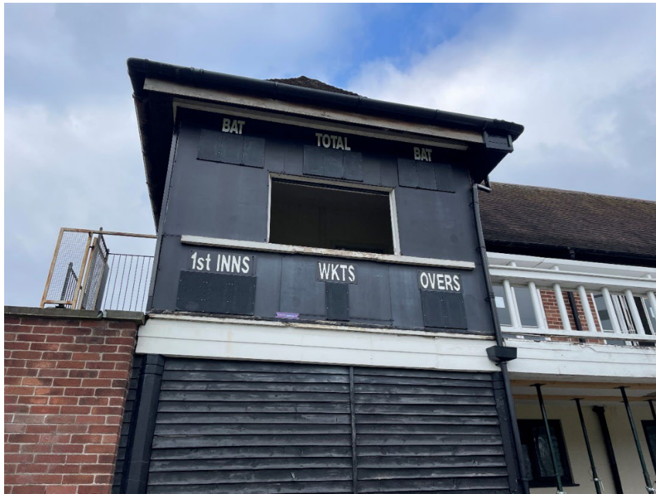
Figure 17: View of the south elevation illustrating the veranda to the ground floor and terrace above. The projecting bay contains a room and opening from which the cricket scores are hung. The timber cladded infill and central opening to the ground floor are alterations. The original windows and door have also been altered and replaced with modern double glazed units.
