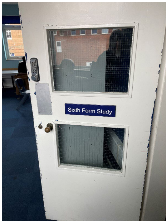
Figure 114: Original 1950s door leading into sixth-form classroom (north aspect of floorplate). Original brass handle. Georgian wire glass. Modern lock and door plate.
