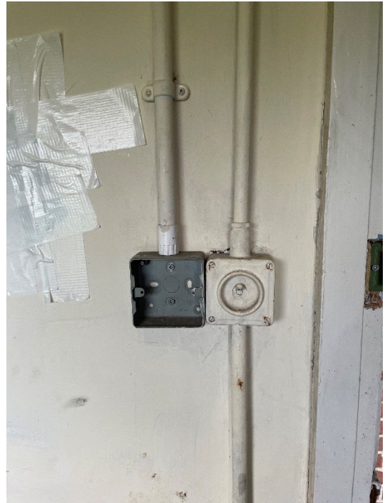
Figure 130: Interior of cricket score room. Original dolly light switch.
