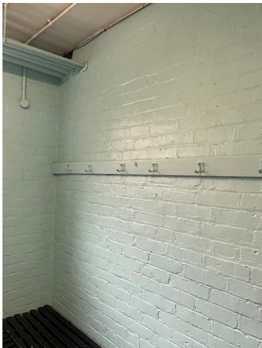
Figure 82: Changing room 2.6, northwest corner. Fixed benches and wall hooks.
