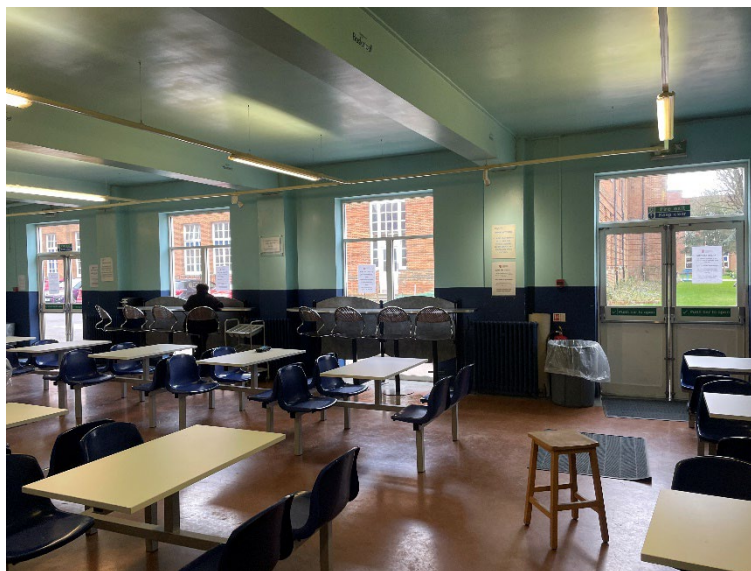
Figure 55: View of the ground floor canteen space to the east side of the building (orientated to north-east aspect of the space). Modern doors and window lights above. Modern lighting / M&E.
