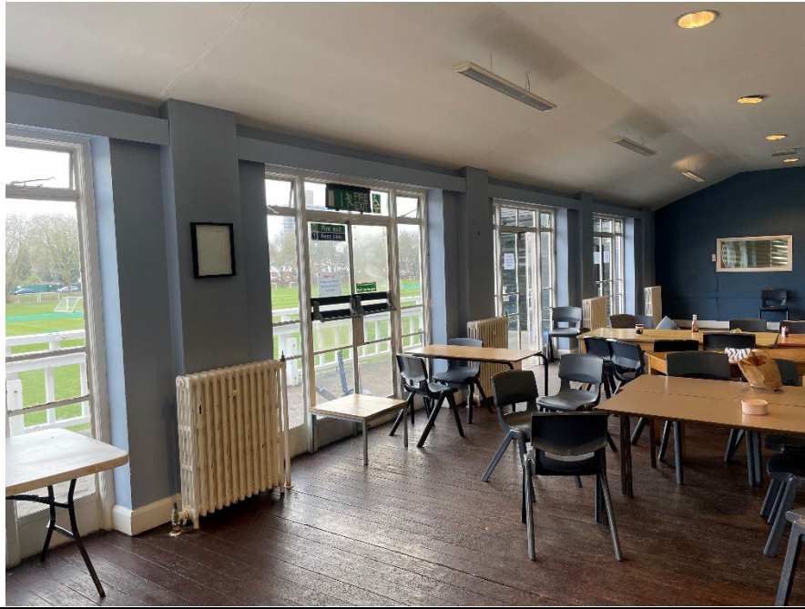
Figure 116: View of the linear room to the south aspect of the building. The doors to the left provide access out on to the terrace. Metal framed windows/ doors, timber board flooring and radiators are original / 1950s.
