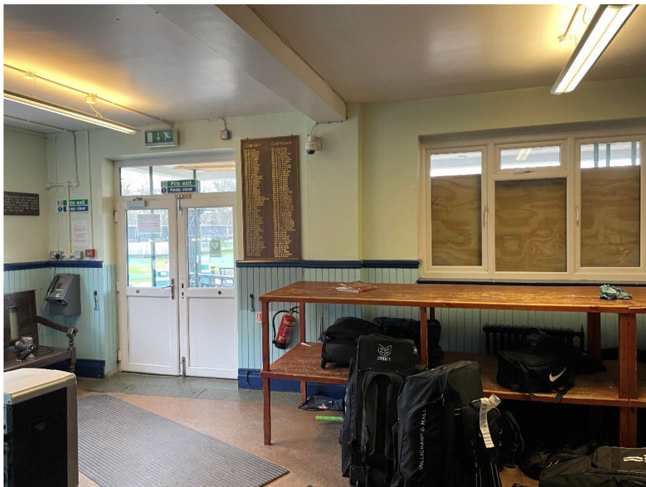
Figure 39: Room 1, looking south-east. Entrance hall with wooden honour boards. Fixed telephone to far SE corner. Replacement upvc windows and doors. Later M&E / lighting.
