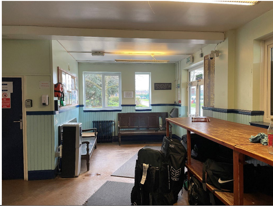
Figure 38: Room 1, looking east. Entrance hall with wooden honour boards. Replacement upvc windows and doors.
