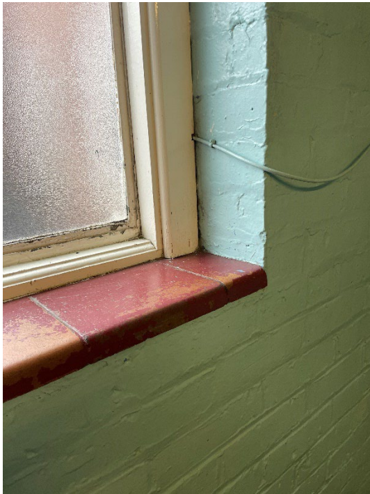
Figure 70: Changing room 2.2, north-east corner. Original window cill red / orange tile.
