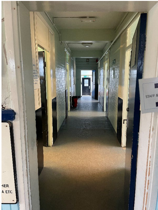
Figure 64: Corridor from Entrance Hall (Room 1), looking west towards changing room area. Original brick walls and concrete floor. Total of 6 changing rooms.
