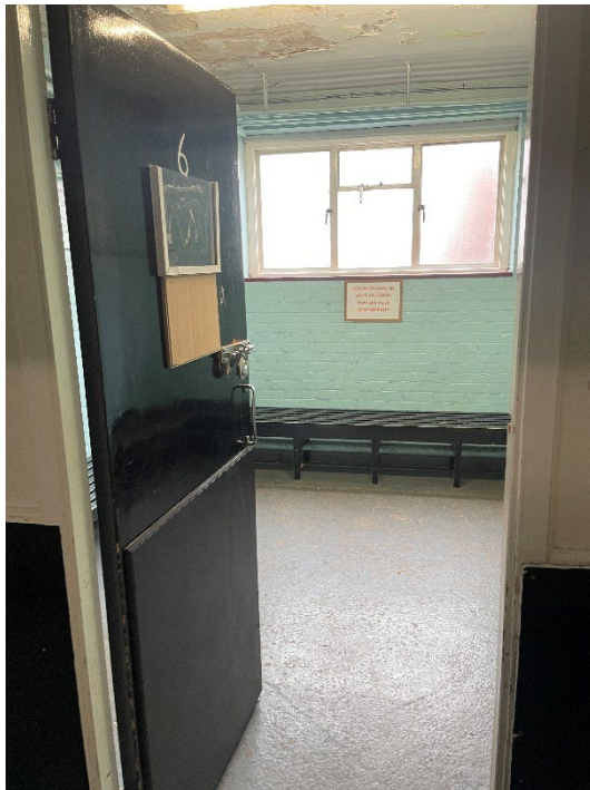
Figure 80: Changing room 2.6, northwest corner. Original tripartite window with brass latches. Brick walls overpainted blue.
