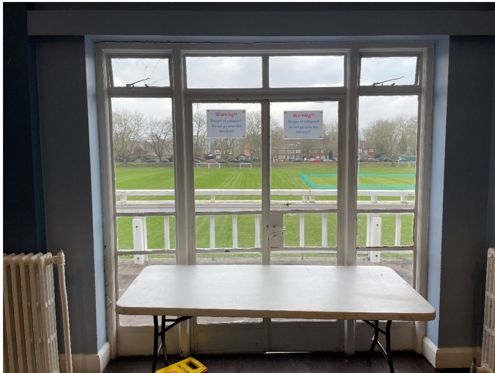
Figure 117: Detail of one of the metal framed doors from the linear, first floor room to the terrace, orientated south towards fields.
