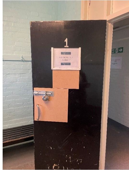
Figure 67: Changing room 2.1, south-east corner. Original door and surround, modern handle and lock.
