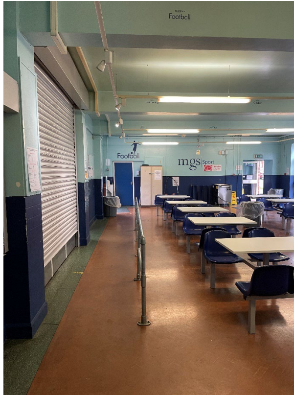
Figure 54: Room 6. View of the ground floor canteen space to the east side of the building, looking north across space. Walls part tiled (half height) to western wall, painted dark blue. Original woodblock floor and green terrazzo to perimeter. Roller shutter to west wall (kitchen behind) Fixed railing to west side of floorspace and fixed seating to centre.
