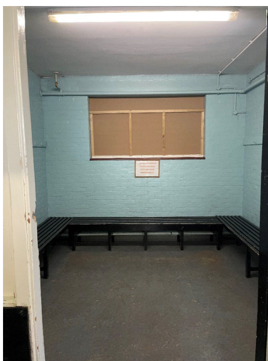
Figure 77: Changing room 2.5, south-west corner. Original tripartite window (overcovered). Brick walls overpainted blue.
