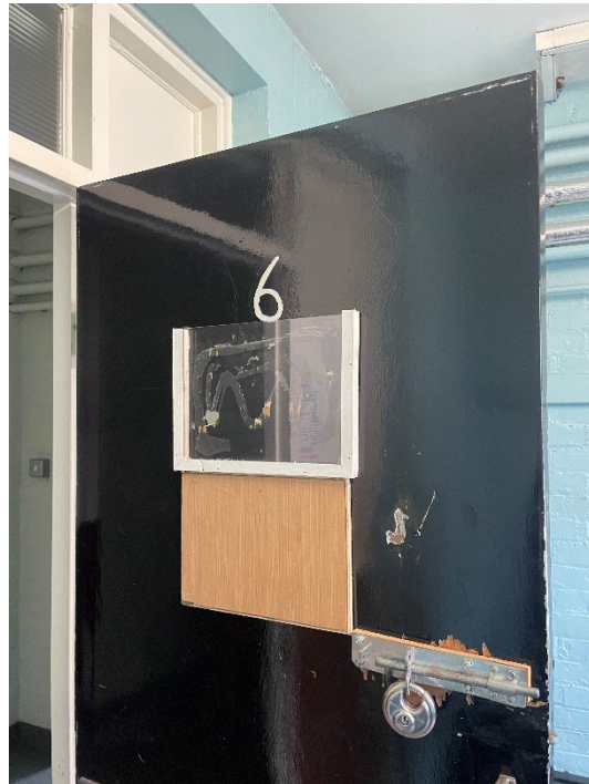
Figure 83: Changing room 2.6, northwest corner. Original 1950s door and glazed architrave (part covered over), with modern lock to door.
