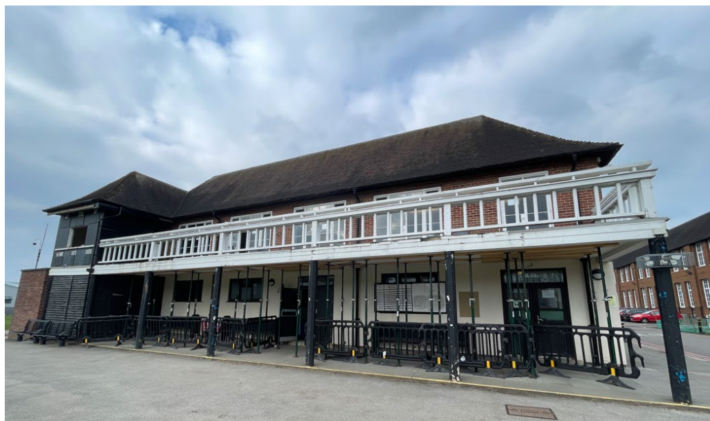
Figure 13: South elevation, illustrating the veranda to the ground floor and terrace above. The projecting bay to the left contains a room and opening from which the cricket scores are hung. The timber cladded infill and central opening to the ground floor are alterations. The original windows and door have also been altered and replaced with modern double glazed units. Bellcast / sprocketed eaves and clay roof tiles.
