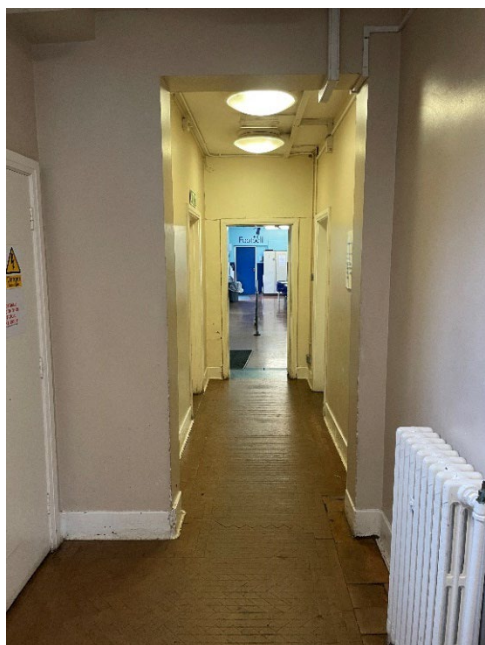
Figure 45 (left): North corridor leading from Room 1 into dining hall to the north. Original woodblock flooring, plain skirting and radiator. Figure 46 (right): Original door and brass handle, store cupboard (not accessible).
