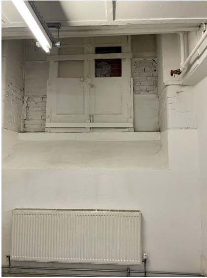
Image 7: Existing high level door. Bricked up behind.
