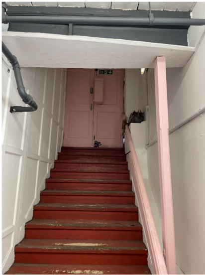
Image 1: Existing Entrance Stair
