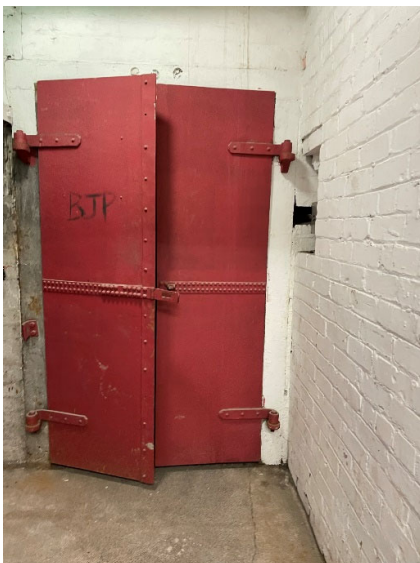
Image 4: Existing Rear doors to redundant Lift.
