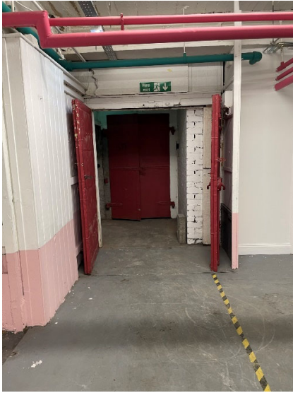
Image 5: View to rear escape route – looking at existing lift.
