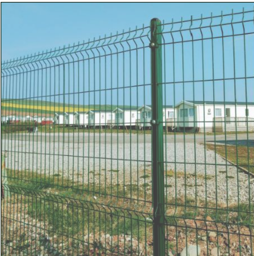
Indicative image of typical site boundary fence
