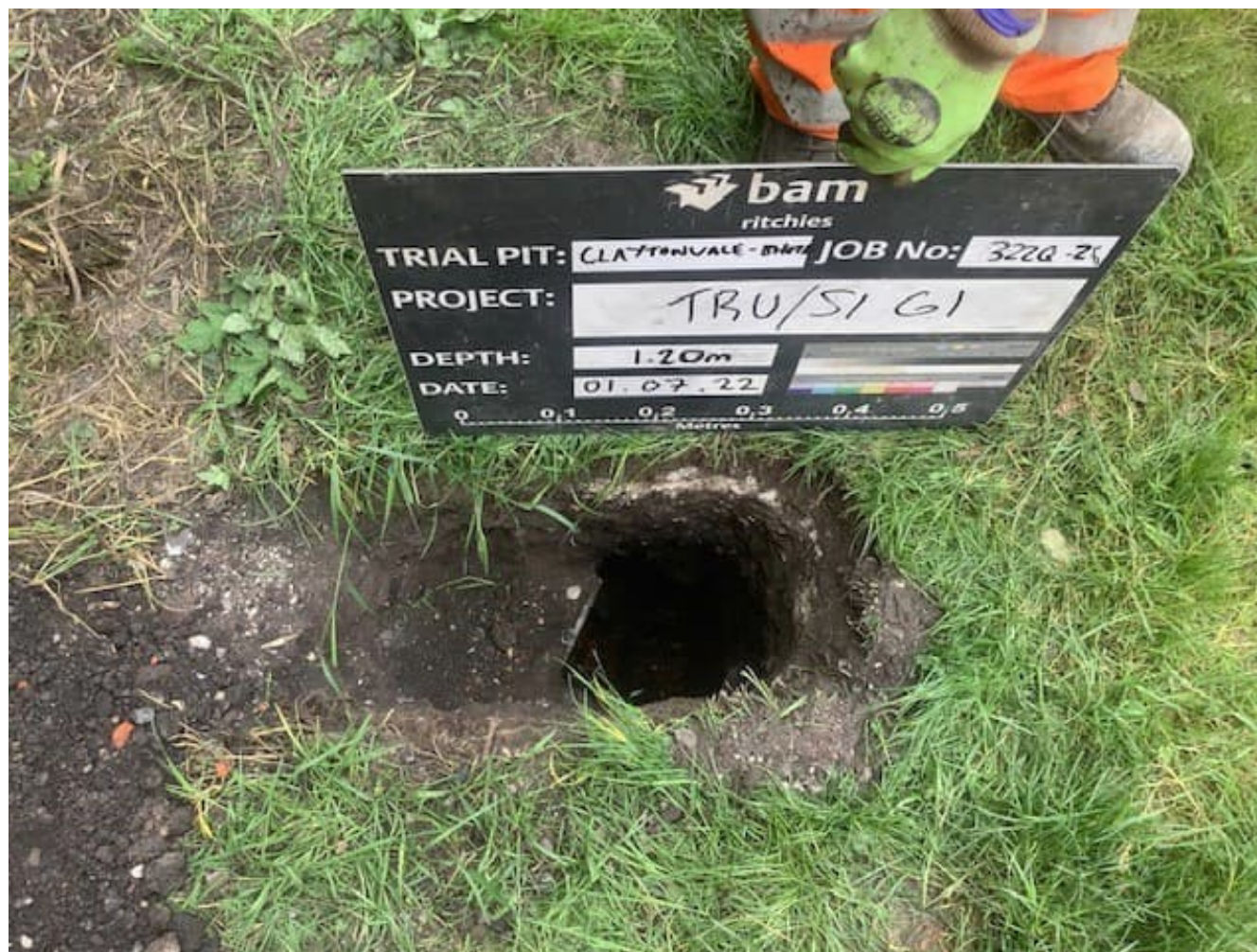
CLAYTON VALE-BH02A - 0.00 - 1.20m - North
