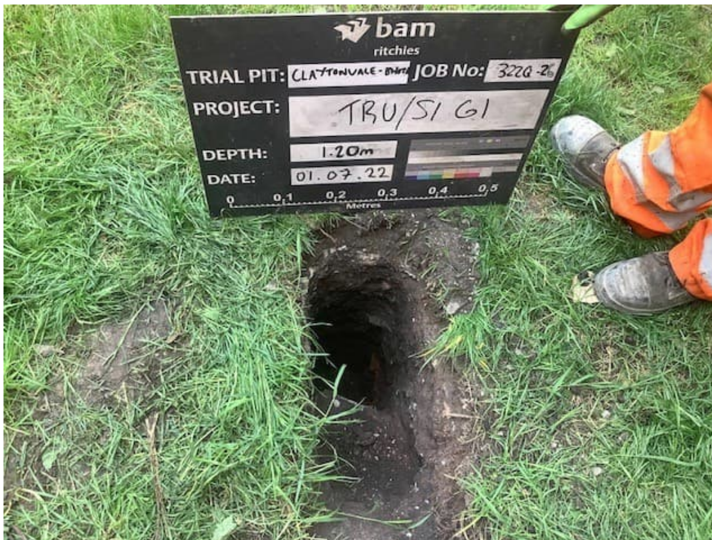
CLAYTON VALE-BH02A - 0.00 - 1.20m - West
