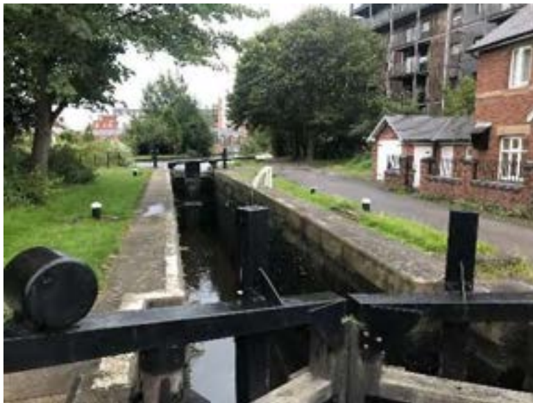
Figure 3.4 Lighting bollards east of Allan Turing Way
