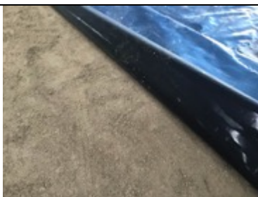
Acceptable sub base under the office area membrane
