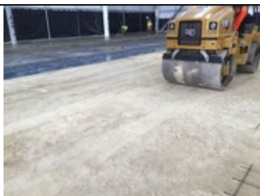
Substrate prep ahead of the membrane installation
