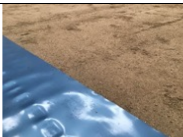
Rolled sand blinding substrate
