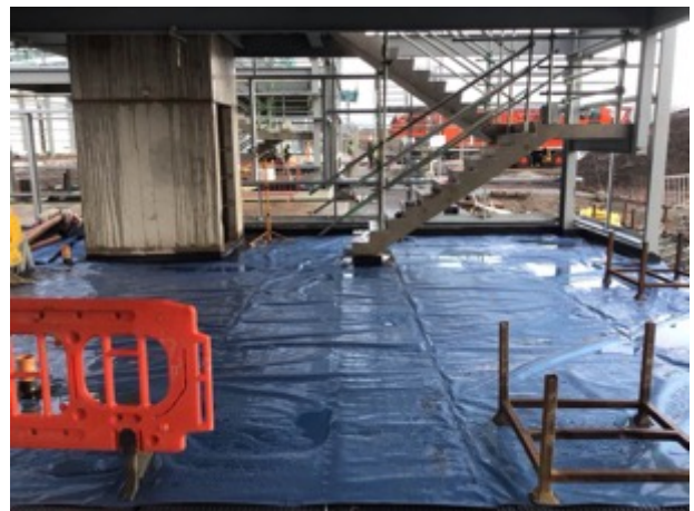
Unit 1 core area overview
