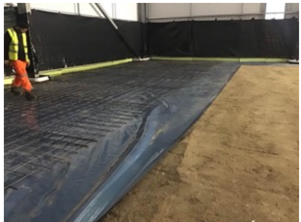
Membrane installed ahead of the first pour
