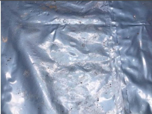
Membrane inspected after plant feet are raised
