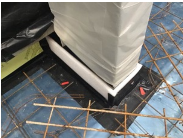
Restricted inspection to stanchion detailing
