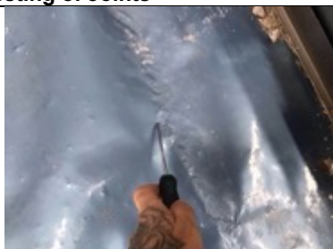
Probe test hand welded membrane lap joint
