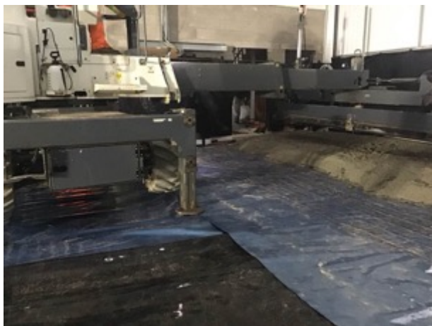
Laser screed machine keeping off the mesh on the membrane
