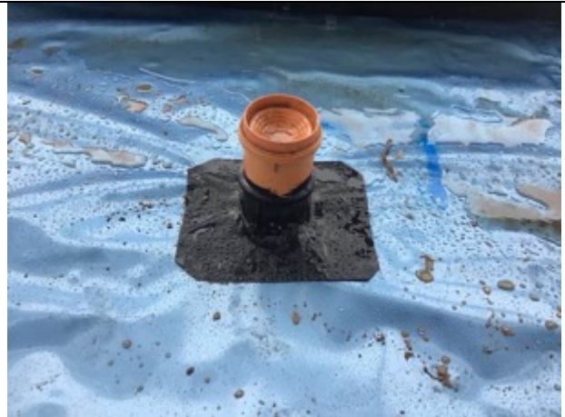
Stair core 3 pipe penetration
