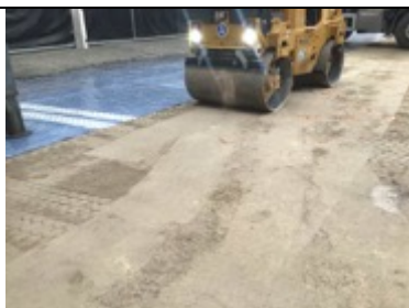
Substrate prep ahead of the membrane installation
