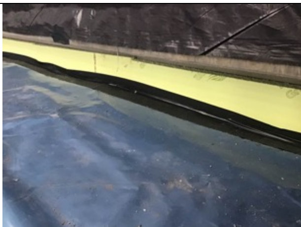
Restricted inspection to perimeter retro fit detailing
