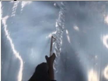
Testing hand welded membrane lap joint
