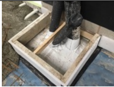
Pipe penetrations sealed using SAGM and heat applied
