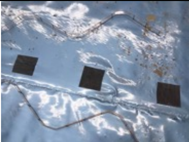
Recorded defects sealed using SAGM patch repairs and heat applied
