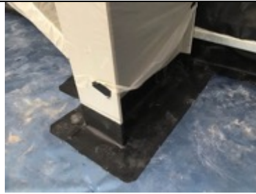
Stanchion detailing sealed using SAGM and heat applied
