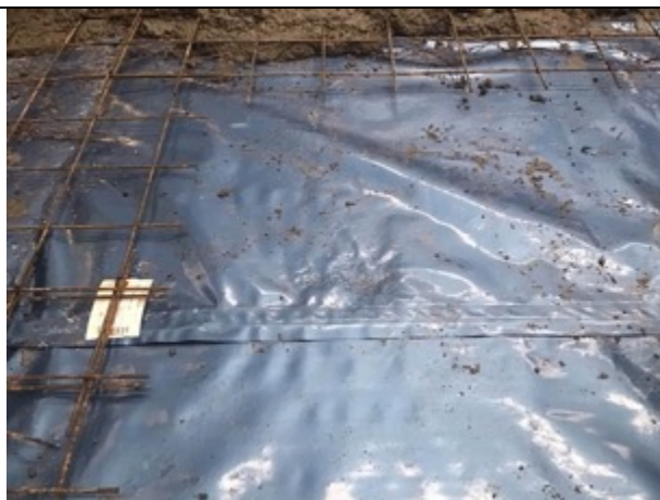
Membrane inspection after laser machine feet lifted
