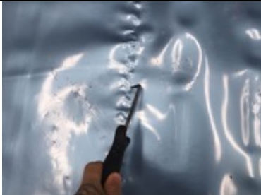
Probe test to hand weld membrane lap joint
