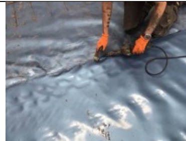
Hand welding membrane lap joint
