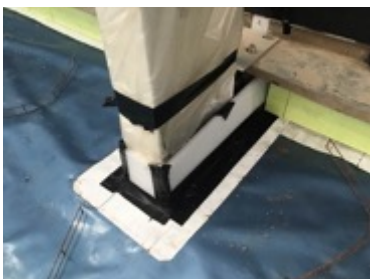
Insulation and miothene installed after the inspection of works carried out
