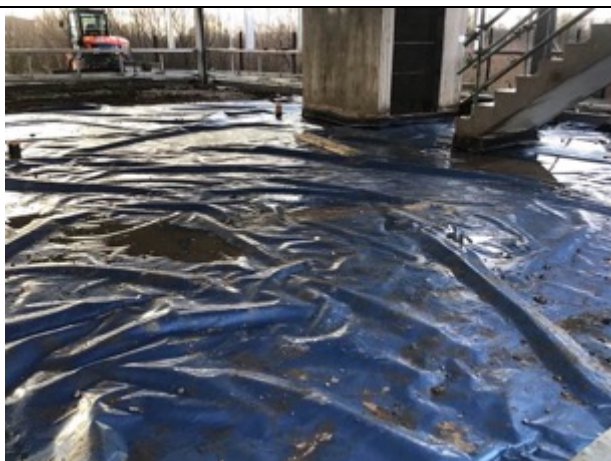
Unit 6 core area overview
