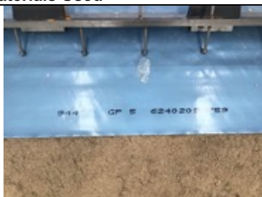
Evidence of Juta GP5 gas barrier membrane
