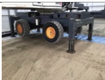
Plant keeping off the mesh above the membrane
