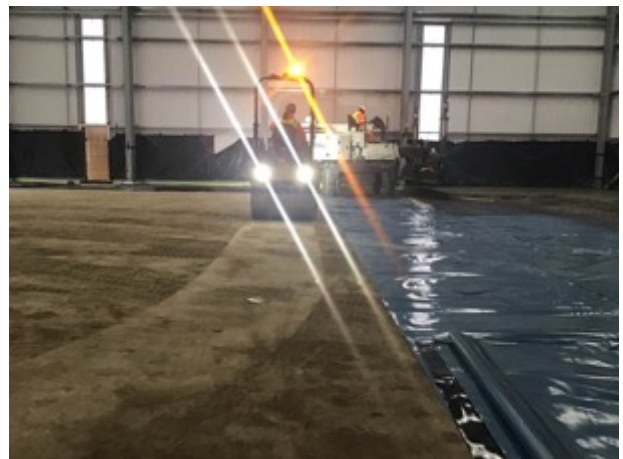
Sub grade rolled ahead of the membrane installation
