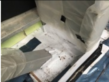
Sealed stanchion using SAGM and heat applied
