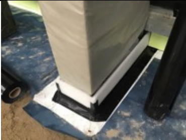
Miothene restricting stanchion inspection
