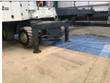
Plant keeping off the steel above the membrane
