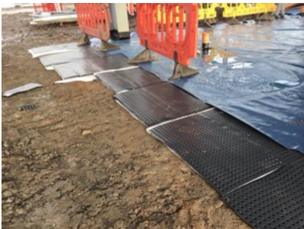
Vent mat installed under the membrane
