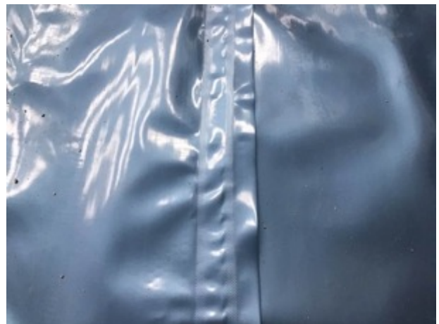
Sealed auto weld membrane joint
