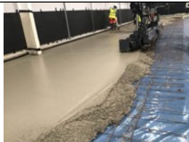
Laser screed installation over the membrane
