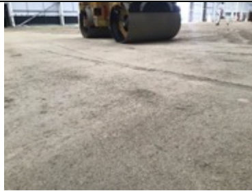
Close up of compacted sand blinding
