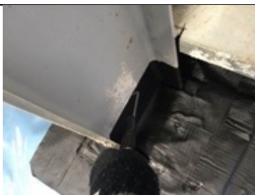
Testing sealed dock leveller area stanchion detailing using SAGM and heat applied
