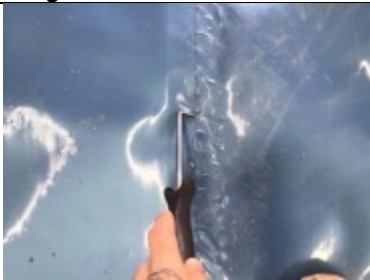
Testing hand welded membrane lap joint
