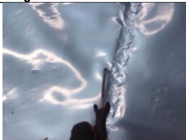
Testing hand welded membrane lap joint
