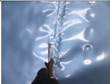
Probe test to hand welded membrane lap joint
