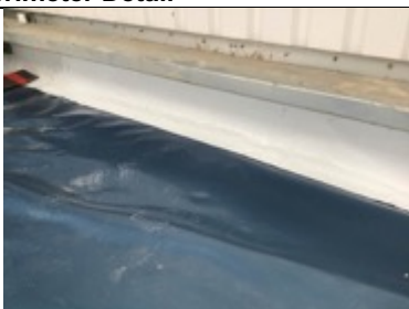
Perimeter retro fit detailing to cladding using SAGM and heat applied
