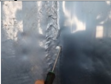
Probe test hand welded membrane lap joint
