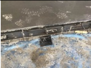
Sealed shuttering pin patch repair using SAGM and heat applied
