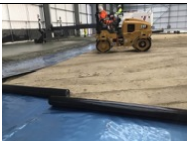
Roller prep ahead of the membrane installation
