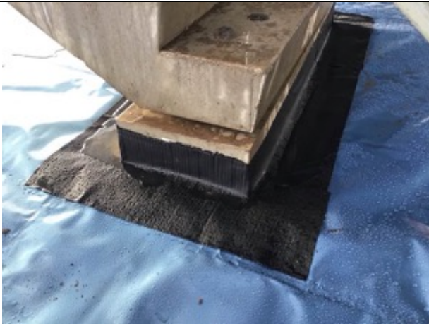
Stair base retro fit detailing
