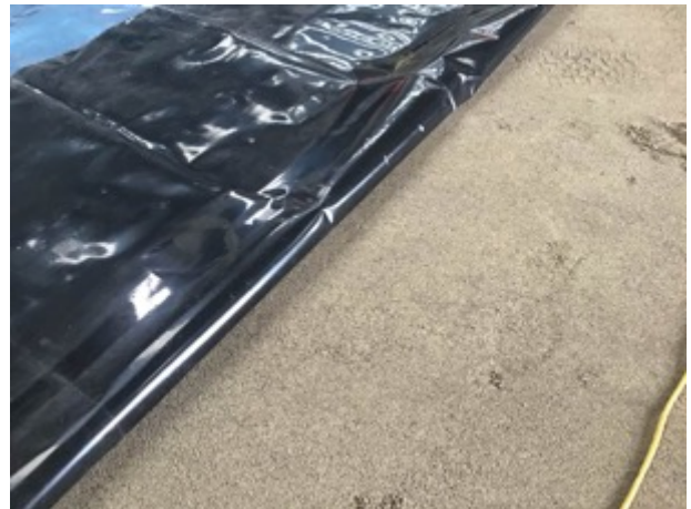
Rolled substrate under the membrane
