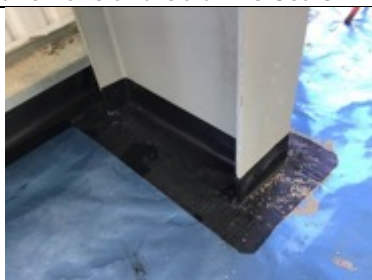
Sealed office area stanchion detailing using SAGM and heat applied
