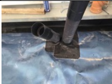
Sealed pipe penetrations using SAGM and heat applied
