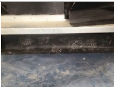
Retro fit detail to the perimeter cladding using SAGM and heat applied
