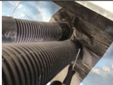
Testing pipe detailing
