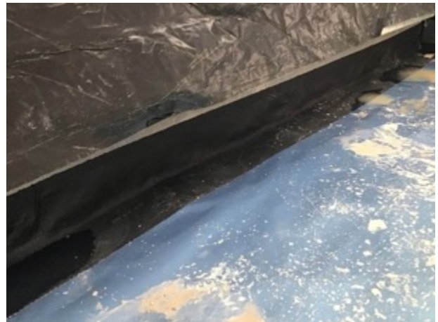
SAGM perimeter retro fit detailing
