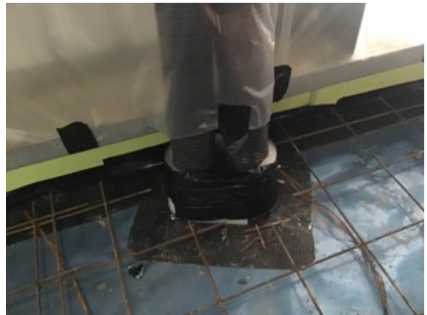
Restricted inspection to sealed pipe penetrations
