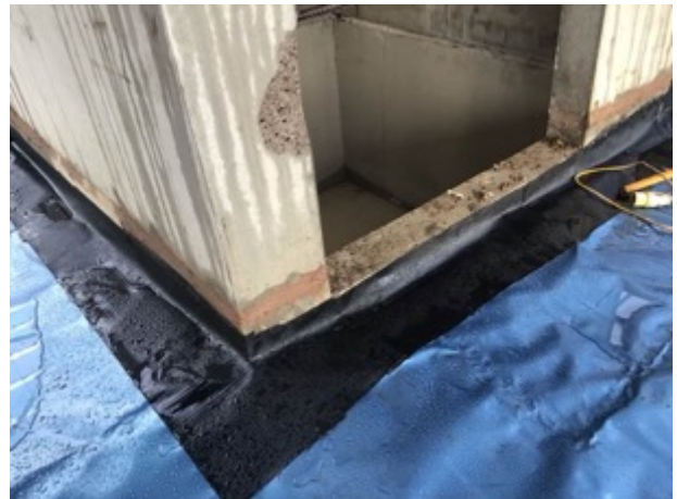
Lift pit retro fit detailing
