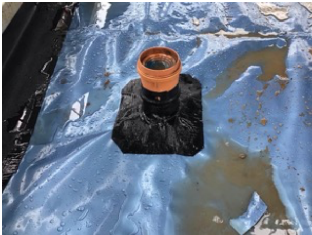
Stair core 2 pipe penetration
