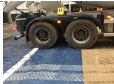
Wagons keeping off the steel above the membrane
