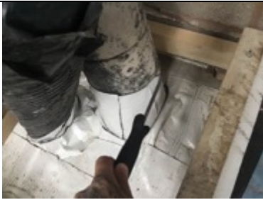
Probe test to pipe sealing
