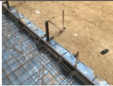
Membrane extended under the armoured joint
