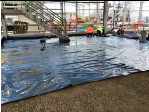
Stair core 2 overview
