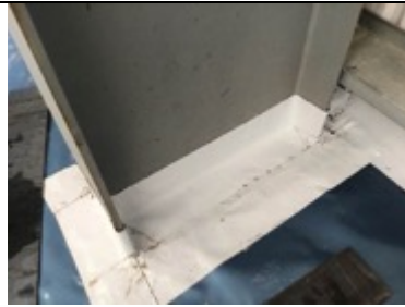
Sealed stanchion detailing using SAGM and heat applied
