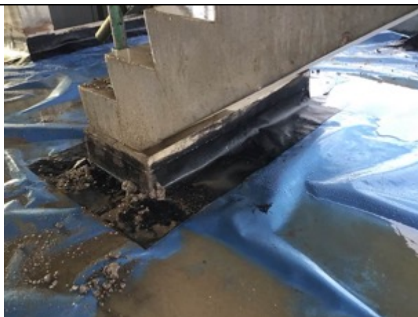
Sealed stair base
