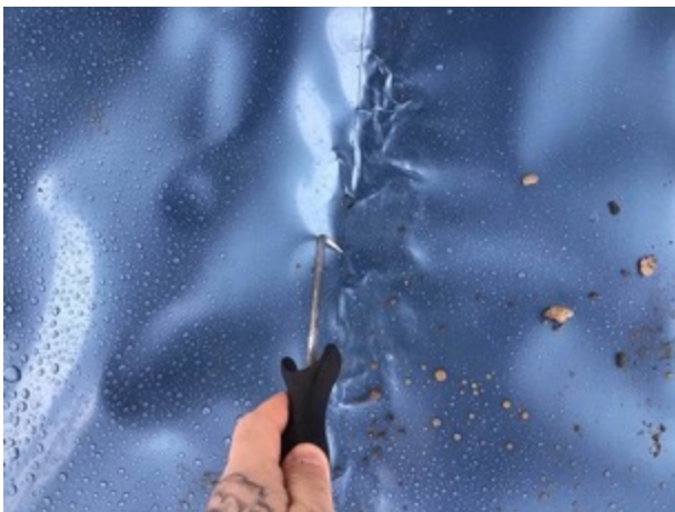
Probe testing hand welds
