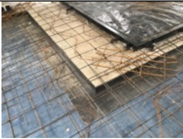
Corner retro fit detailing using SAGM and heat applied
