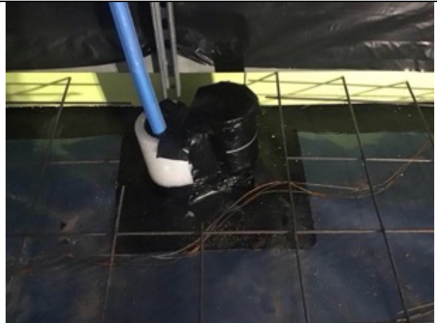
Sealed pipe penetrations with miothene installed by site
