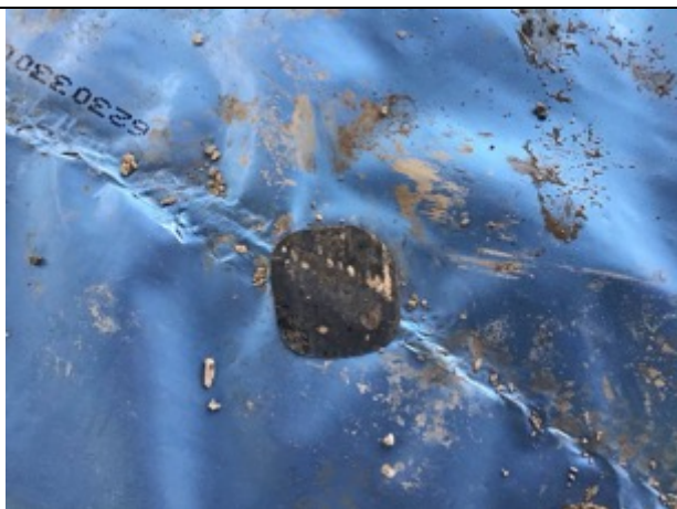
SAGM patch repair
