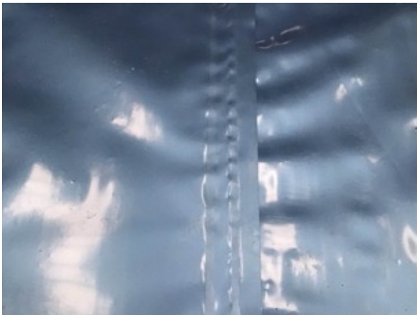
Sealed auto weld membrane joint
