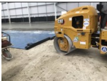
Roller prep ahead of the membrane installation
