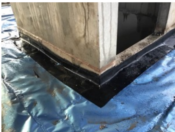
Lift pit retro fit detailing
