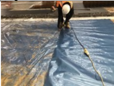
Membrane hand welded into position
