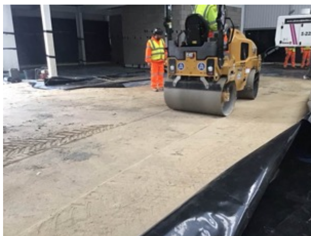
Rolled substrate ahead of the membrane installation
