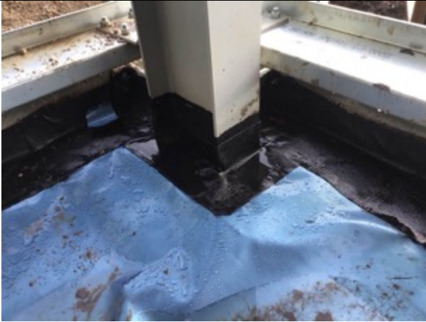
Sealed stanchion detailing
