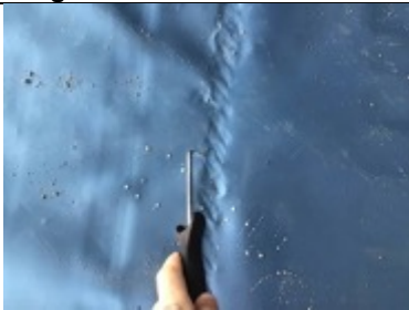
Hand weld membrane lap joint testing
