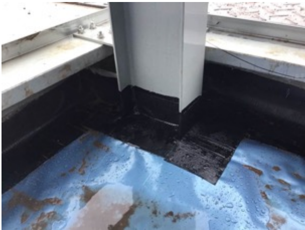
Stair core3 stanchion detailing
