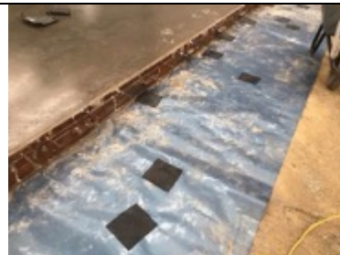
Armoured joint pin hole patch repairs made using SAGM and heat applied
