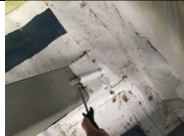
Probe test to stanchion sealing
