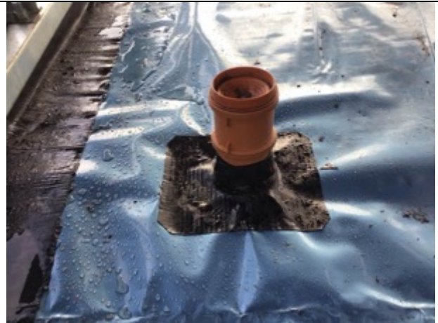
Sealed pipe penetration
