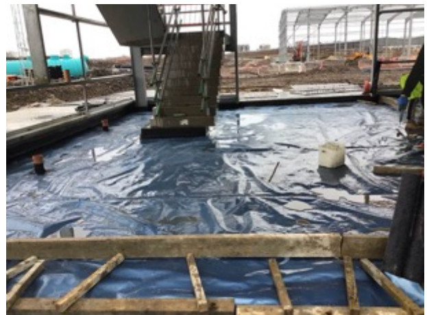
Stair core 3 overview
