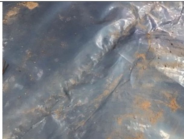
Membrane inspected after laser screed machine feet raised
