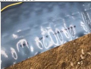
Evidence of Juta GP5 gas barrier membrane
