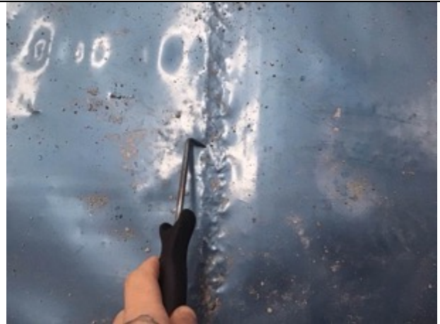
Probe test to hand weld joint
