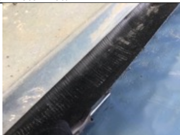
Testing perimeter detailing
