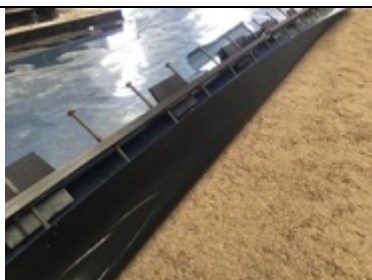
Acceptable sub base under the dock leveller membrane
