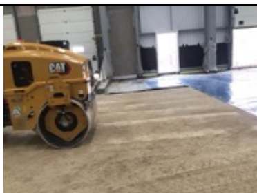
Roller prep ahead of the membrane installation
