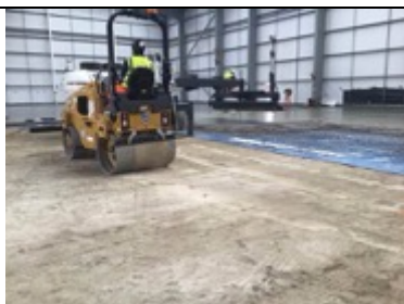
Roller prep ahead of the membrane installation
