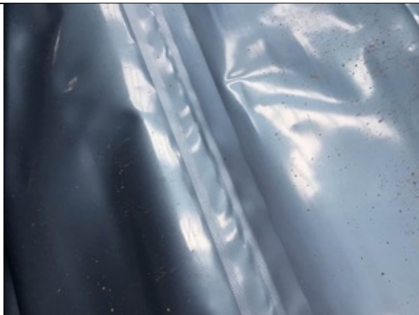
Sealed auto weld membrane joint
