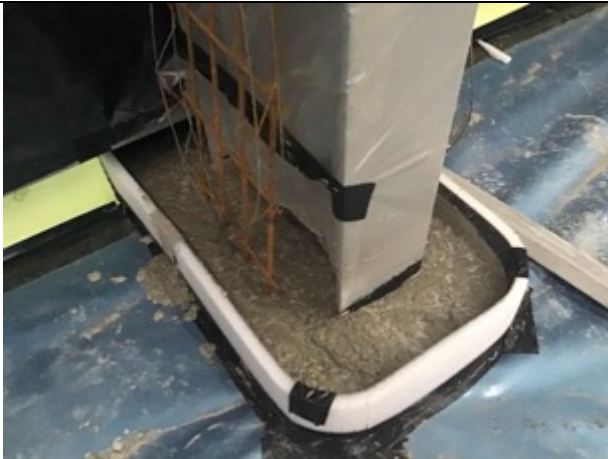
Sealed stanchions poured prior to the inspection
