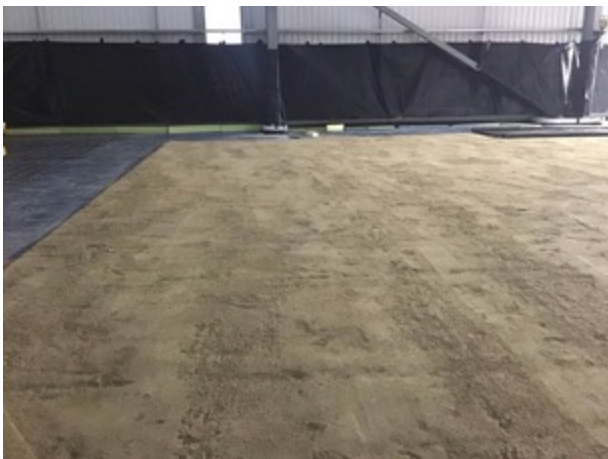
Blinded substrate prior to membrane installation
