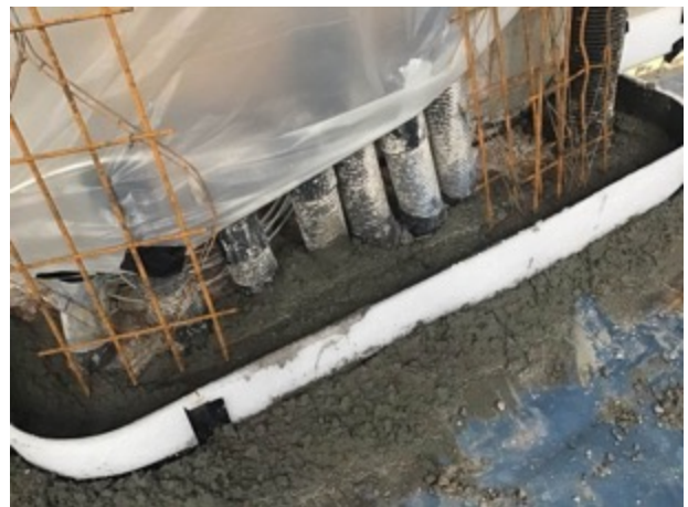
Restricted inspection to pipe penetrations
