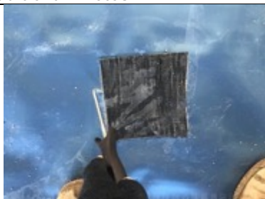
Testing sealed patch repair made by the installers prior to our inspection using SAGM and heat applied
