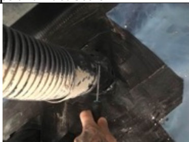
Pipe penetrations testing
