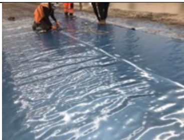
Membrane hand welded into position ahead of the pour
