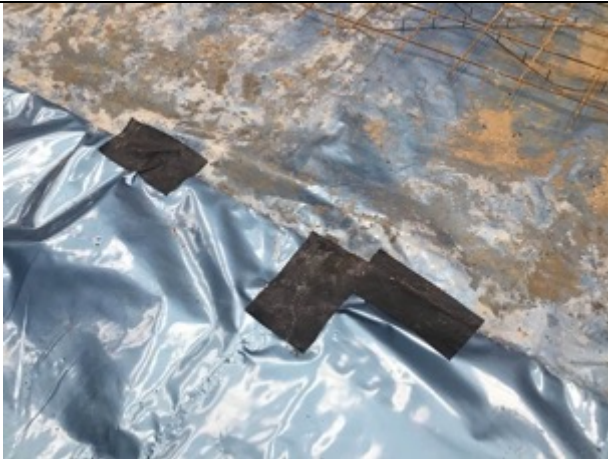
Sealed SAGM defect patch repairs
