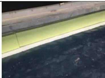
Restricted inspection to perimeter detailing
