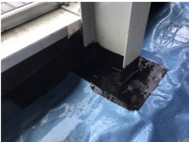
Stair core 2 stanchion detailing
