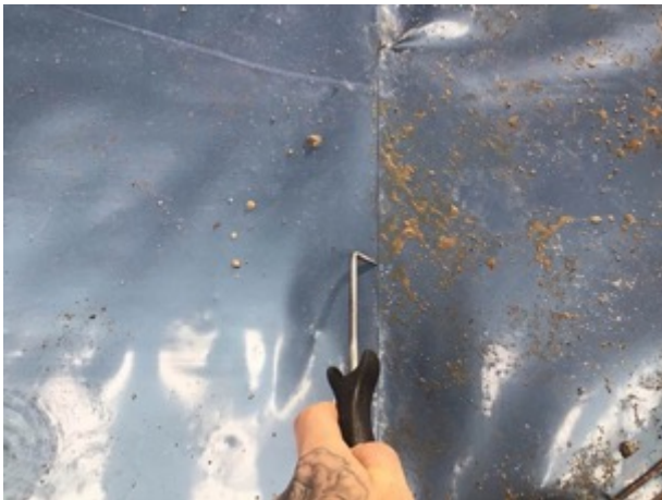
Probe test to sealed hand weld membrane joint
