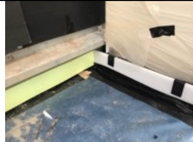
Insulation and miothere installed after the inspection
