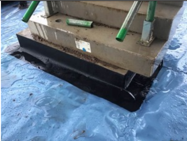
Stair core 3 detailing
