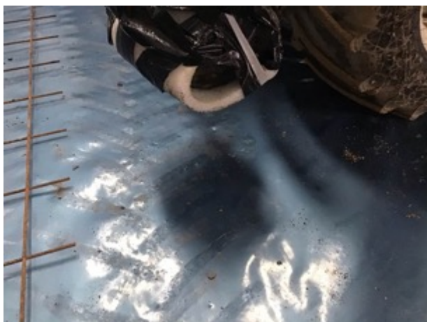
Membrane inspected after laser machine feet were raised
