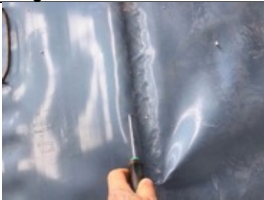
Probe test hand welded membrane lap joint
