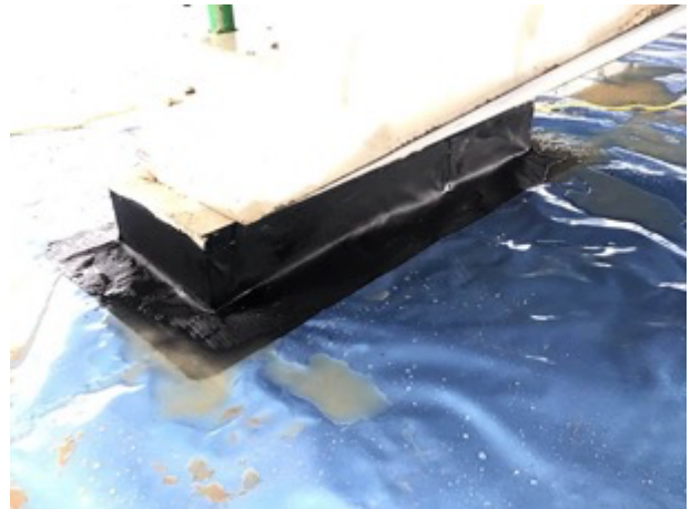
Stair core 2 detailing
