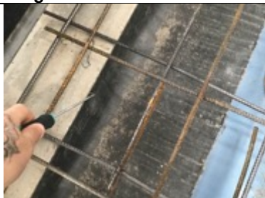
Probe testing the membrane retro fit detail to the dock levellers
