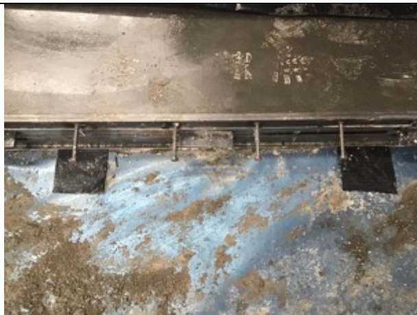
Sealed SAGM pin hole repairs
