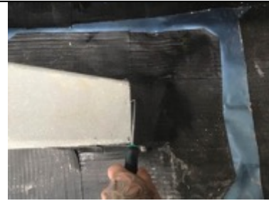
Stanchion detail testing
