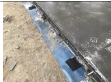
Pin patch repairs made using SAGM and heat applied
