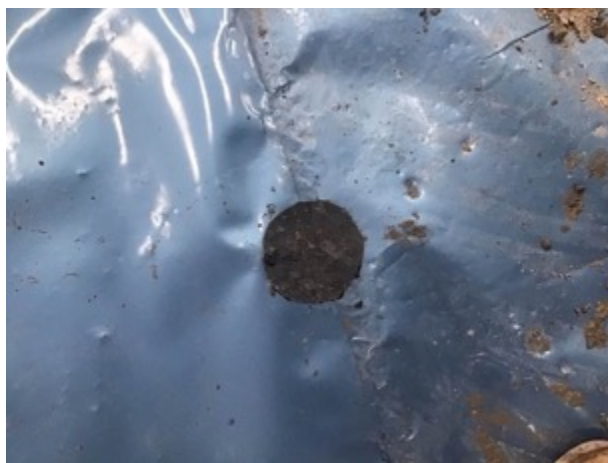
Sealed SAGM patch repair during the installation
