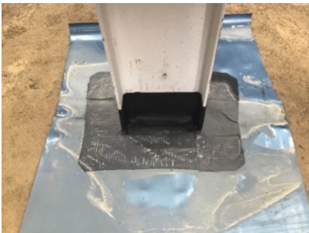
Sealed stanchion detailing using SAGM
