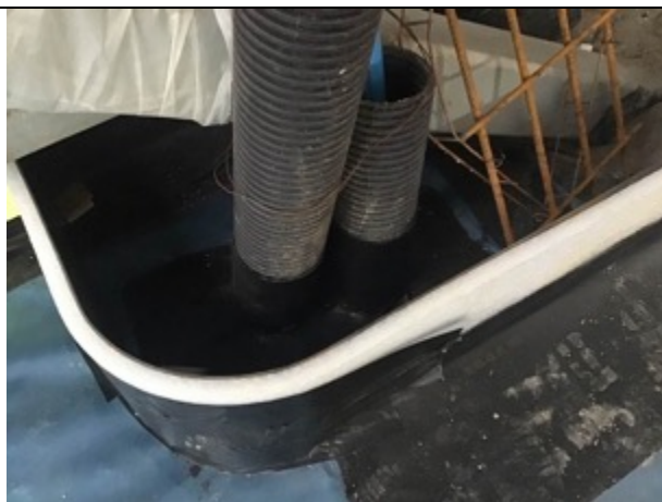
Sealed pipe penetrations using SAGM
