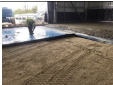
Membrane installed 4 meters at a time ahead of the pour
