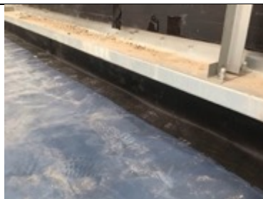
Retro fit detail to the perimeter cladding using SAGM and heat applied
