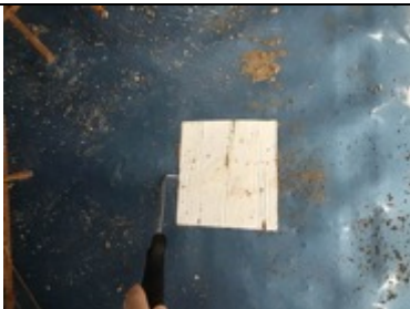
Sealed patch repair using SAGM and heat applied
