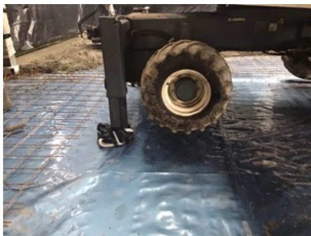
Plant keeping off the membrane and using miothene to protect the membrane from the laser machine feet
