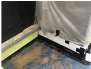
Insulation and miothene installed after the inspection
