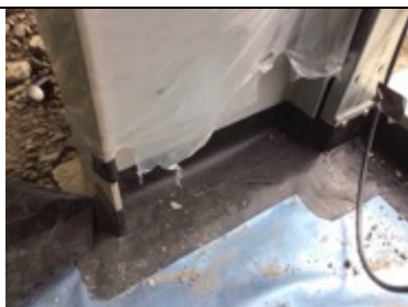
Stanchion detailing sealed using SAGM and heat applied
