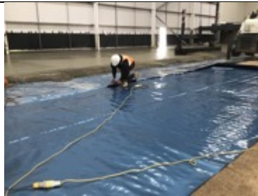
Membrane hand welded into position ahead of the pour
