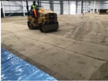
Substrate prep work ahead of the membrane installation
