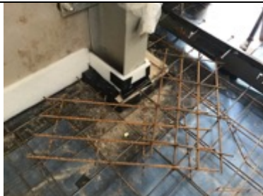
Miothene installed at the perimeter and around the stanchion detail
