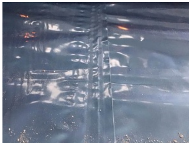
Sealed auto weld membrane joint
