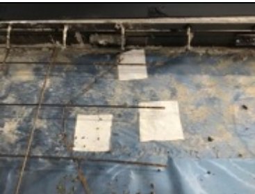
Sealed pin hole repair patches using SAGM and heat applied
