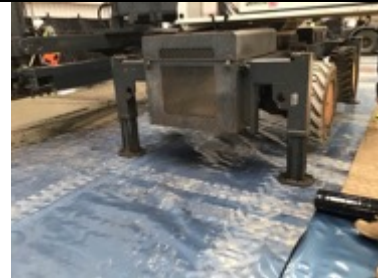
Plant keeping off the mesh above the membrane
