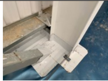
Sealed stanchion detailing using SAGM and heat applied
