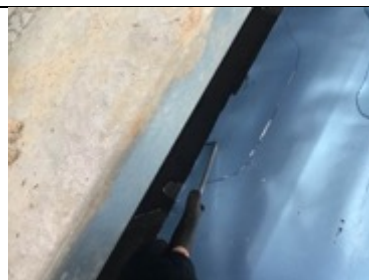
Perimeter detailing testing
