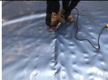
Membrane being hand welded together
