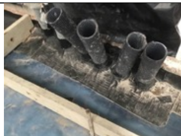
Pipe penetrations sealed using SAGM and heat applied
