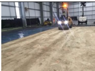
Substrate prep ahead of the membrane installation
