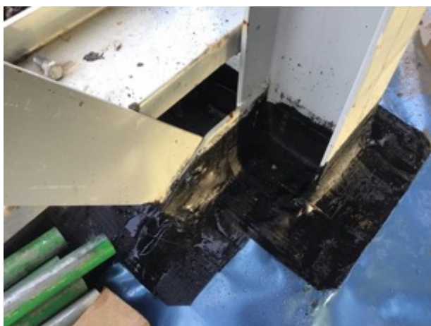
Sealed stanchion detailing
