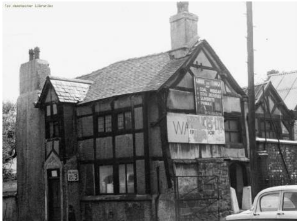
1968: BUILDING IS IN USE FOR LIGHT INDUSTRIAL PURPOSES. NOTE THE ROOF COVERINGS ON THE CROSSWING HAVE BEEN CHANGED FROM THOSE IN THE 1960 PHOTO. NOTE ALSO THE ROOF COVERINGS ON THE EXTANT PORTION APPEAR TO BE MISSING, AND THE ROOF OF THE NOW-DEMOLISHED PORTION IS COVERED WITH CORRUGATED SHEETS.
