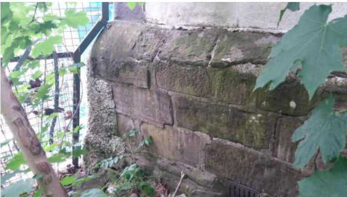
19: NORTH ELEVATION, CROSSWING. STONE PLINTH COURSE AT GROUND LEVEL WITH LATER CEMENT-BASED POINTING AND RENDER.
