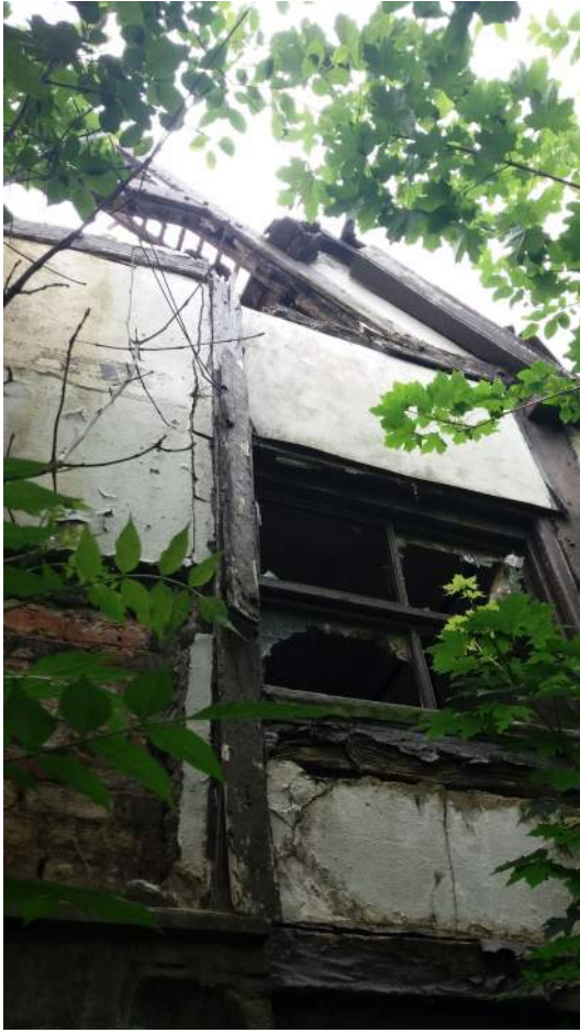
21: NORTH ELEVATION. GABLE OF CROSSWING. ROOF STRUCTURE BEYOND IS NO LONGER PRESENT.
