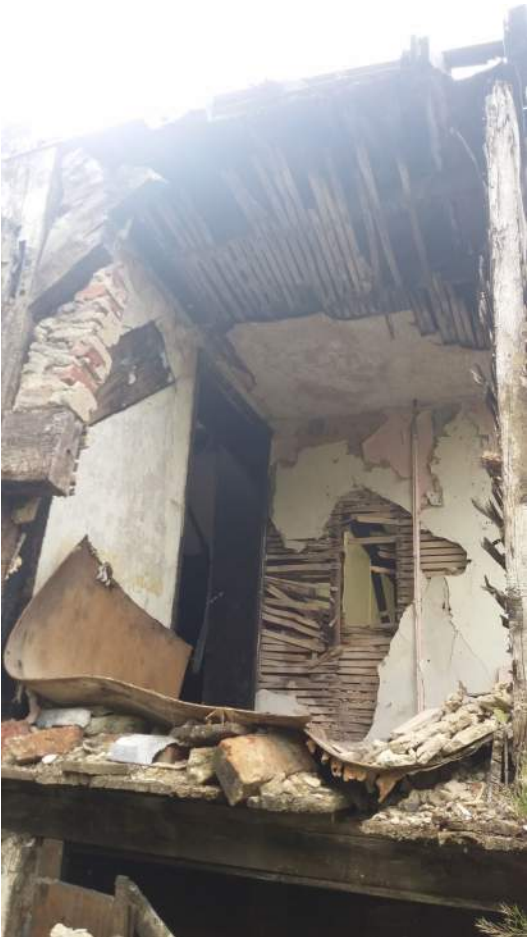
35: LOOKING INTO ROOM F5.
