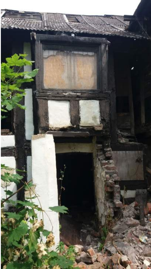
08: SOUTH ELEVATION. ENTRANCE INTO BUILDING AND BAY WINDOW ABOVE. EVIDENCE OF A PORCH, NOW REMOVED.
