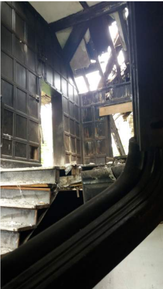
33: ROOM F4. MAIN STAIRWAY WITHIN THE BUILDING.
