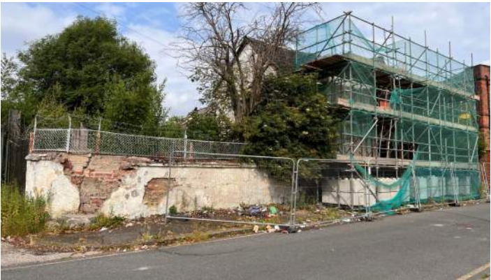
02: EAST ELEVATION WITH SCAFFOLD PROPPING IN PLACE. MOUNTING BLOCK IS AT THE LEFT OF FRAME.
