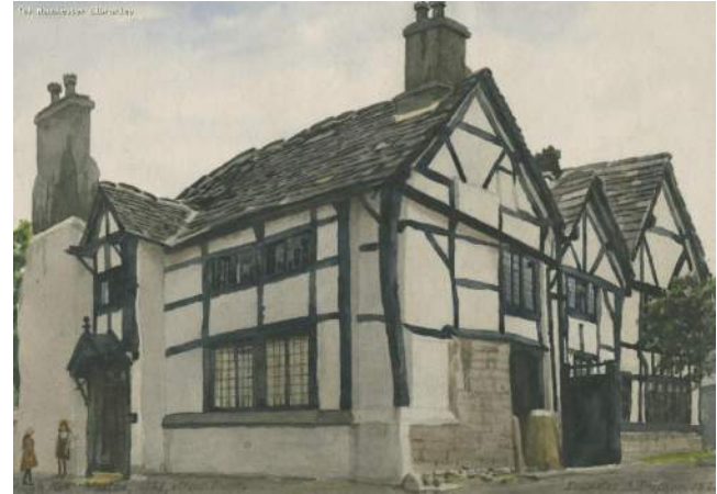
1925: NOTE THE ENTRANCE WHICH HAS BEEN INTRODUCED IN THE NORTH WALL OF THE CROSSWING, ADJACENT TO THE STONE WALL OF THE CHIMNEY.
