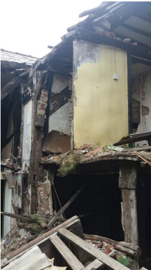
15: NORTH ELEVATION. CENTRAL BAY OF MAIN RANGE. FIRST FLOOR AND ROOF ARE IN SITU. NOTE TIMBER COLUMNS AND PRIMARY BEAM SUPPORTING FIRST FLOOR.
