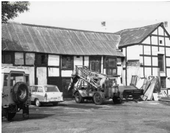
1970a: MAIN RANGE AND SOUTH END OF CROSSWING.
