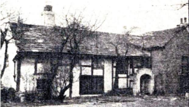
1849: MAIN RANGE, SOUTH ELEVATION. NOTE THE SLATE / STONE SLATE ROOF COVERINGS TO THE MAIN RANGE, THE PORCH SURROUNDING THE ENTRANCE AND THE BRICK WALLS OF THE CROSSWING.
