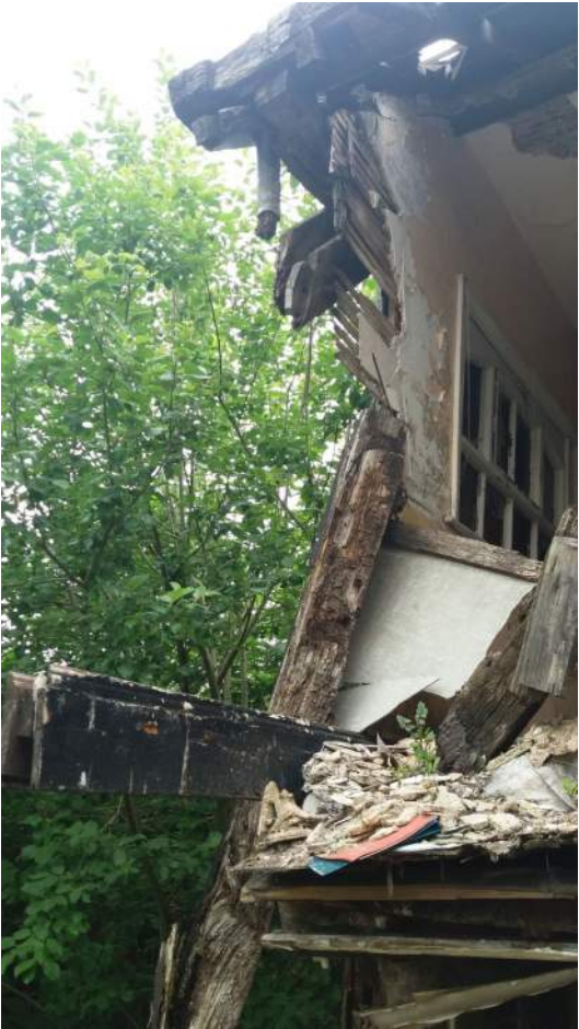
17: NORTH ELEVATION. CORNER OF PROJECTION FROM MAIN RANGE. CORNER POST HAS BEEN REMOVED.
