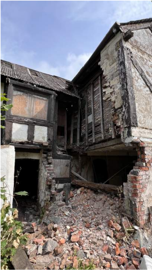
06: SOUTH ELEVATION. REAR WALL OF CROSSWING AT JUNCTION WITH MAIN RANGE. NOTE STUD WALL WITH LATH AND PLASTER AT LEVEL 01.
