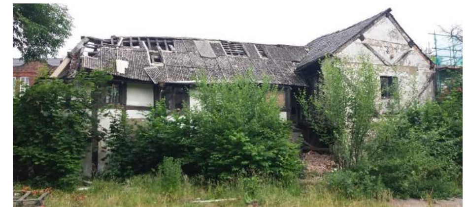
Figure 2.2 – South elevation, general view
