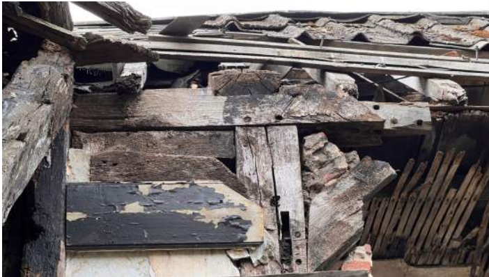
18: NORTH ELEVATION. CENTRAL BAY OF MAIN RANGE. EXAMPLE OF PEG JOINTS BETWEEN TIMBER MEMBERS.
