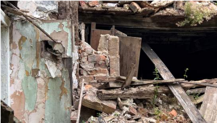
14: NORTH ELEVATION. CENTRAL BAY OF MAIN RANGE. REMNANT WALL AND STONEWORK ADJACENT TO DEMOLISHED PORTION OF BUILDING. FIRST FLOOR IS IN SITU.
