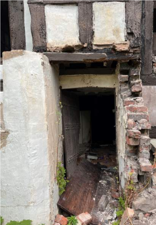
09: SOUTH ELEVATION. REMNANT WALLS OF A PORCH, NOW REMOVED. TIMBER DOOR IS IN SITU.
