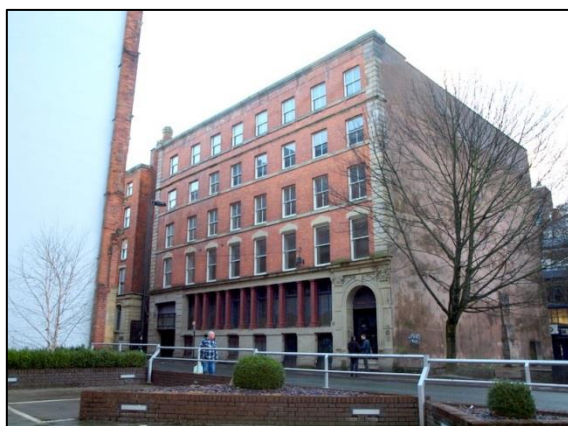
Figure 2: 11 Bloom Street (prior to works starting and installation of scaffolding).
