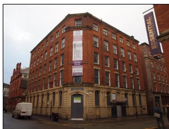
Figure 3: Mindel House (prior to works starting and installation of scaffolding).
