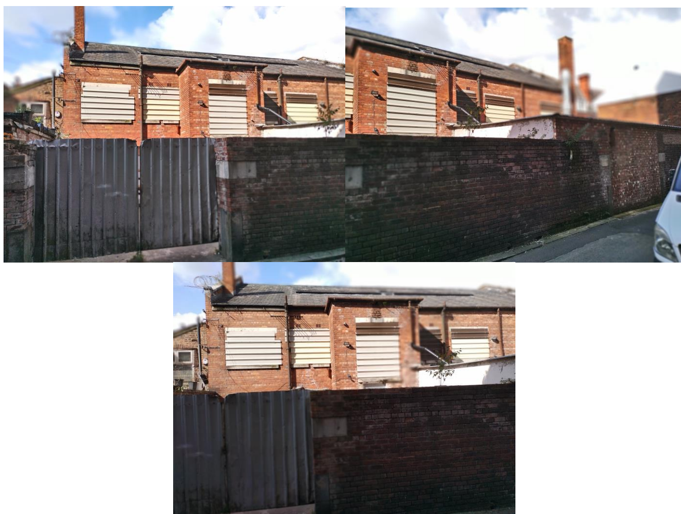
Fig. 2 – Views of the application site from Bankley Street
