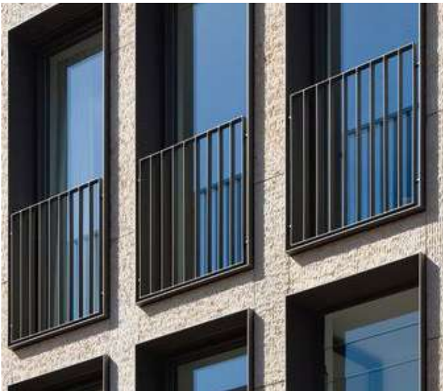
Example of the metal railing within a metal surround
