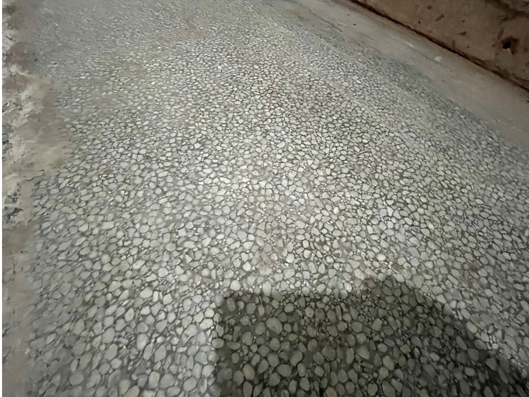
Figure 30 – Example of granolithic marble terrazzo flooring to the curved bay area.
