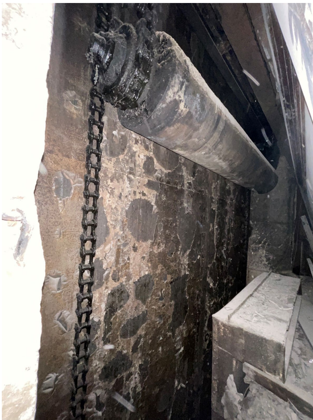
Figure 17 – An example of one of the original 1860s roller shutter mechanism found within the under window cavities, which presumably could be wound allowing the wright iron shutters to be lifted into place via concealed, hinged timber leaf's.
