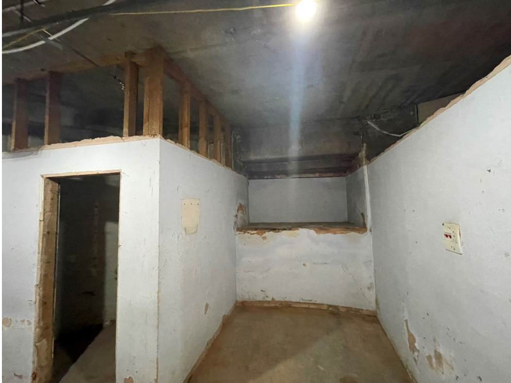
Figure 28 – The room beneath the semi-circular bay, showing modern studwork divisions and c1960s/70s reinforced concrete ceiling structure.
