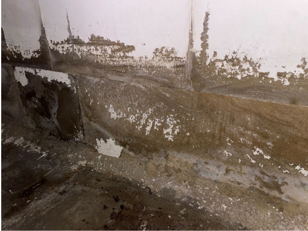
Figure 25 – Detailed view of the interior of the stone vault, showing the ashlar stone through modern paint layers.
