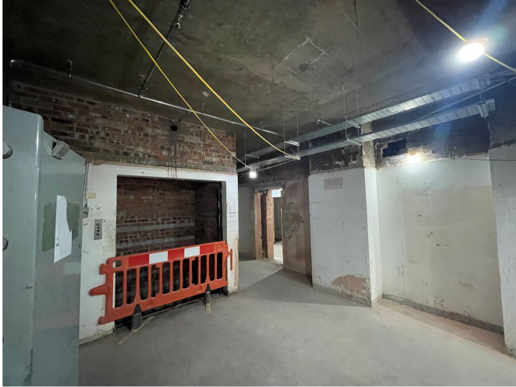
Figure 23 – The centre of the basement, showing the modern, 20 th century hoist to the left, and doorway leading into room beneath semi-circular rear bay. Note this area underwent substantial alterations during the 1960s/70s with the insertion of reinforced concrete ceiling structure.
