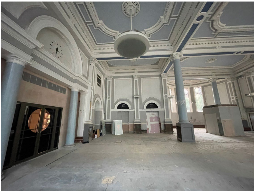
Figure 14 – Looking north-west across the western end of the banking hall, showing the original entrance (left), which gives access from Mosley Street. The blocked doorway to the left leads into one of two original stone staircases, whilst the blocked doorway to the right would have presumably originally led into the bank manager's office.
