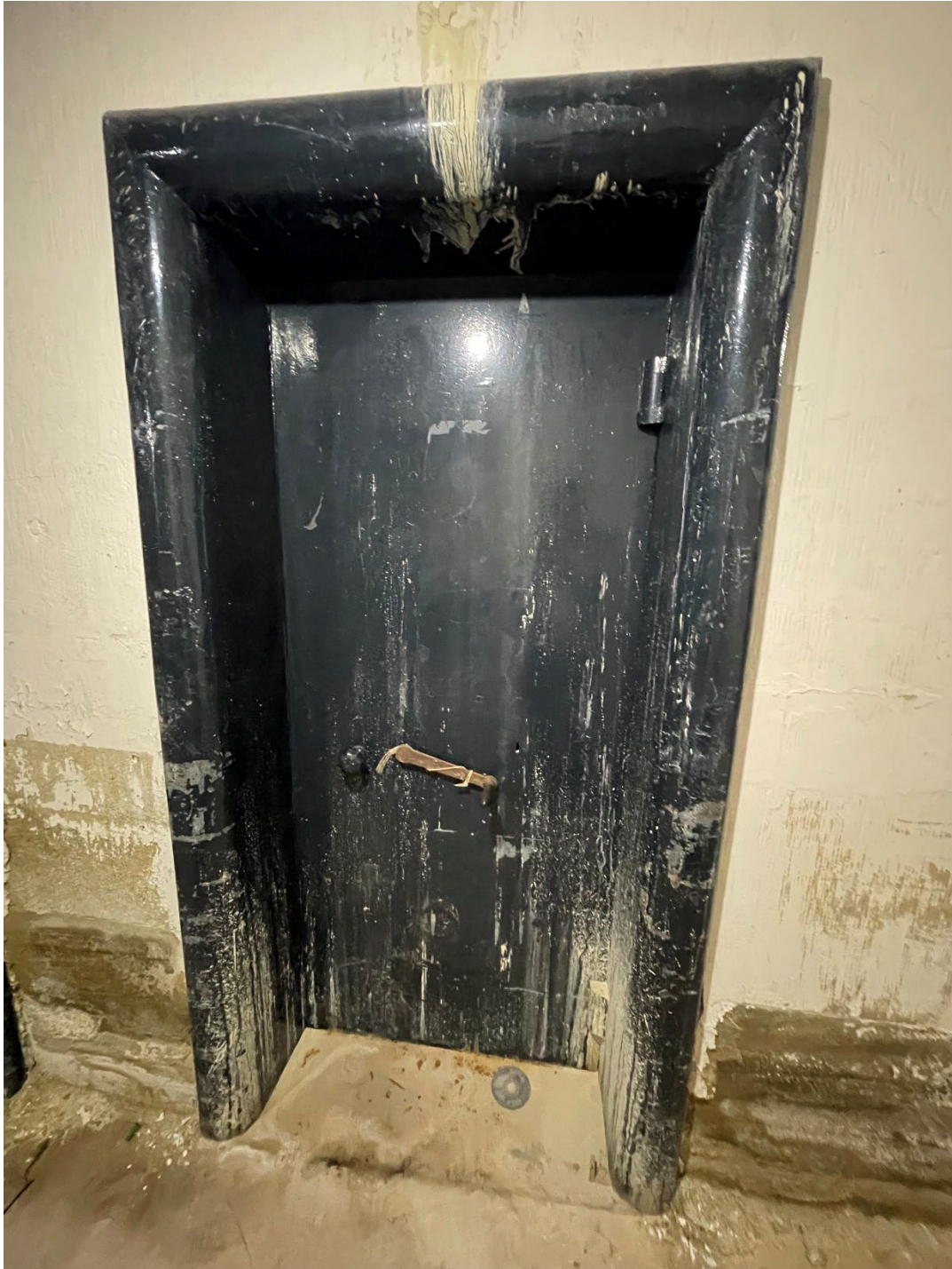
Figure 24 – One of two original iron safe doors leading into a single stone vault. Notice the original ashlar stone walls appearing through modern layers of paint.
