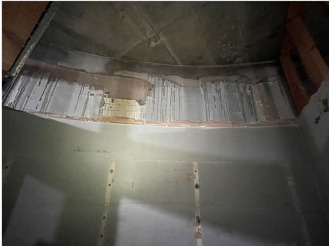
Figure 29 – Detailed view of the surviving white ceramic tiling to the curved walls, seen here partially exposed.
