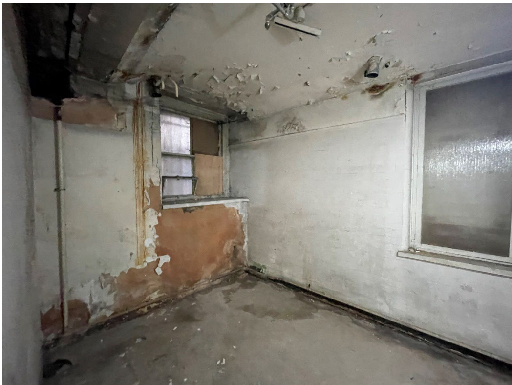
Figure 26 – A room to the north-east corner, which contains white ceramic tiling and a surviving original sash window (left).
