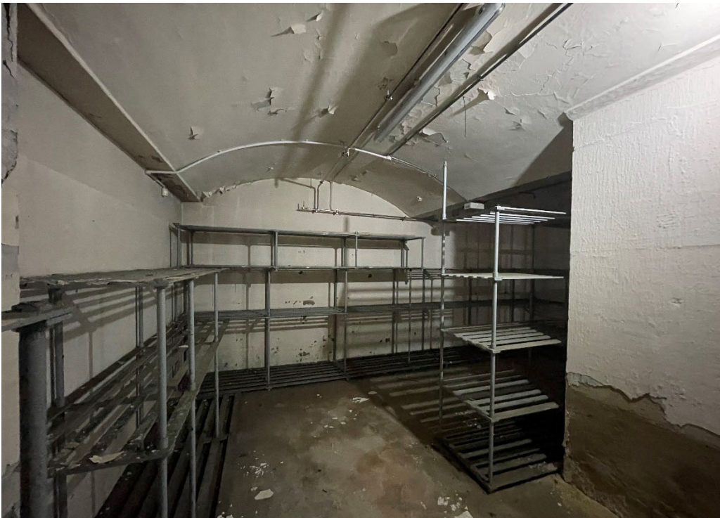
Figure 22 – A vault to the eastern corner showing original ashlar stone support for columns to banking hall (right) and later metal racking.
