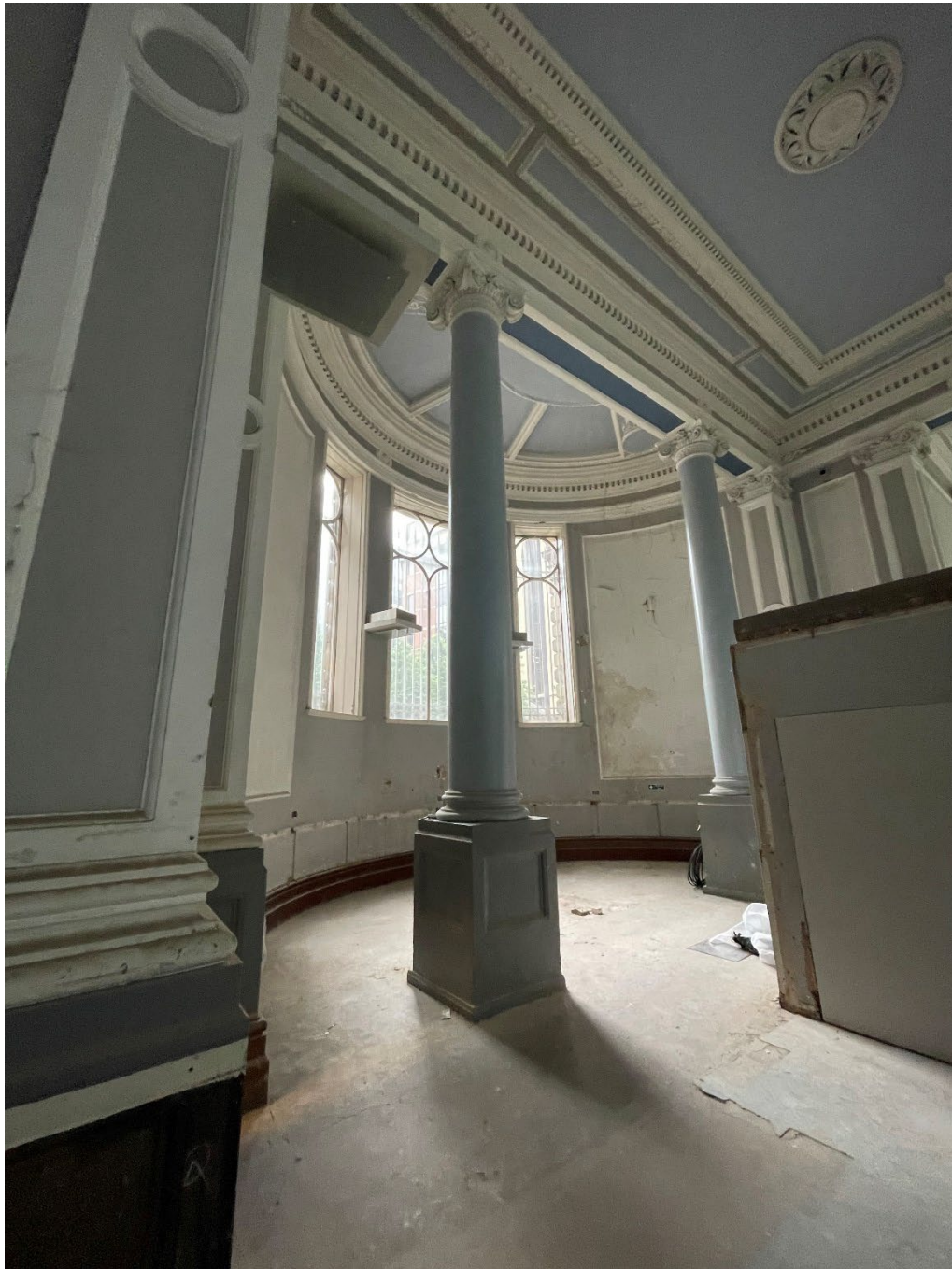
Figure 19 – Looking into the rear semi-circular bay along the rear elevation. The decorative framework to the ceiling was designed as a glazed laylight, lit from skylights on the roof above. These were either over-painted or filled with solid panels at some time in the c1960s/70s.
