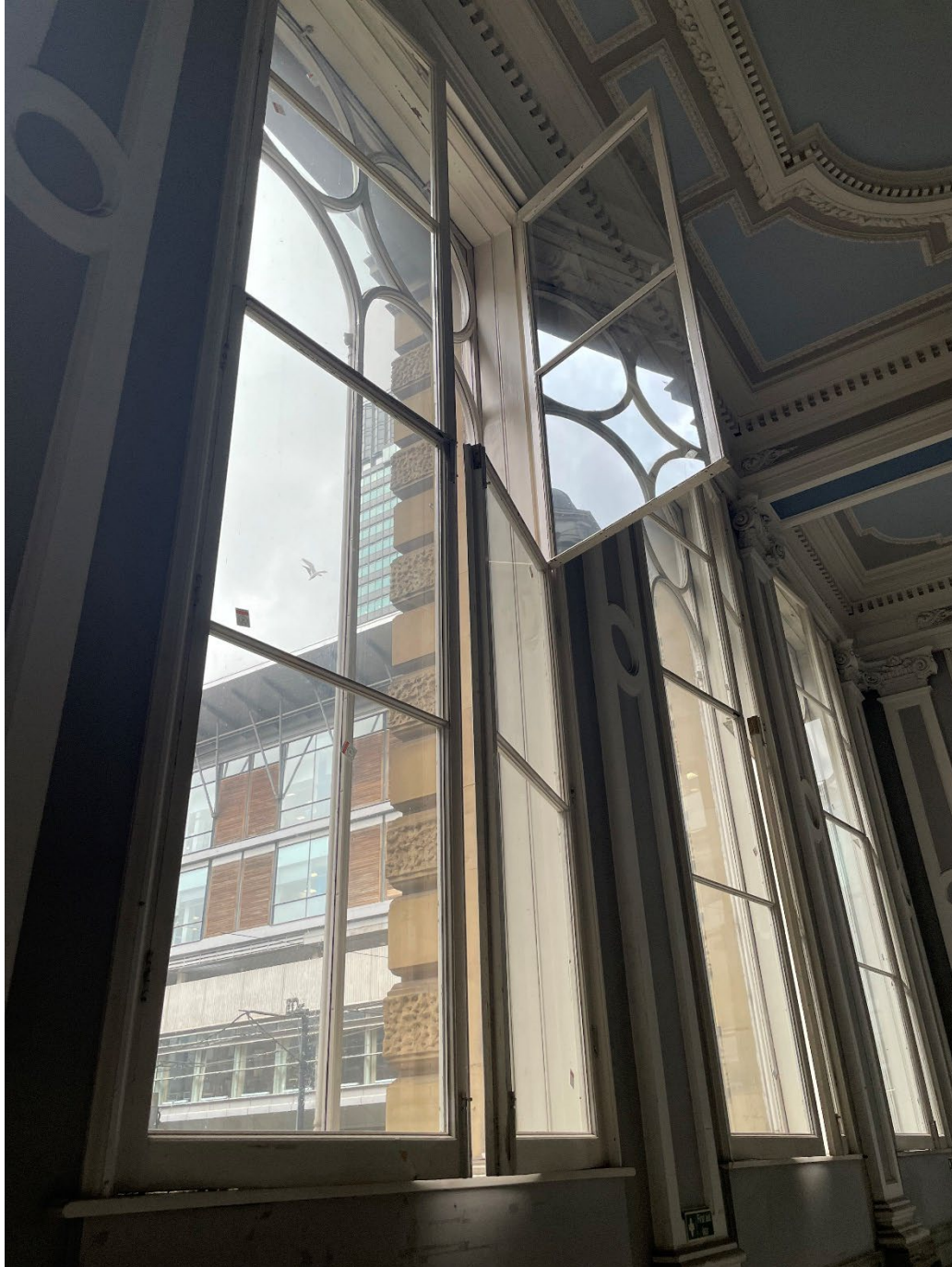
Figure 18 – The windows to the York Street elevation, showing the later secondary glazing.
