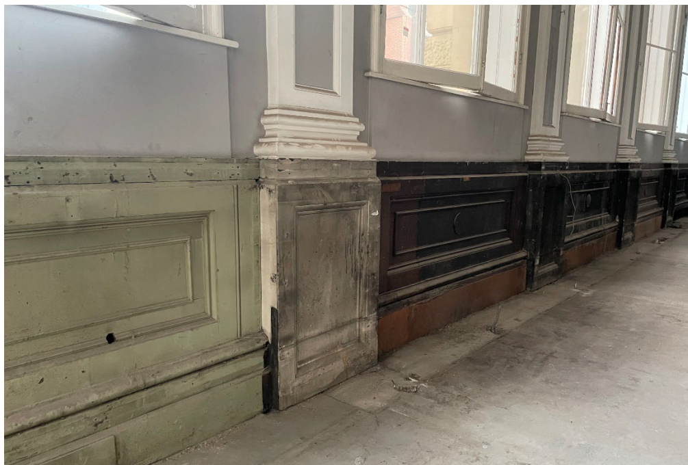
Figure 16 – Detailed view of the original hardwood timber panelling beneath the windows, that runs around the majority of the room. The right of the image shows the original varnished/stained finish of the timber as apposed to the 20 th century paint scheme covering the left panel.
