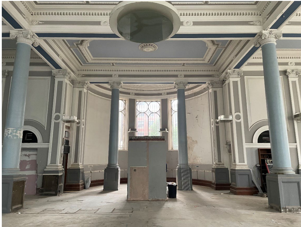
Figure 15 – Looking north-west along the centre of the banking hall towards the curved bay at the rear of the building, showing the mid-to-late 20 th century hoist (which has LBC consent for removal) partially blocking the view to the centre.
