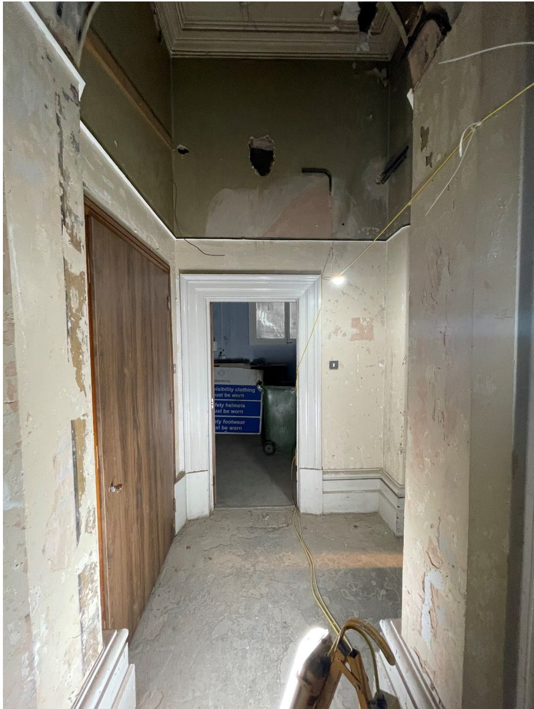
Figure 21b – A view looking from the head of the basement stairs (extreme right) towards the northernmost room, showing the deeply moulded timber architrave, skirting and stone floor.
