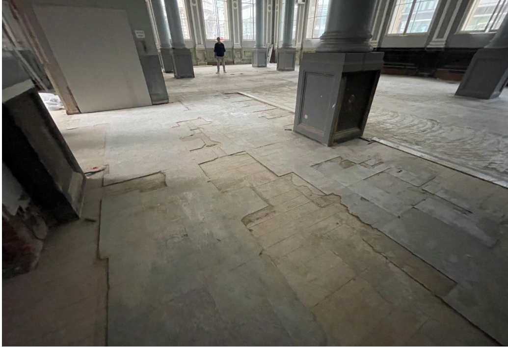
Figure 21 – An example of the differing areas of reflooring, which includes large areas of reinforced poured concrete rafts introduced during the 1960s/70s redevelopments.
