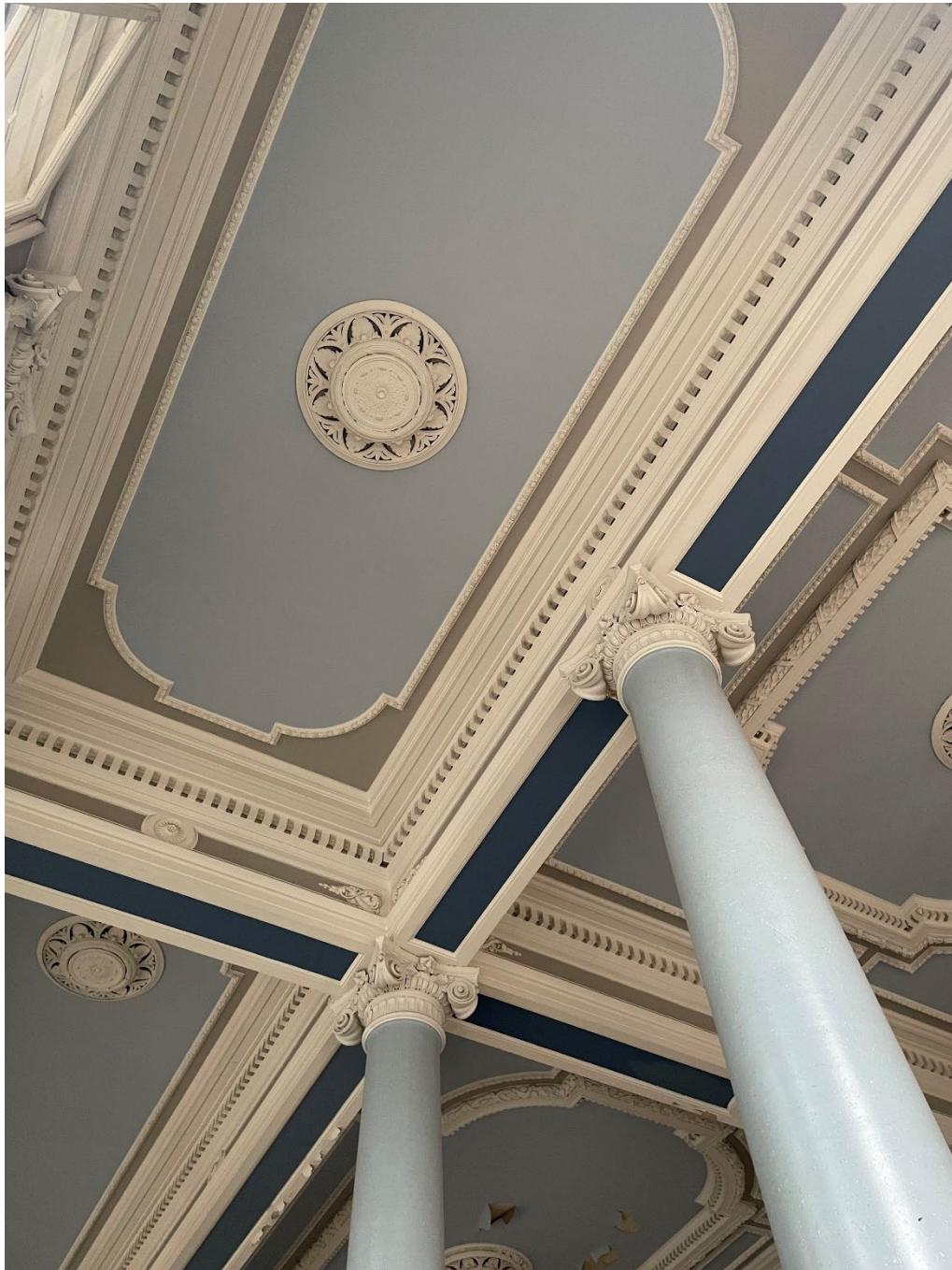
Figure 20 – Looking up at the original decorative plasterwork, plaster ceiling roses, and hollow cast iron ionic columns.
