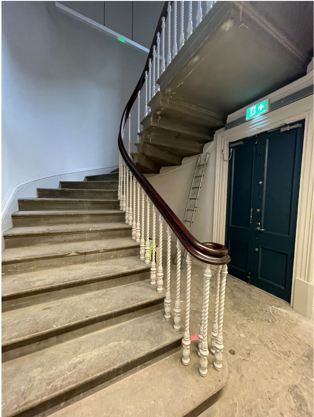
Figure 21a – The original cantilevered stone staircase to the northern corner, giving access from ground level to the upper floors. Note the decorative barley twist cast iron spindles. The steps and hallway flooring are of solid stone.
