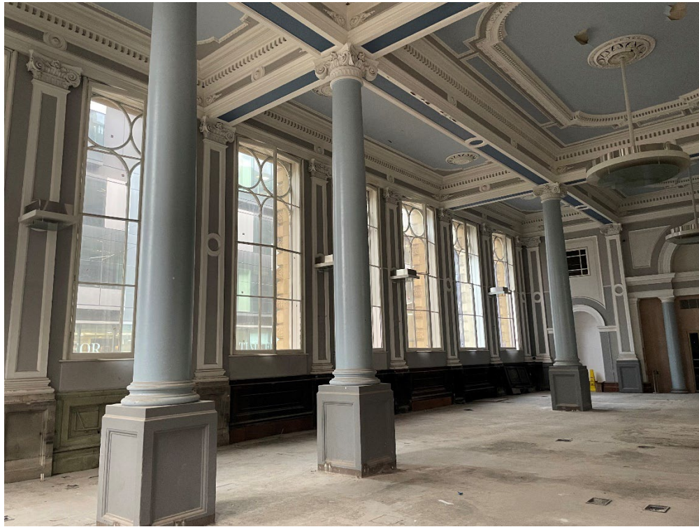
Figure 13 – Looking along the Mosley Street elevation, showing the large original cast-iron windows.
