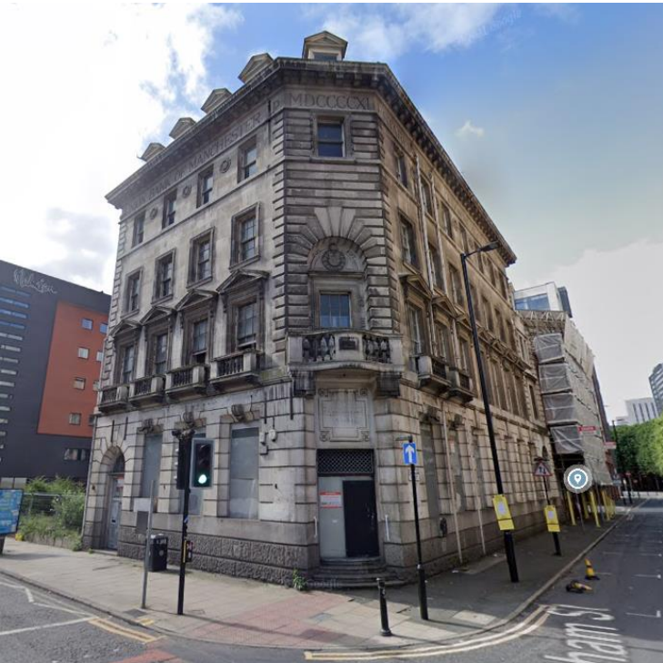
Figure 2-2 Existing Grade II Listed Building, Former Union Bank (Google street view)
