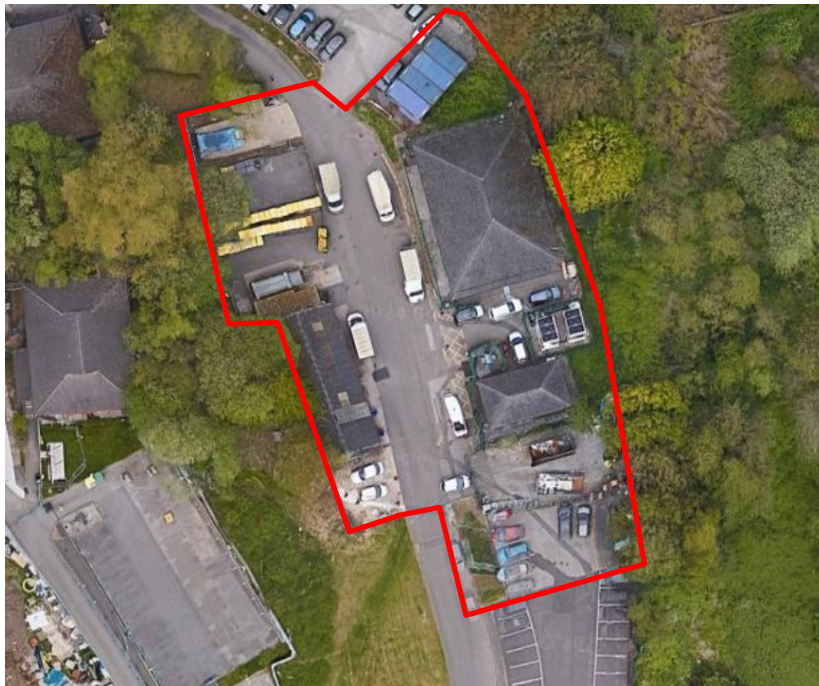
Figure 2.2: Existing Waste Compound at NMGH
