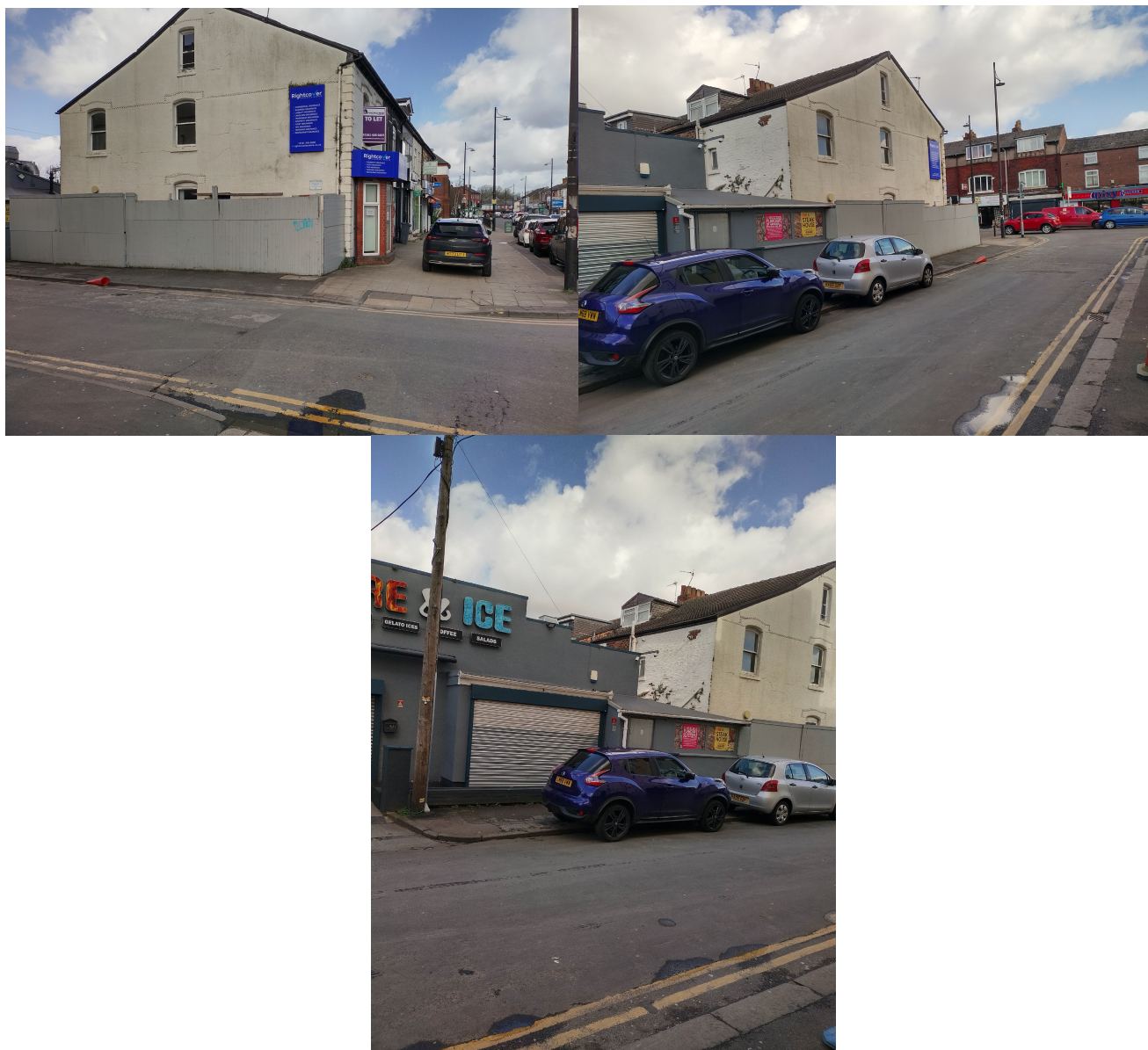
Fig.1 – Views of the applications it from Stockport Road and Western Street
