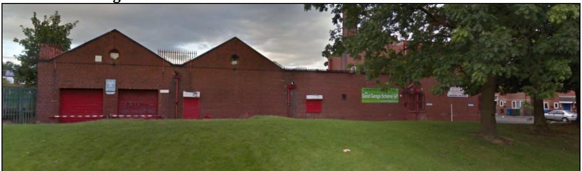
PHOTO 2 -Google Streetview 2012- View S to N
