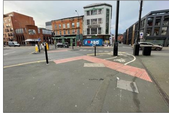
A62 Oldham Road / A665 Ring Road Signalised Junction
