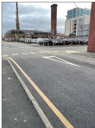
Footway and dropped kerbs / tactile paving provision on Marshall Street and Mason Street
