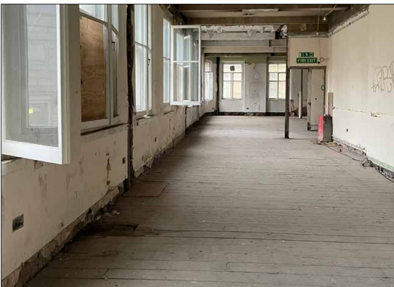
ilmage 46: Photograph showing upper Princess St. section of building with original floorboards.
