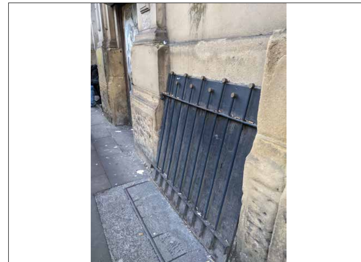
Image 24: Detail of external opening to basement (over-boarded) with railings.
