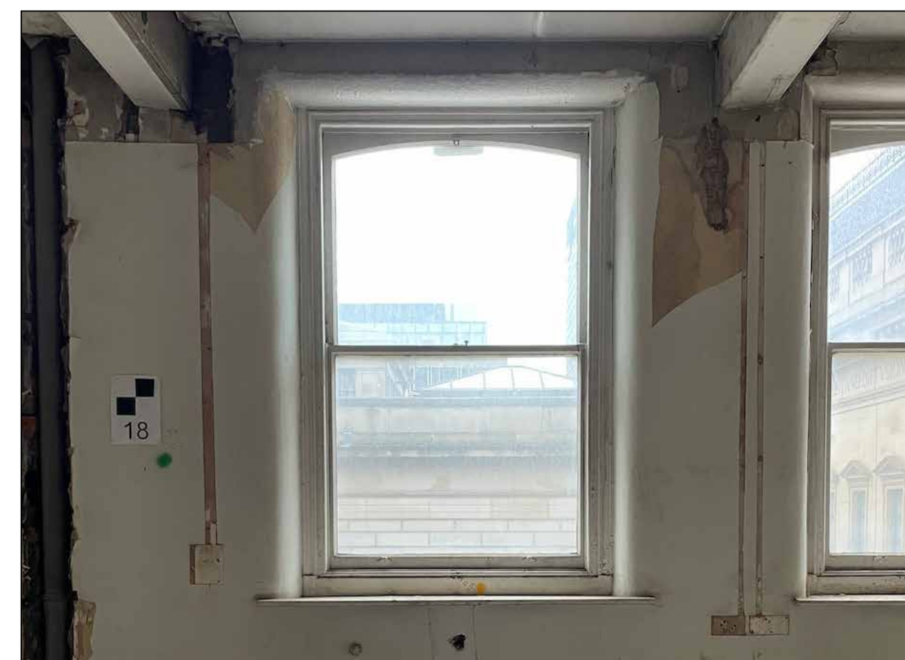
Image 19: Photograph showing typical upper floor one over one sliding sash window to Princess St.
