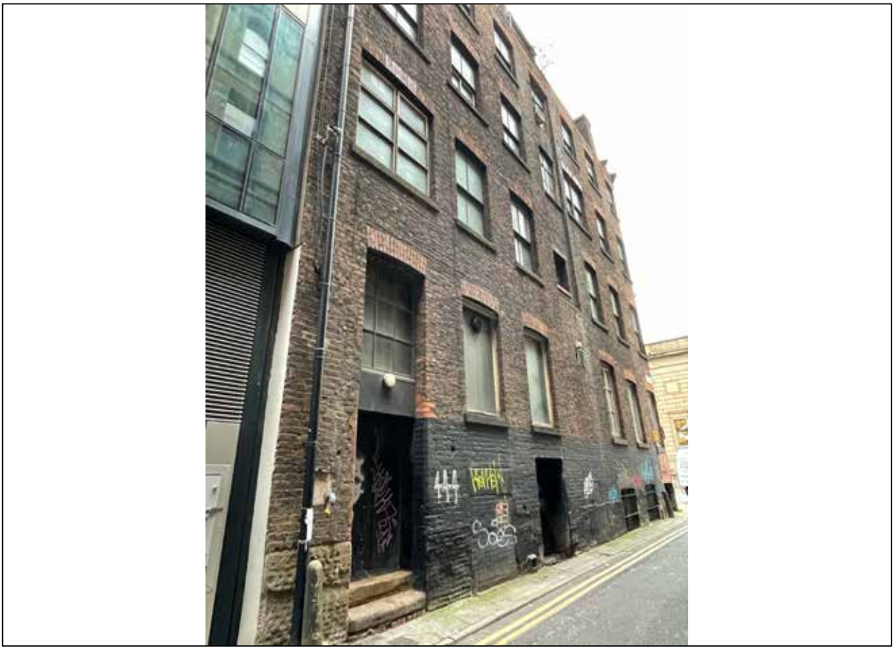
Image 33: View along Back George St. showing doors.
