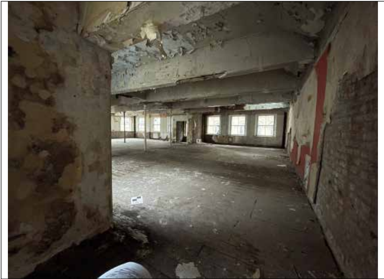
Image 36: View of warehouse side of building with columns and former hoist visible.
