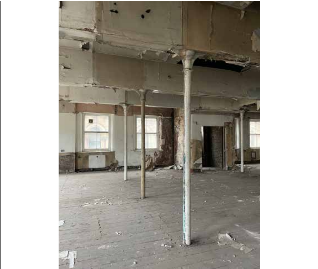
Image 42: View of tight column grid to warehouse space and former hoist to back wall.
