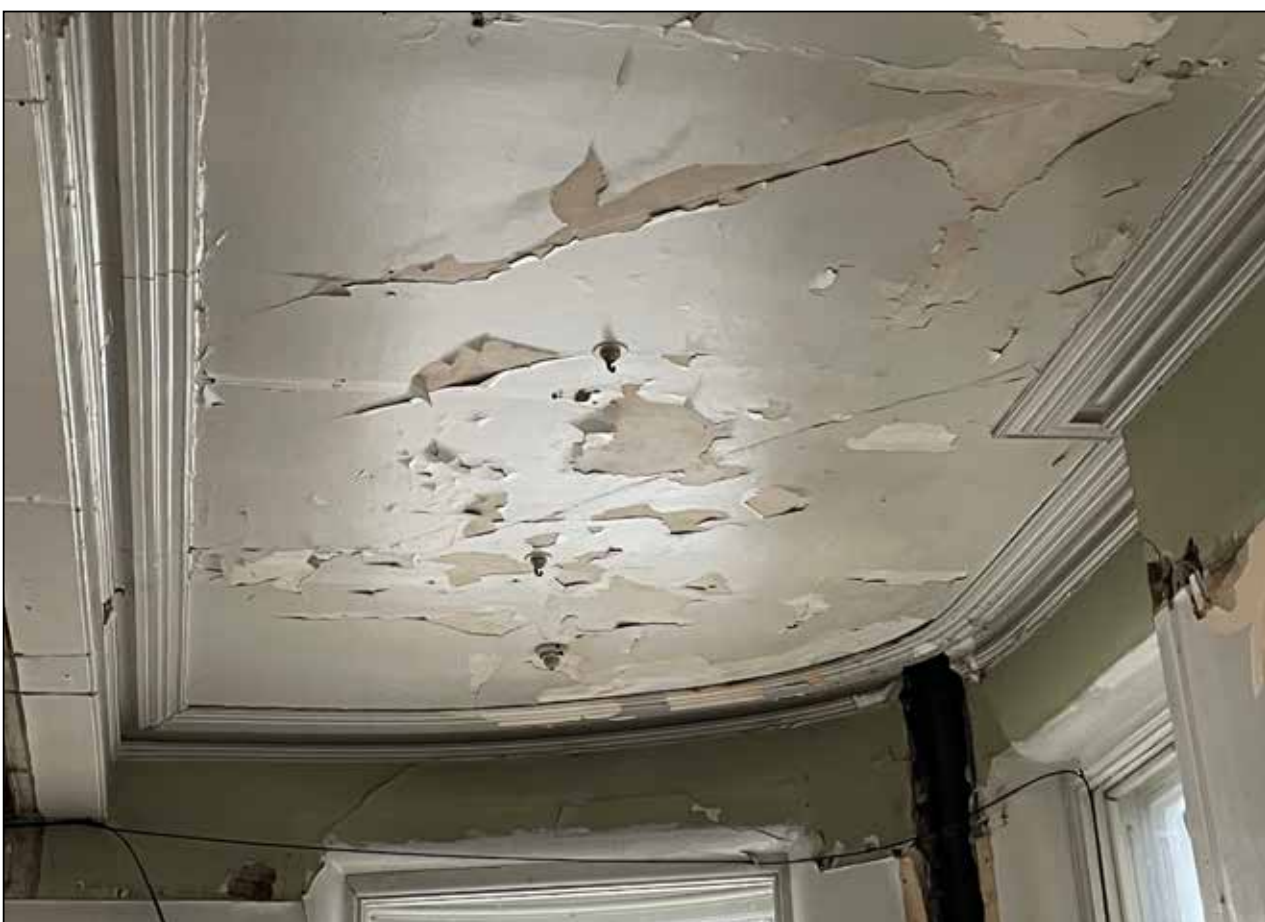
Image 47: First floor example of cornicing to ceiling.
