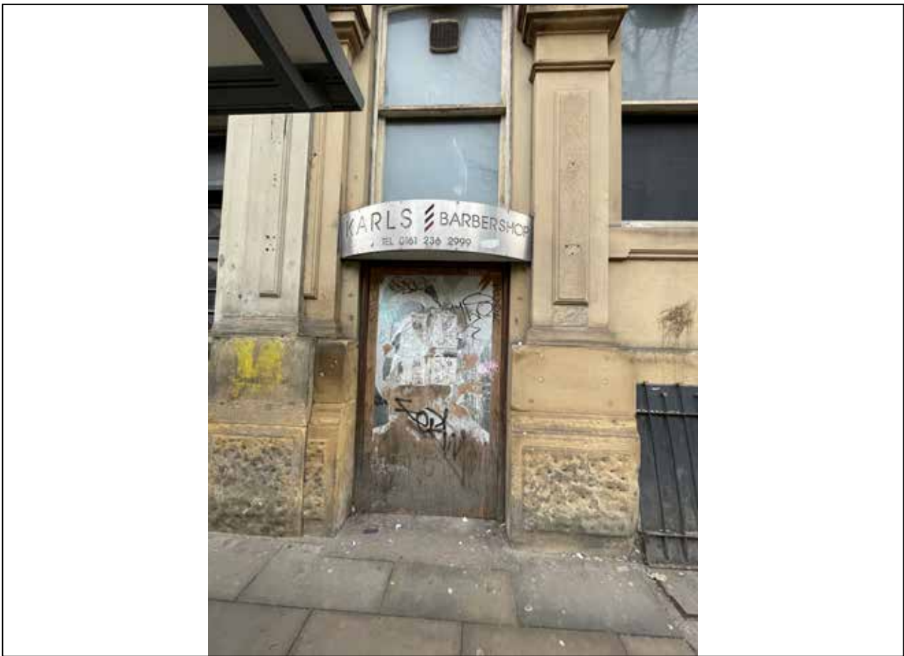
Image 30: Detail of later inserted doorway on Princess St. elevation.
