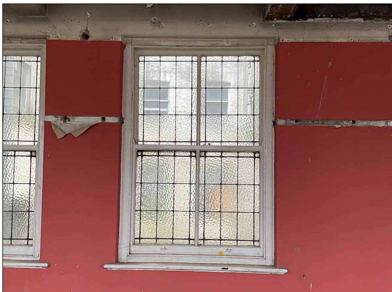
image 14: Photograph showing typical early 20th century leaded windows to lightwell.
