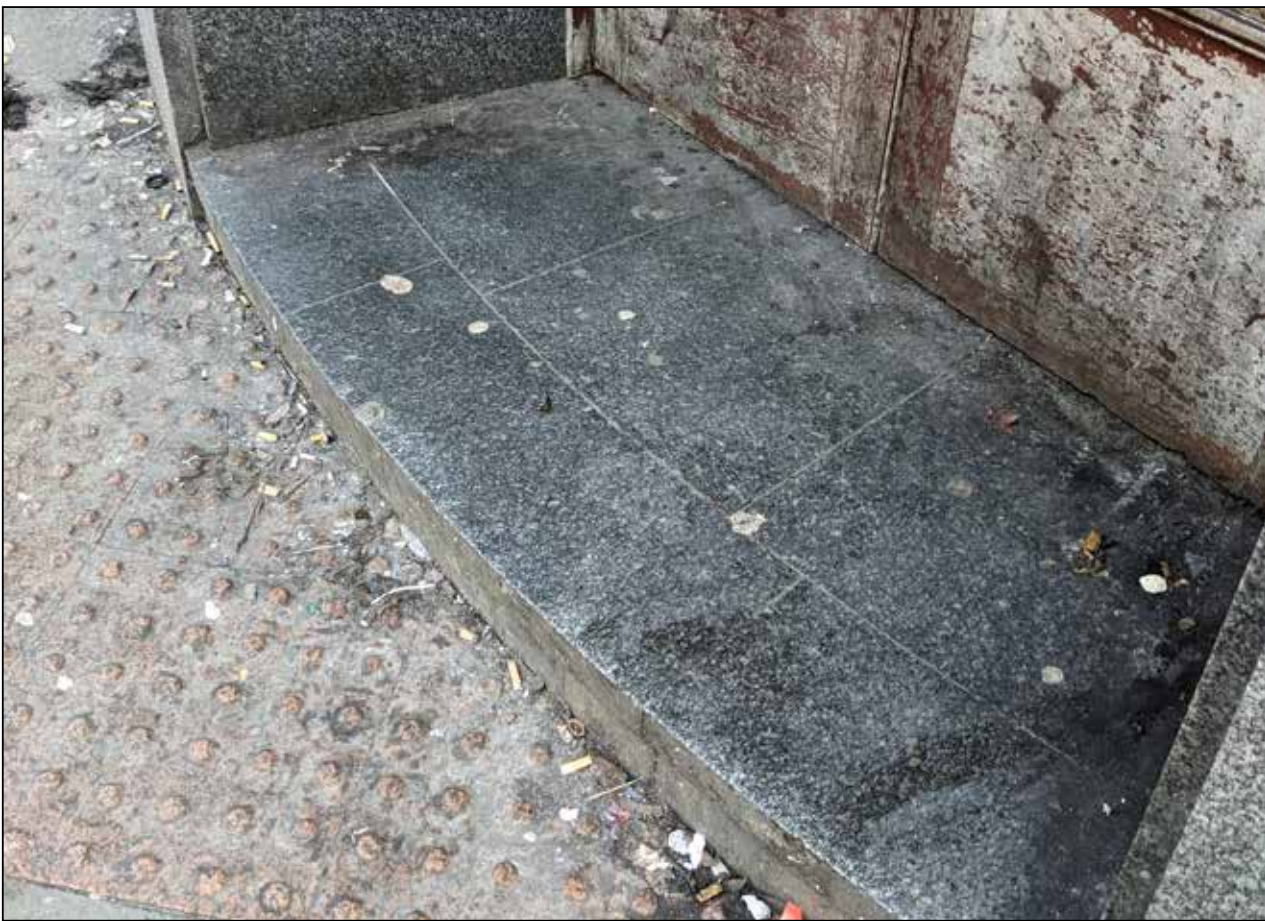
Image 68: Front step to 77 Mosley St. to be replaced with ramp.
