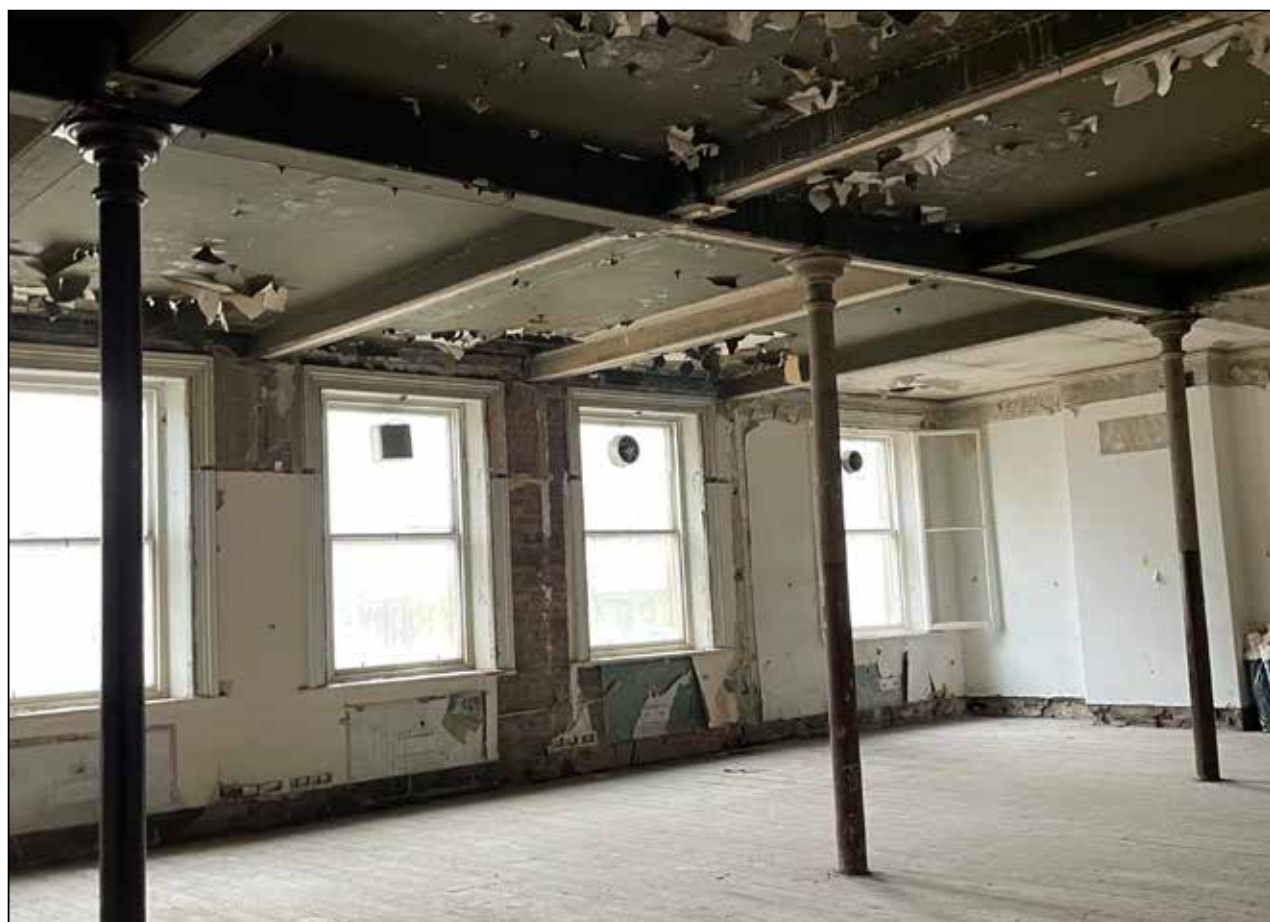
Image 45: First floor windows and columns with exposed heads.
