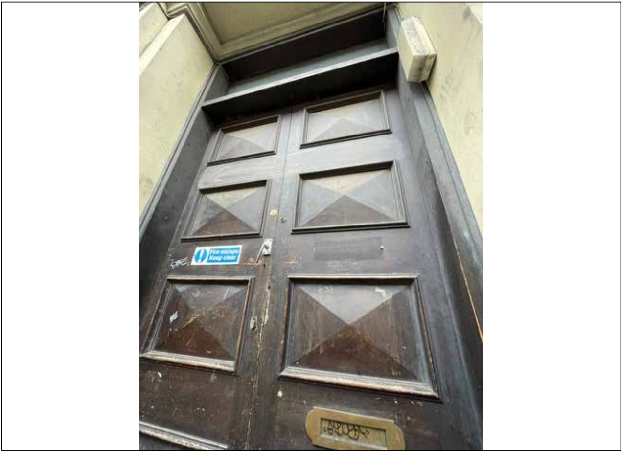
Image 31: Detail of entrance doorway to Princess St. elevation.
