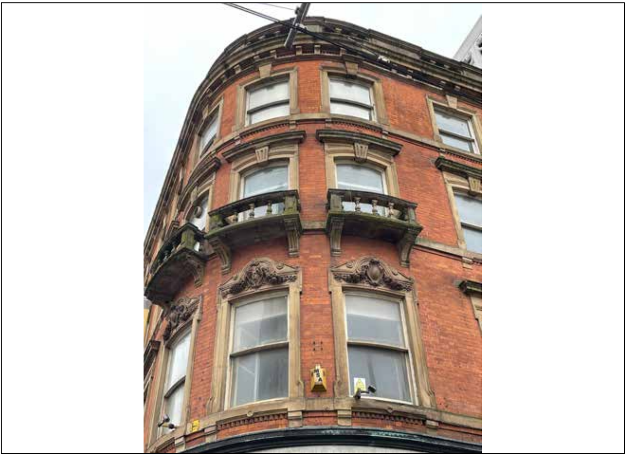
Image 35: Detail of stone decoration and brick elevations to curved Mosley St. corner, showing balconies, windows, and roof level detail.
