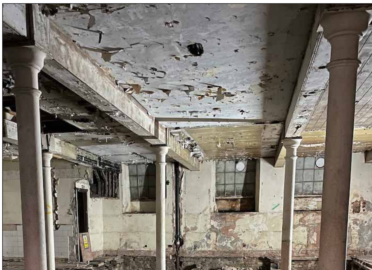
Image 44: Photograph showing basement columns and blocked windows.
