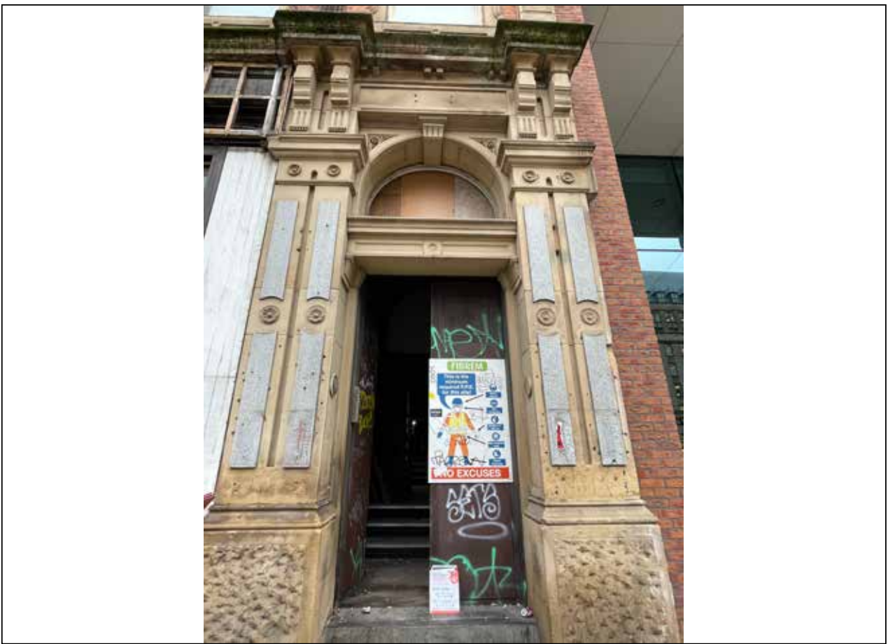
Image 34: Detail of entrance to offices at 79 Mosley Street.
