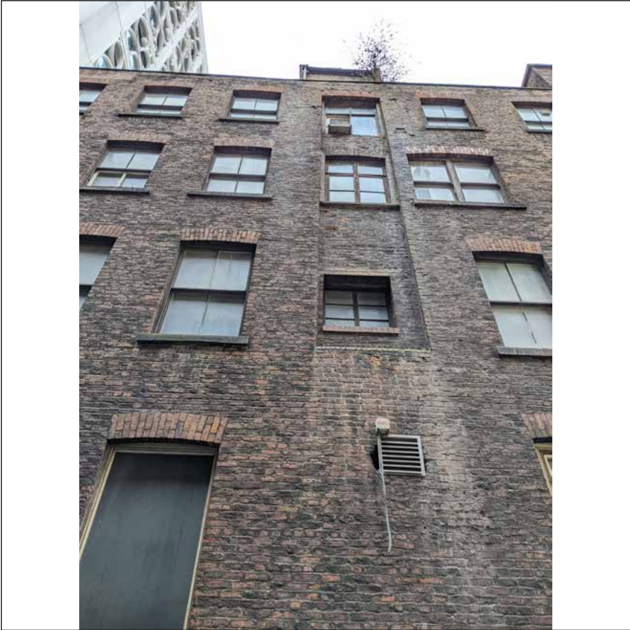
Image 10, 11: View of Princess St. elevation from outside Manchester Art Gallery (top) and detail of former hoist to Back George St. elevation (bottom).
