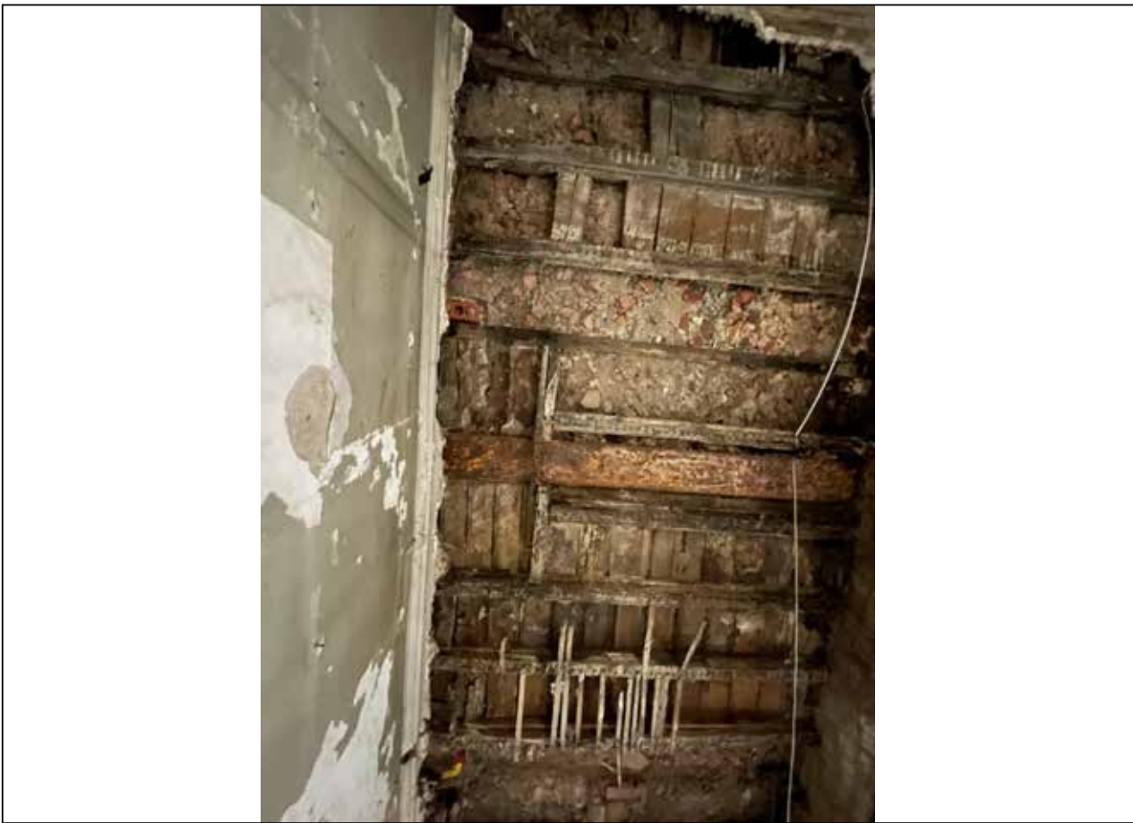
Image 57: Evidence of lath and plaster to ground floor ceiling.
