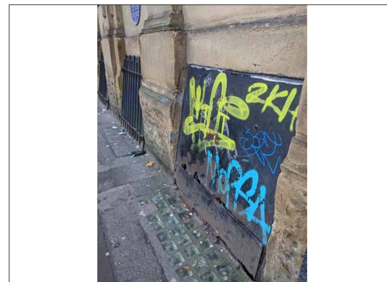
Image 25: Detail of pavement lights to Princess St.
