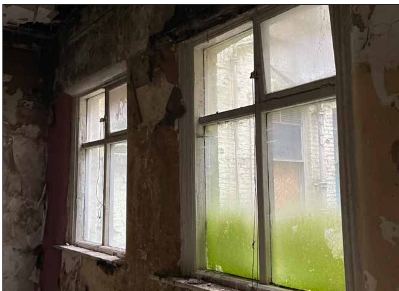
Image 15: Photograph to show later inserted windows to lightwell, upper floor.
