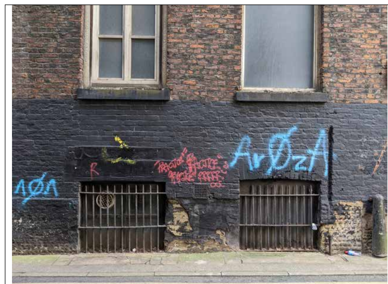
Image 23: Detail on Back George Street elevation showing basement openings and over-painting to brickwork.
