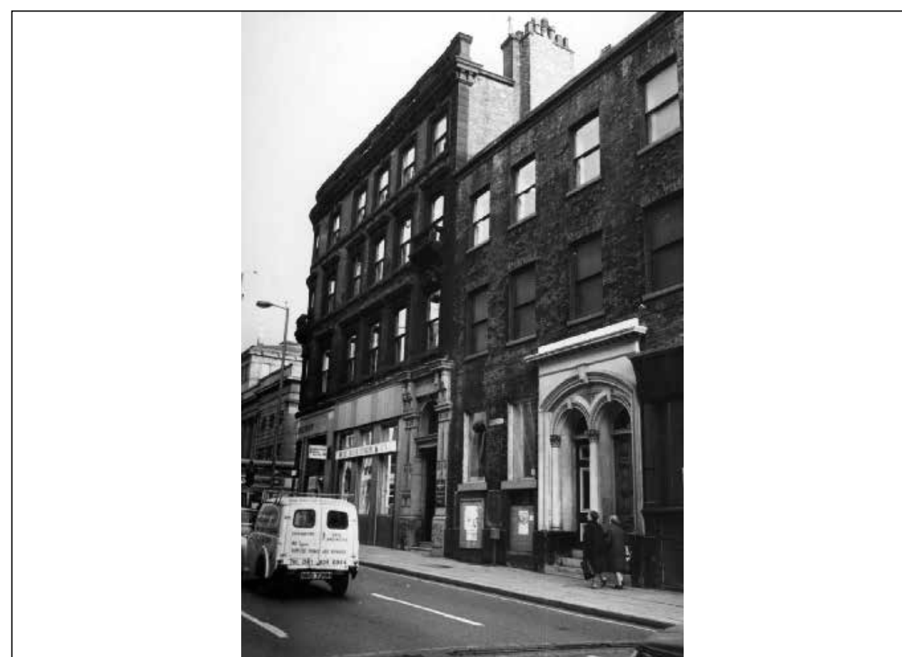
Image 7: Photograph, 1973, showing external view of Mosley St. elevation. Manchester Archives.
