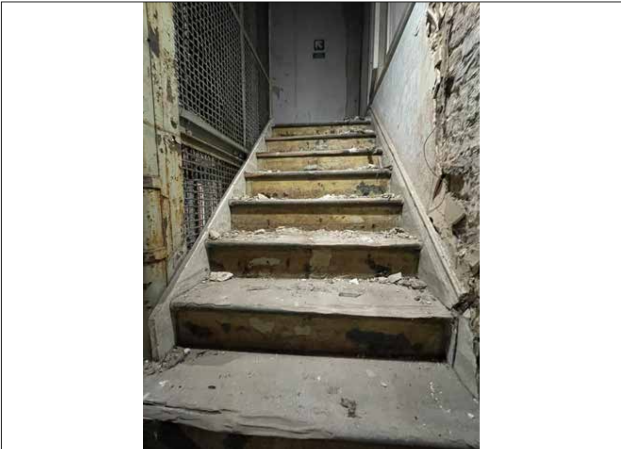
Image 56: Detail of original timber staircase to ground floor, former office side.
