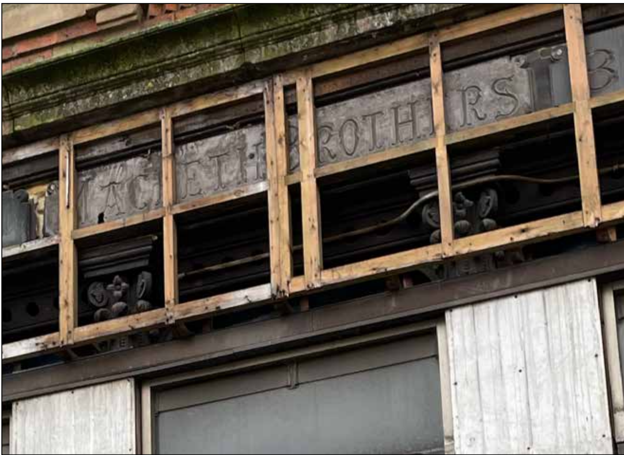
Image 66: Historic shop front to be revealed to former tailors shop on Mosley St.
