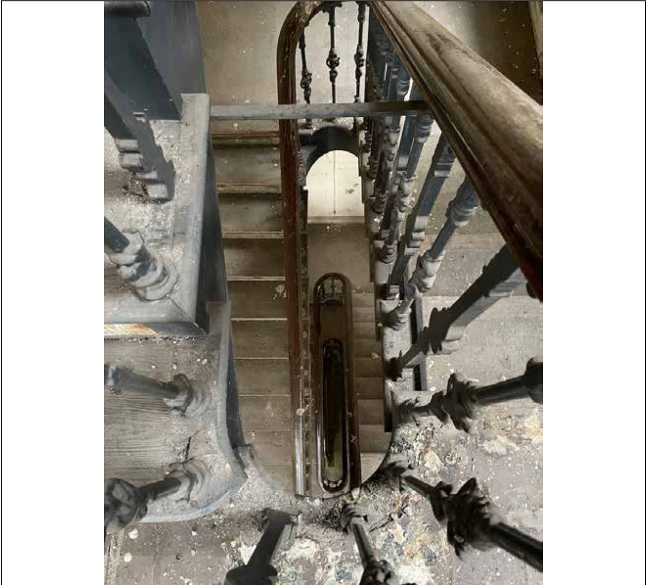
Image 76: Detail of secondary (warehouse) staircase with cast iron balustrade.
