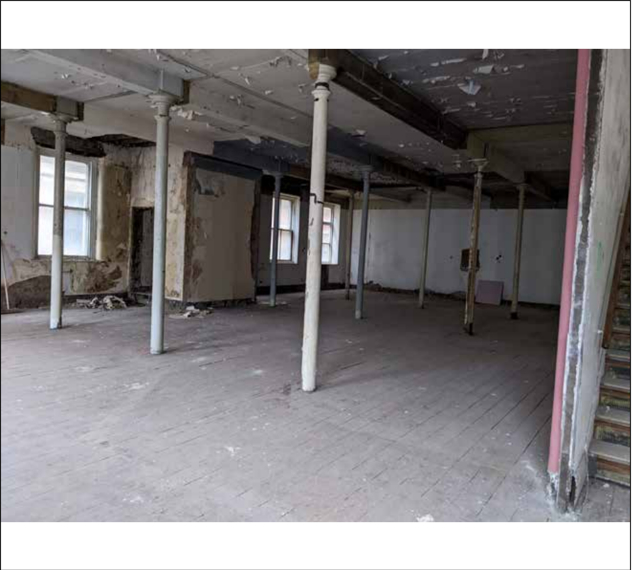
Image 79: Photograph showing internal space to former warehouse. The close knit grid of columns is evident, as is the former hoist which extends into floor space from the Back George St. wall. The warehouse staircase is visible to the right hand side.
