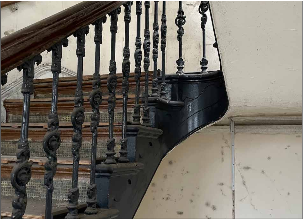
Image 75: Detail of secondary (warehouse) staircase.
