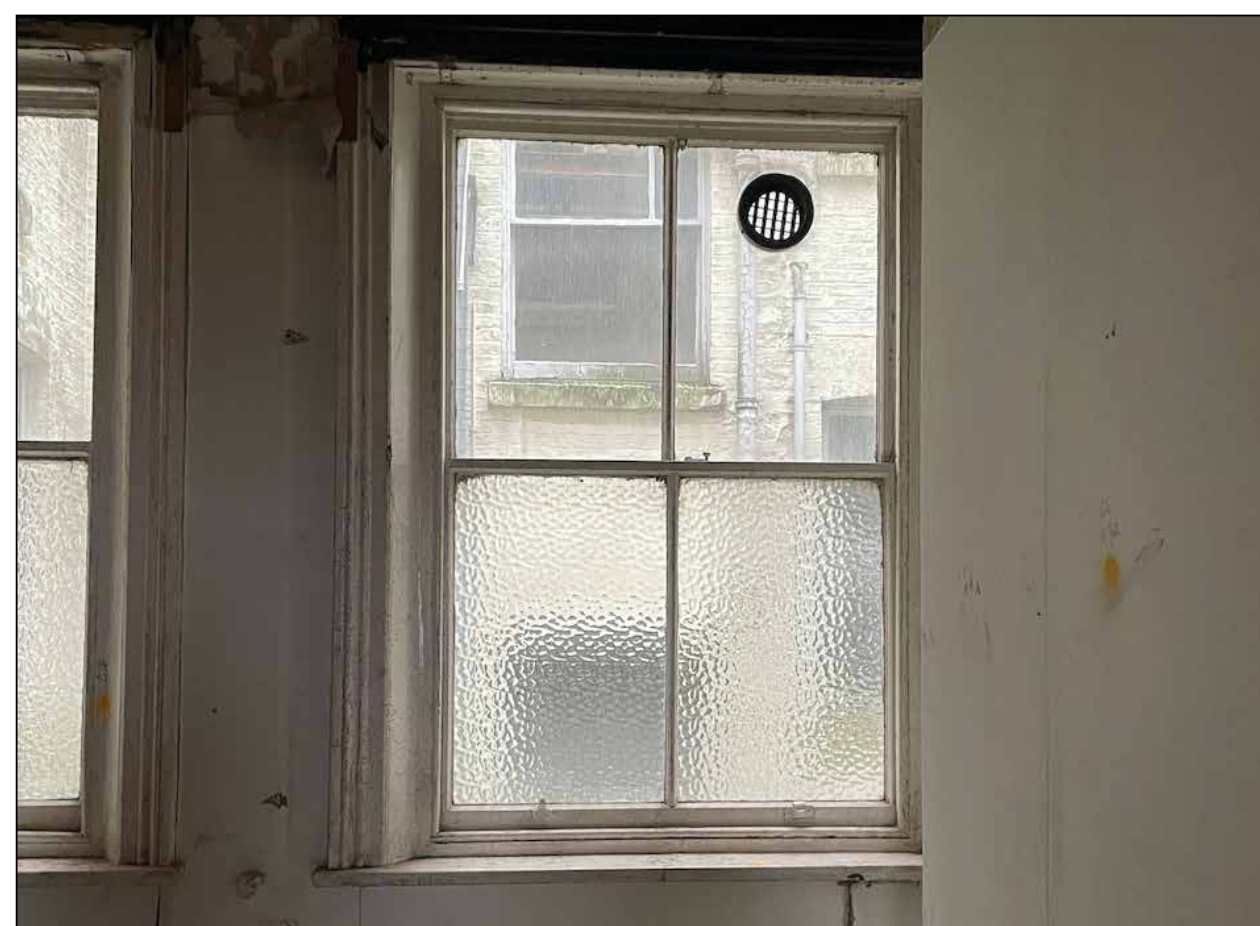
Image 17: Photograph showing example of two over two sliding sash windows to lightwell, with vent hole and obscured glass (later alteration).
