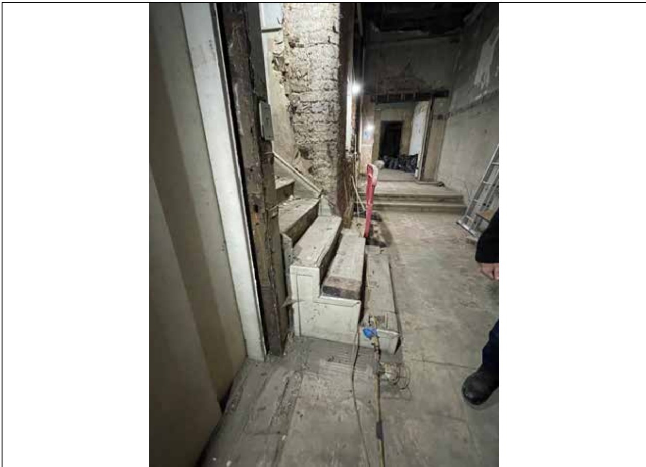
Image 58: Detail of ground floor office stair and further steps (background).
