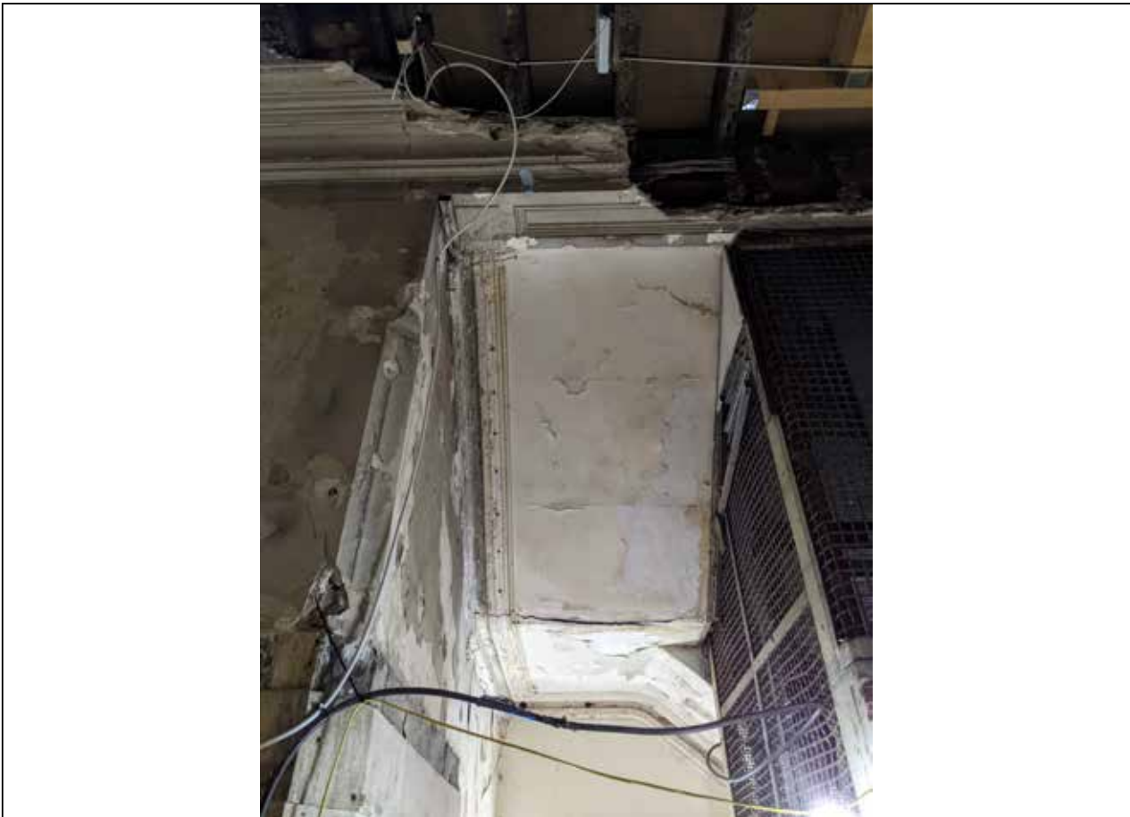
Image 64: Detail of ceiling cornice around lift and office stairs.
