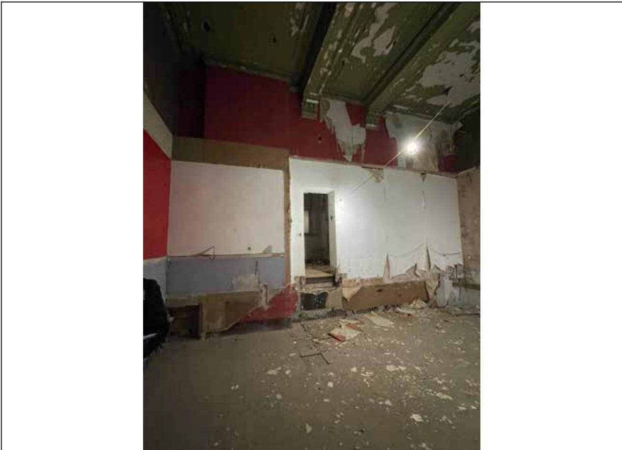
Image 60: View of tall space to ground floor, former shop section.
