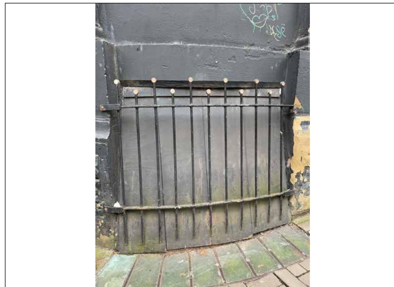
Image 22: Detail of corner of Princess St. showing basement opening and original pavement lights.
