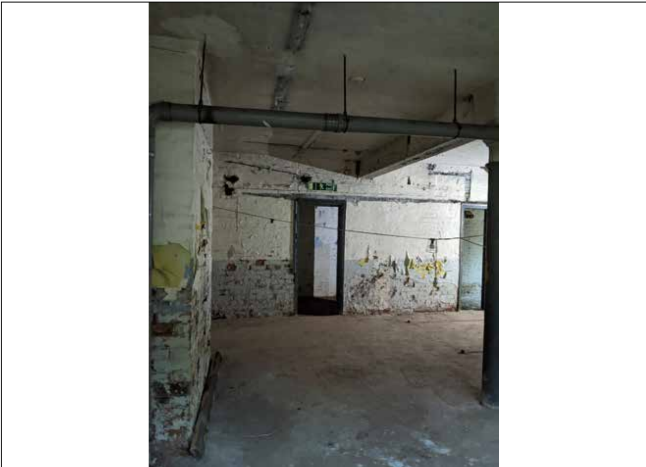
Image 71: Interior view of basement, with chimney breast to left hand side.
