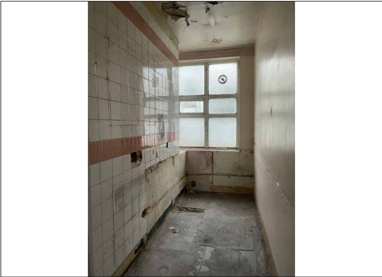
Image 38: An example of modern finishes to typical bathroom/kitchen spaces and altered window to lightwell.
