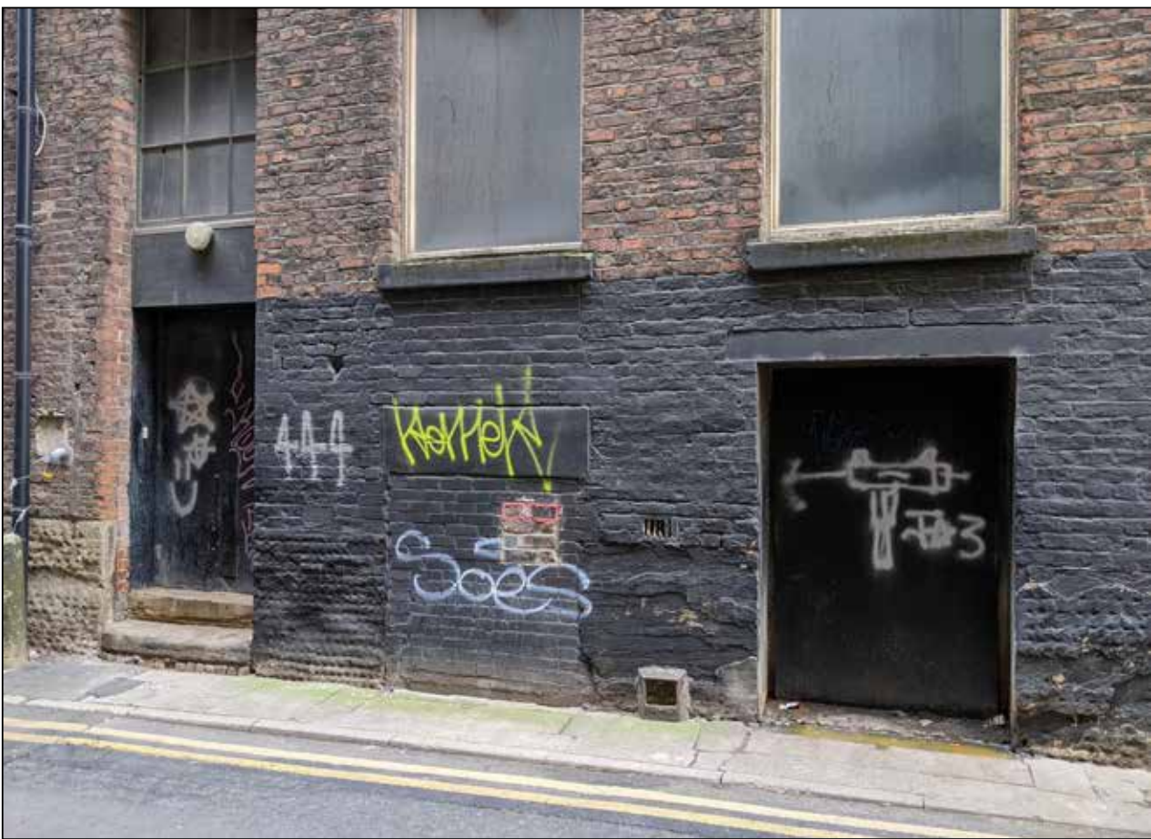
Image 69: Photograph of Back George St. showing existing street scape.
