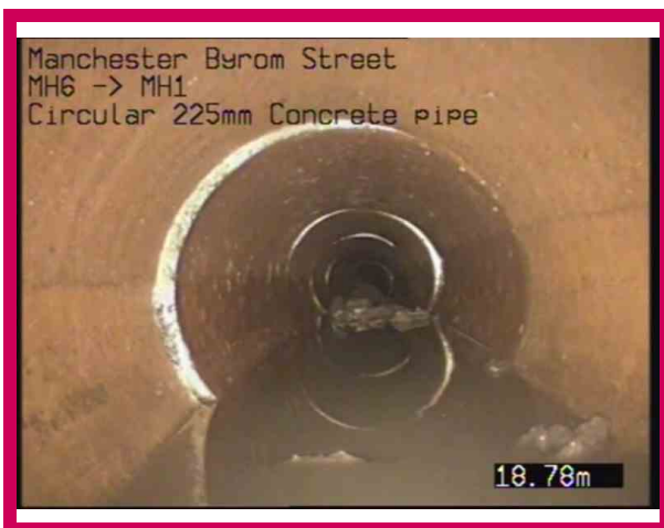
11, 00:01:19, 18.79 m Survey abandoned, Due to debris
