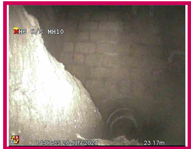
2, 00:05:19, 23.17 m Finish node, other special chamber, reference: MH10, BMH1, buried Manhole, not MH10.
