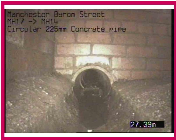
7, 00:02:06, 27.39 m Finish node, manhole, reference: MH14
