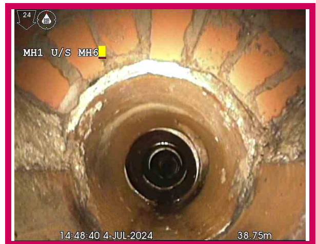
4, 00:04:50, 38.75 m Finish node, manhole, reference: MH6
