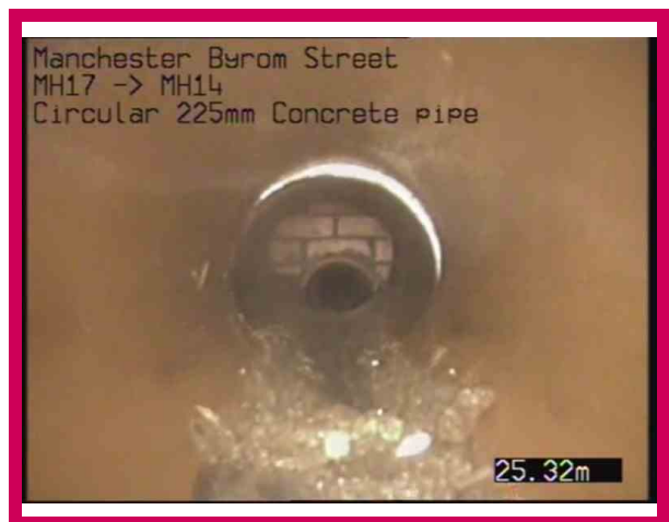
6, 00:01:58, 25.32 m Settled deposits, fine, 10% cross-sectional area loss
