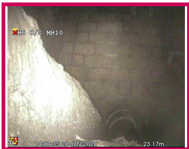
5, 00:05:19, 23.17 m Finish node, other special chamber, reference: MH10, BMH1, buried Manhole, not MH10.
