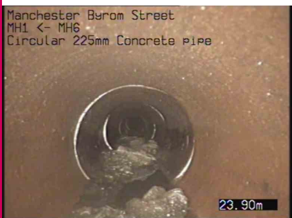
15, 00:02:16, 23.90 m Survey abandoned, Due to debris
