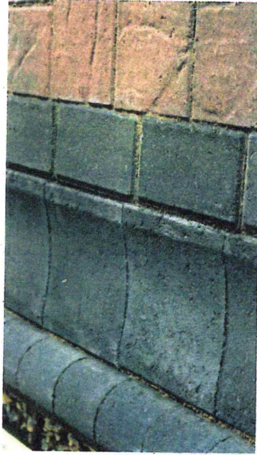
Driveline Drainage Channel
