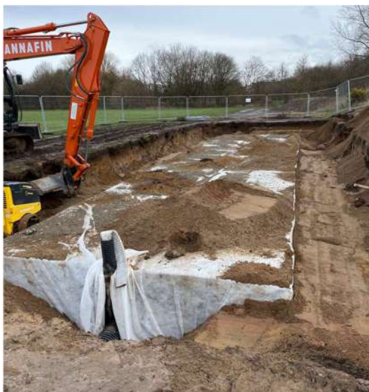
Figure 1 – Attenuation Tank Installation
