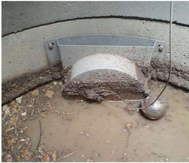
Figure 2 – Flow Control Installation
