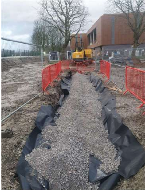
Figure 5 – Swale Installation
