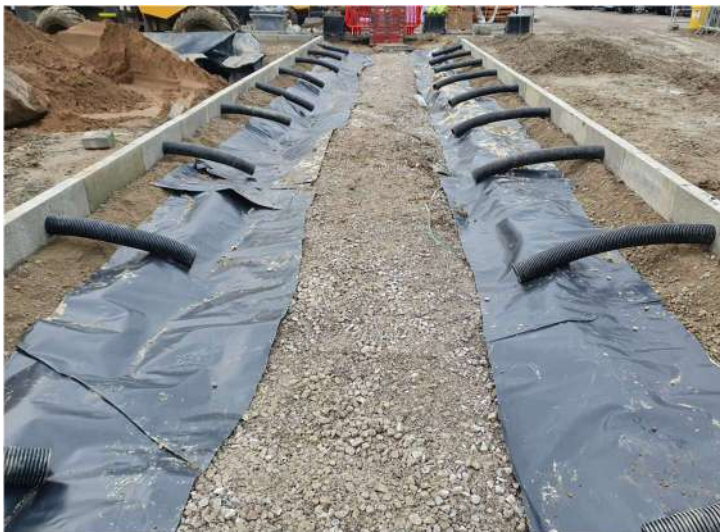
Figure 5 – Swale Installation
