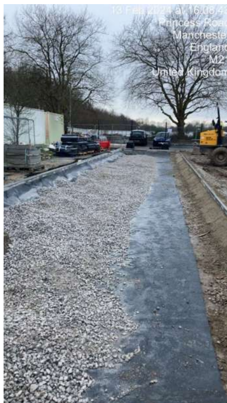
Figure 3 – Permeable Paving Installation
