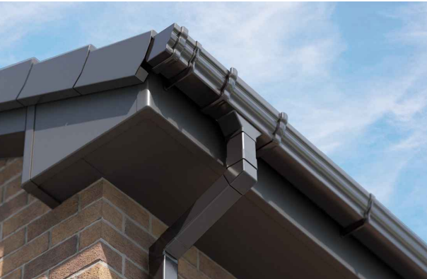
05. Gutter, Fascia and Soffit in Black colour
