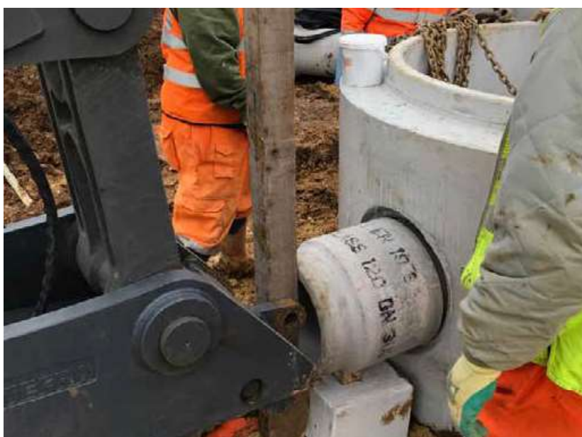
Double Spigot Pipe connected into a Perfect Base™
