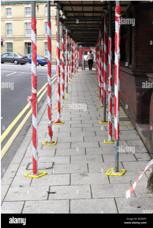
Figure 3 - An example of the gantry scaffolding.
