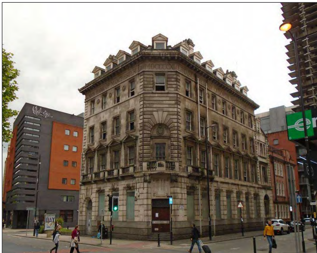
Plate 2: The Grade II listed former bank occupying the northern part of the Site Area
