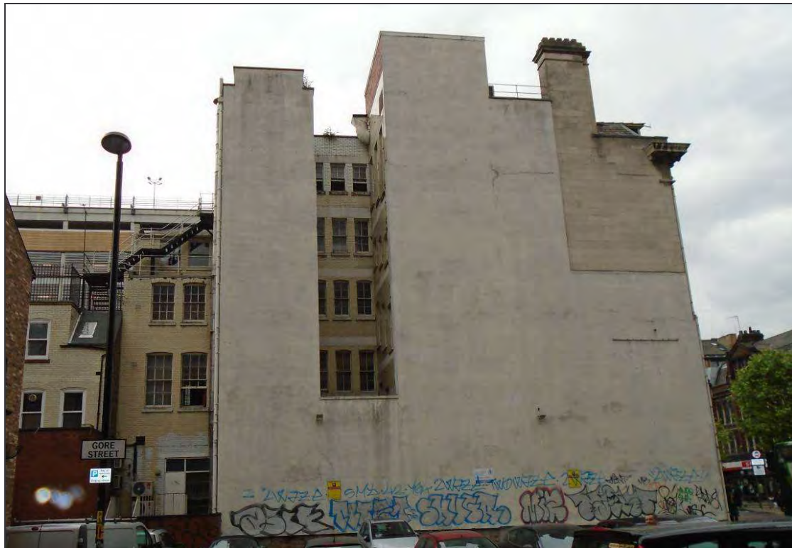
Plate 3: The south-east-facing elevation of the Grade II listed building
