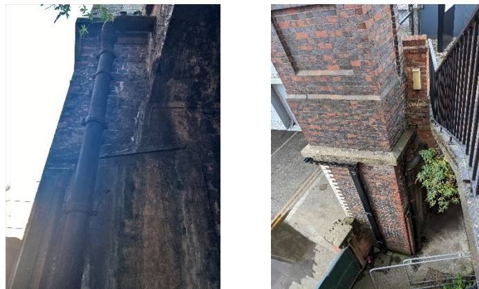
Figure 3—7 Downpipe from station viaduct
