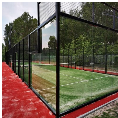
Padel court external materials: Steel frames, tempered glass and monofilament turf
