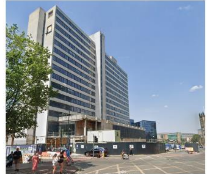
1. View of the site from the junction of Deansgate and Blackfriars street.
