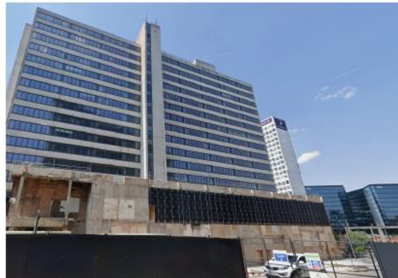
2. Existing view along Deansgate on Eastern boundary of the site.
