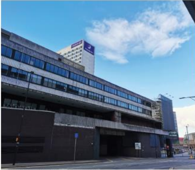
4. View from Deane Gate to existing service yard entrance
