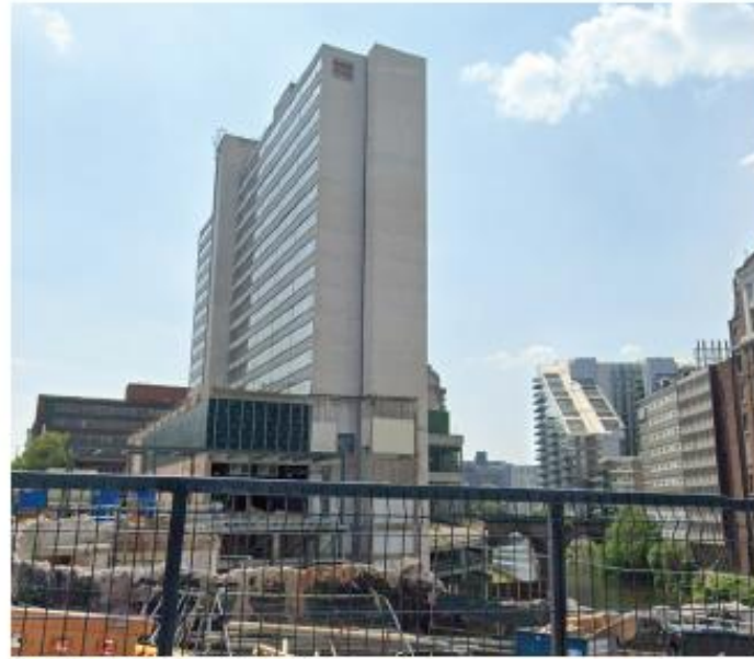
5. North view of site from Victoria Bridge Street.
