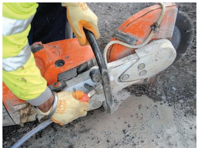
Figure 3 Water suppression on a cut-off saw
