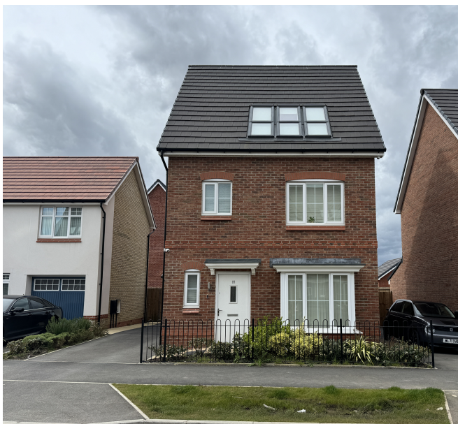
Figure 1. Front view of the property.
