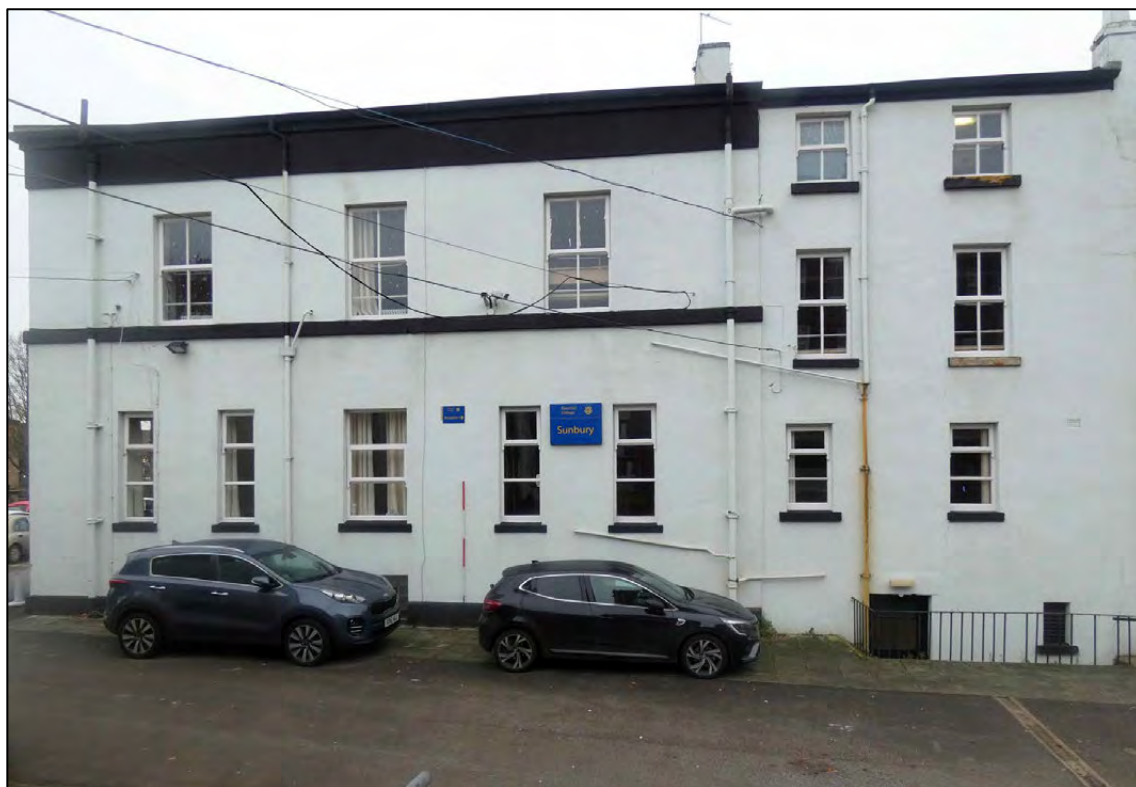
Appendix 2.8: General view of east elevation looking west (D9) (Scale 2m)
