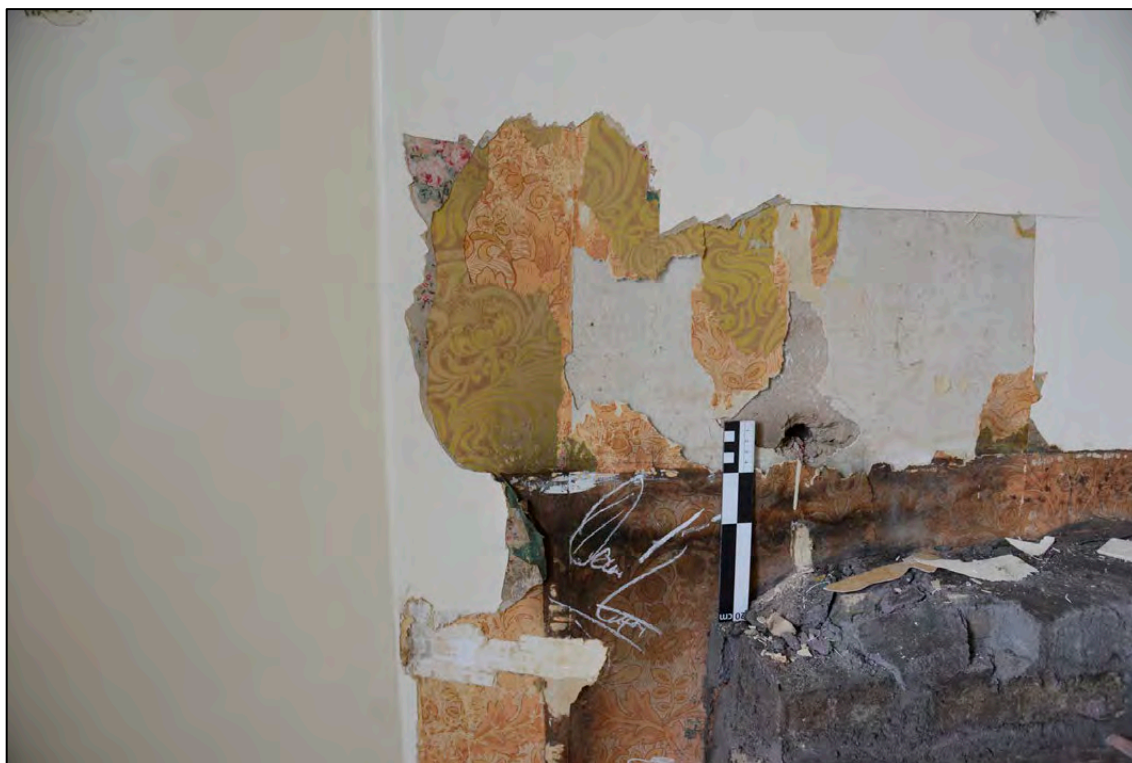
Appendix 2.70: GII Detail of wallpaper revealed behind chimneypiece during SWB looking N (D189) (Scale 20cm)
