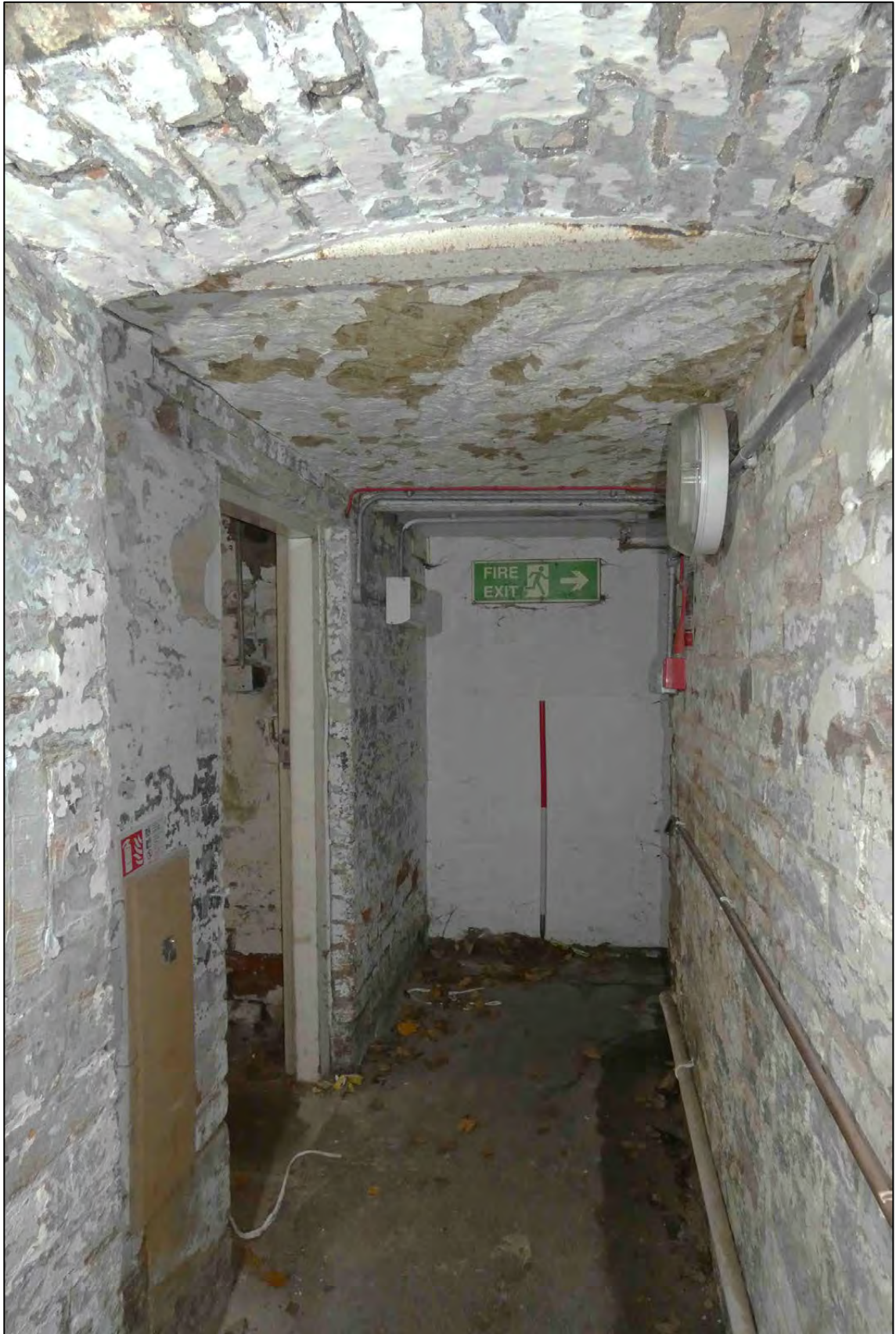
Appendix 2.27: General view B9 (D172) (Scale 1m)
