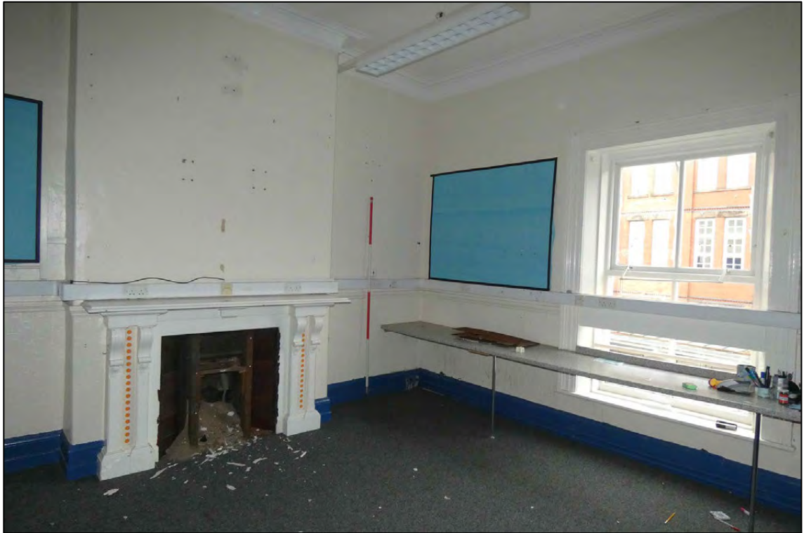
Appendix 2.94: General view of north and east wall F7 (D53) (Scale 2m)
