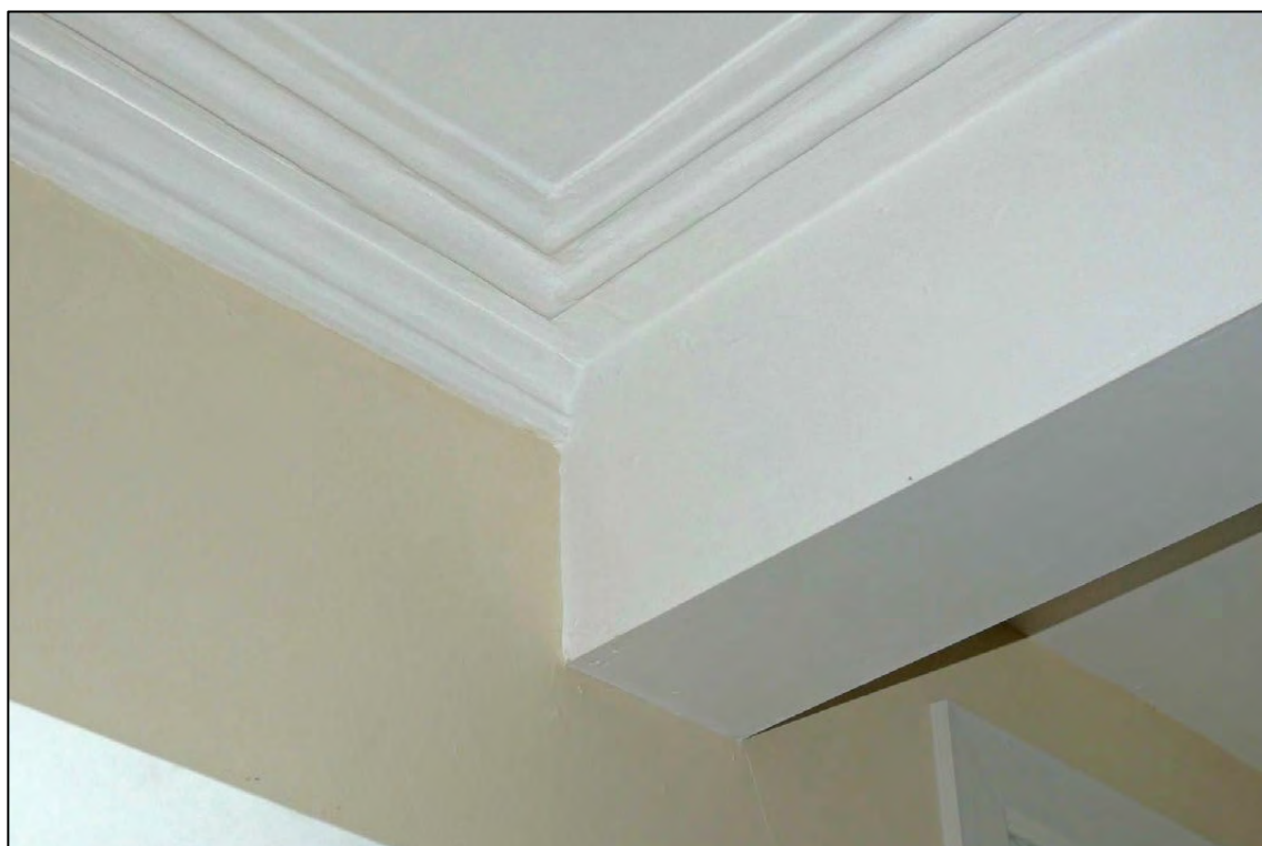
Appendix 2.75: Detail of ceiling and possible inserted RSJ G14 (DI13)
