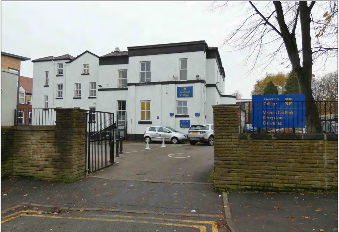
Appendix 2.3: Entrance from Thurloe Street looking east (D3) (Scale 2m)
