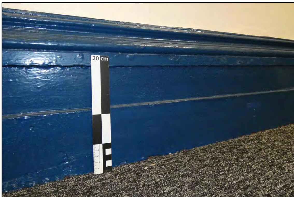
Appendix 2.67: Detail of skirting board on east wall G11 (DI38) (Scale 20cm)
