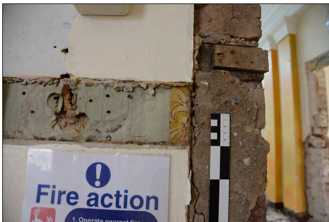
Appendix 2.105: F3 Detail of wallpaper on north wall during SWB looking N (D185) (Scale 10cm)
