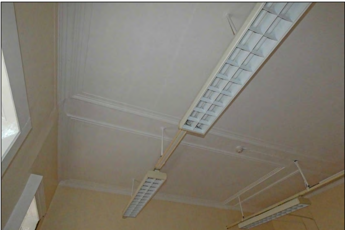
Appendix 2.81: General view of ceiling G12 (DI22)
