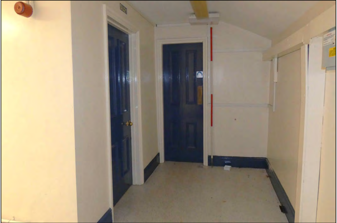
Appendix 2.138: General view from S5 looking towards doorways to S6 and S7 (D18)
