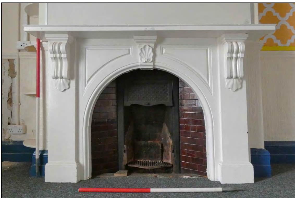
Appendix 2.119: General view of fireplace F2 (D94) (Scale 1m)
