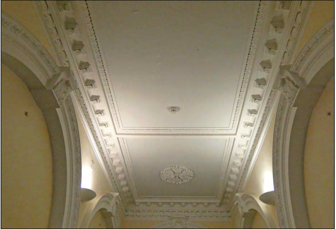
Appendix 2.37: General view of ceiling G4 (DI32)
