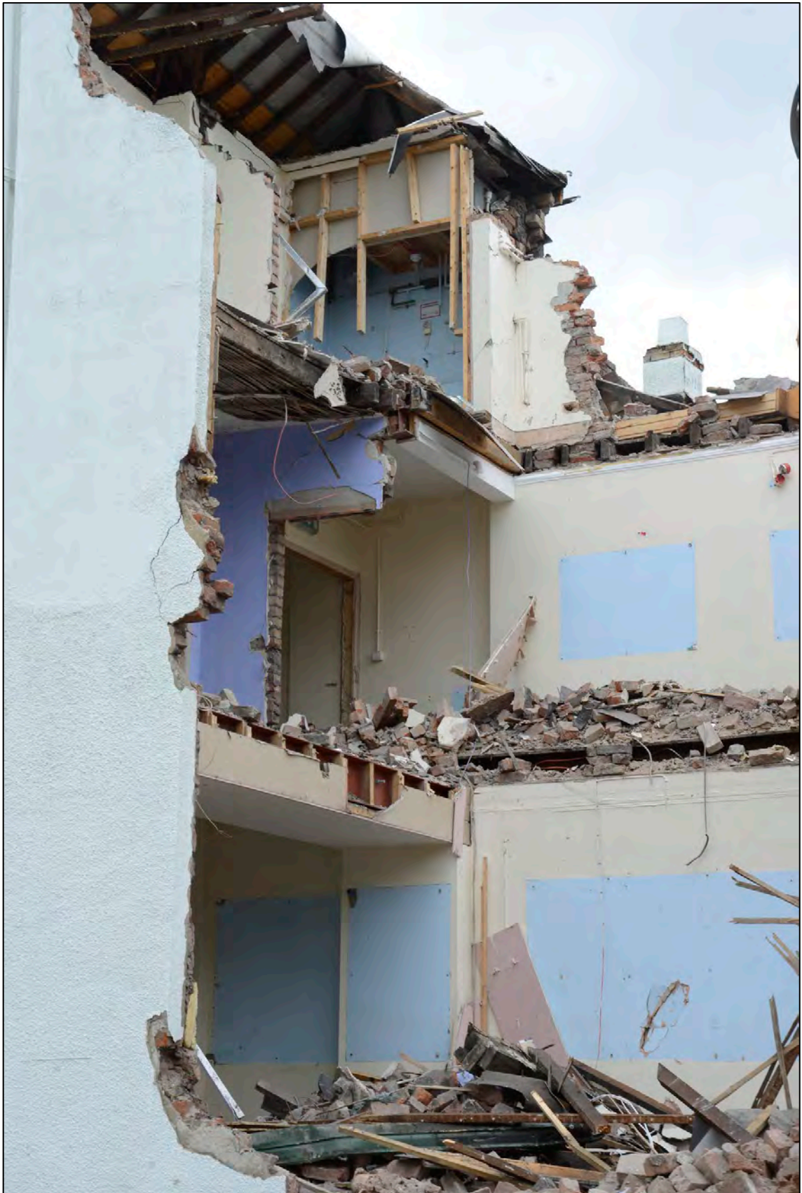
Appendix 2.147: General view of inserted RSJs at junction of Ancillary Range and Extension looking NE (D193) (Scale N/A)
