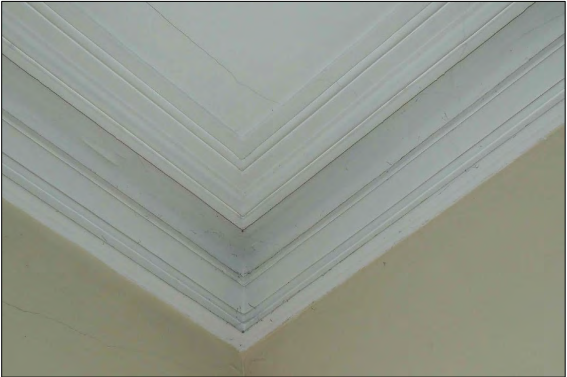
Appendix 2.114: Detail of coving in north west corner of F3 (D70)
