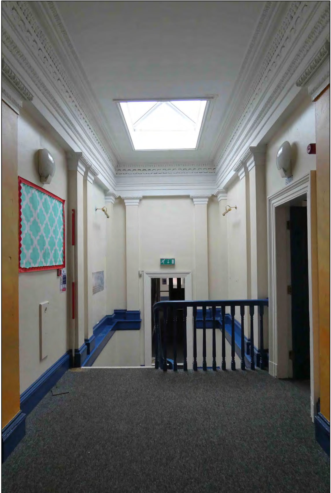
Appendix 2.88: General view of stairwell looking north F1 (D51) (Scale 1m)
