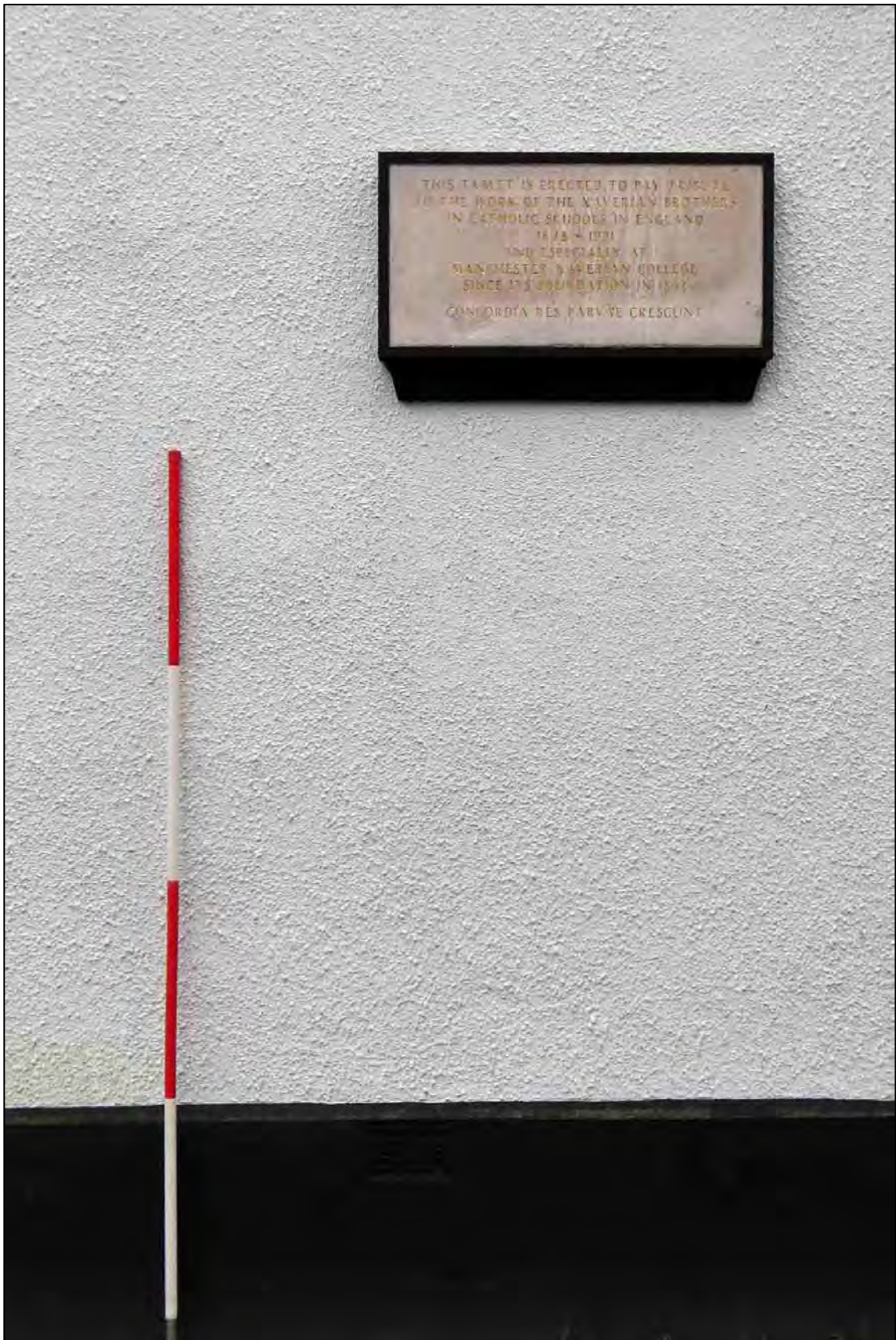
Appendix 2.12: Detail of plaque in north facade (D13) (Scale 2m)
