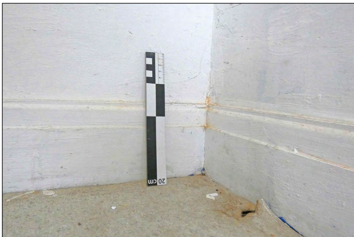
Appendix 2.130: Detail of skirting boards in north-east corner F5 (D92) (Scale 20cm)
