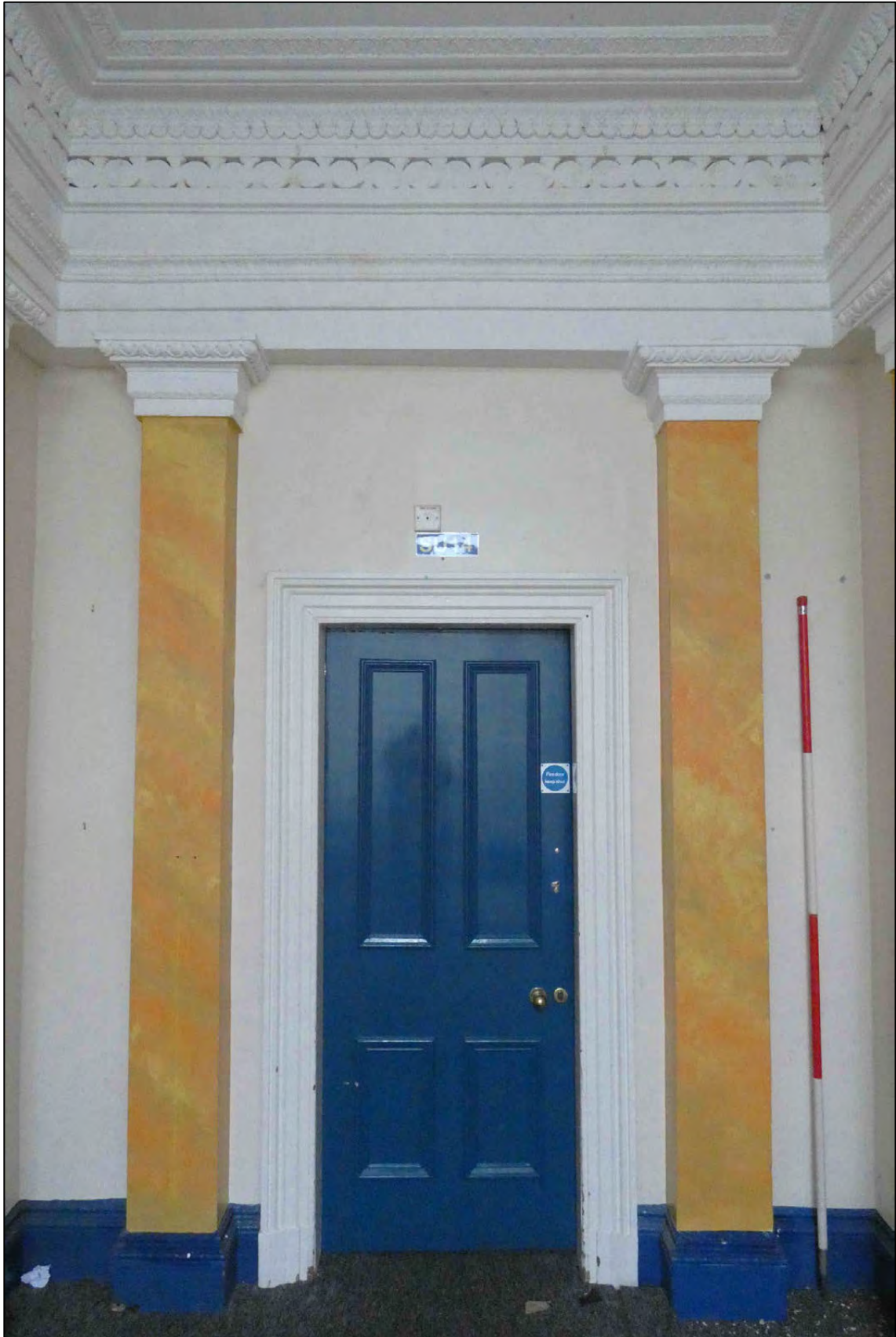
Appendix 2.89: General view of doorway F1 to F3 looking south (D48) (Scale 2m)
