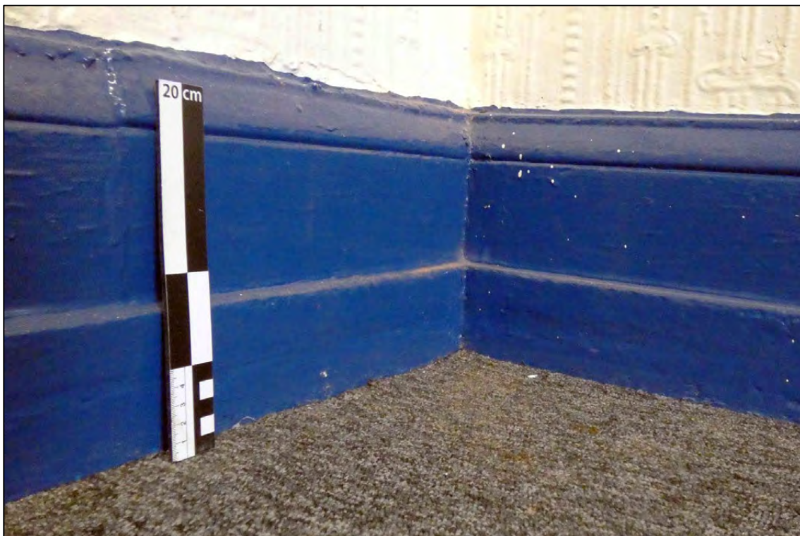
Appendix 2.96: Detail of skirting board in north west corner F7 (D56) (Scale 20cm)
