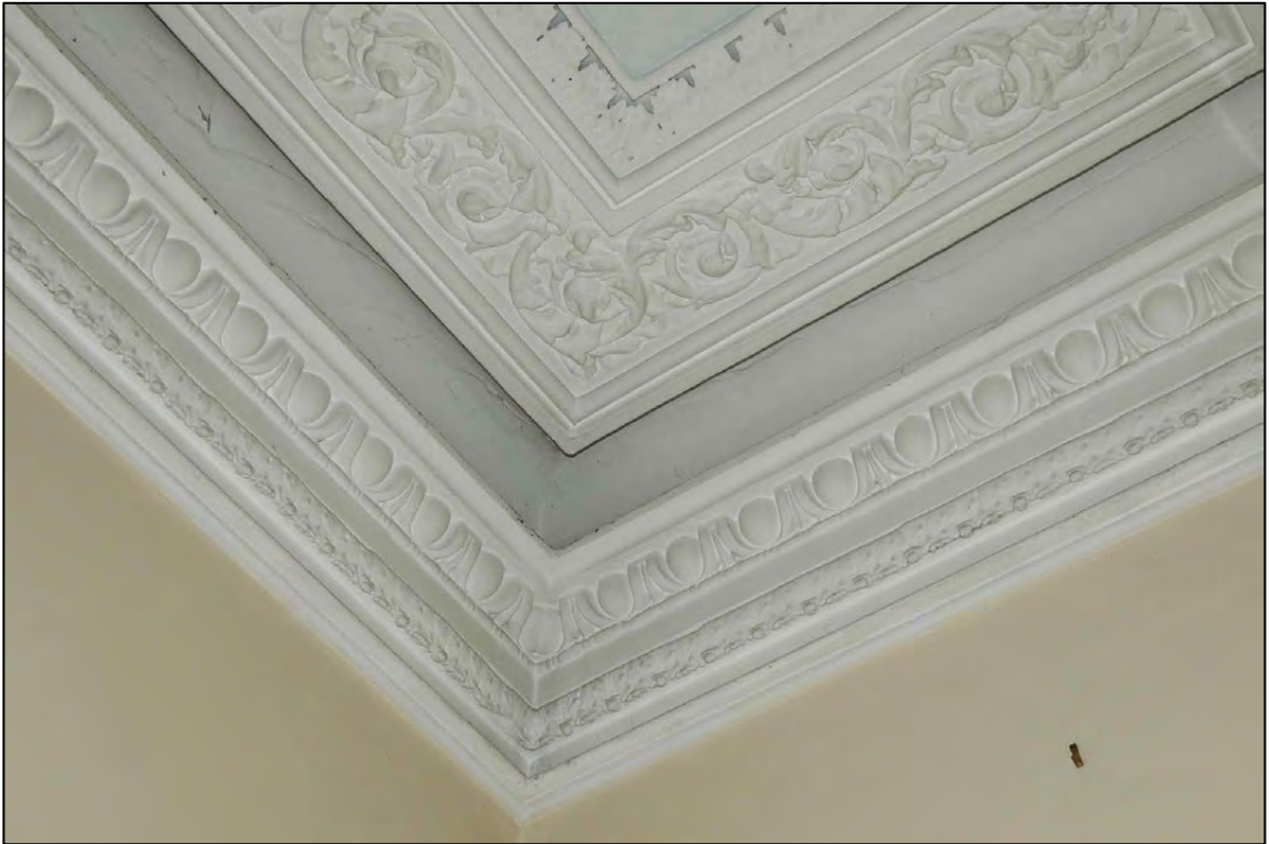
Appendix 2.62: Detail of coving in south-west corner G9 (DI45)
