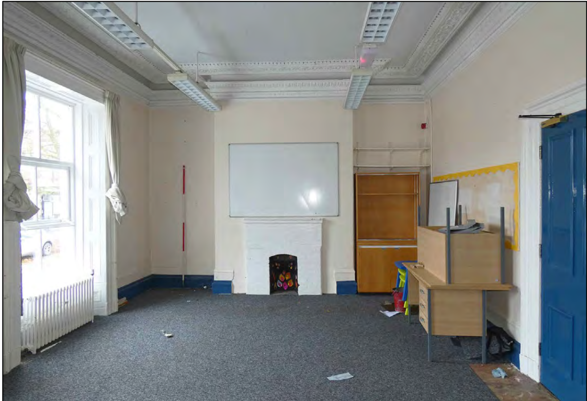
Appendix 2.57: General view G9 looking towards fireplace on west wall (D140) (Scale 2m)
