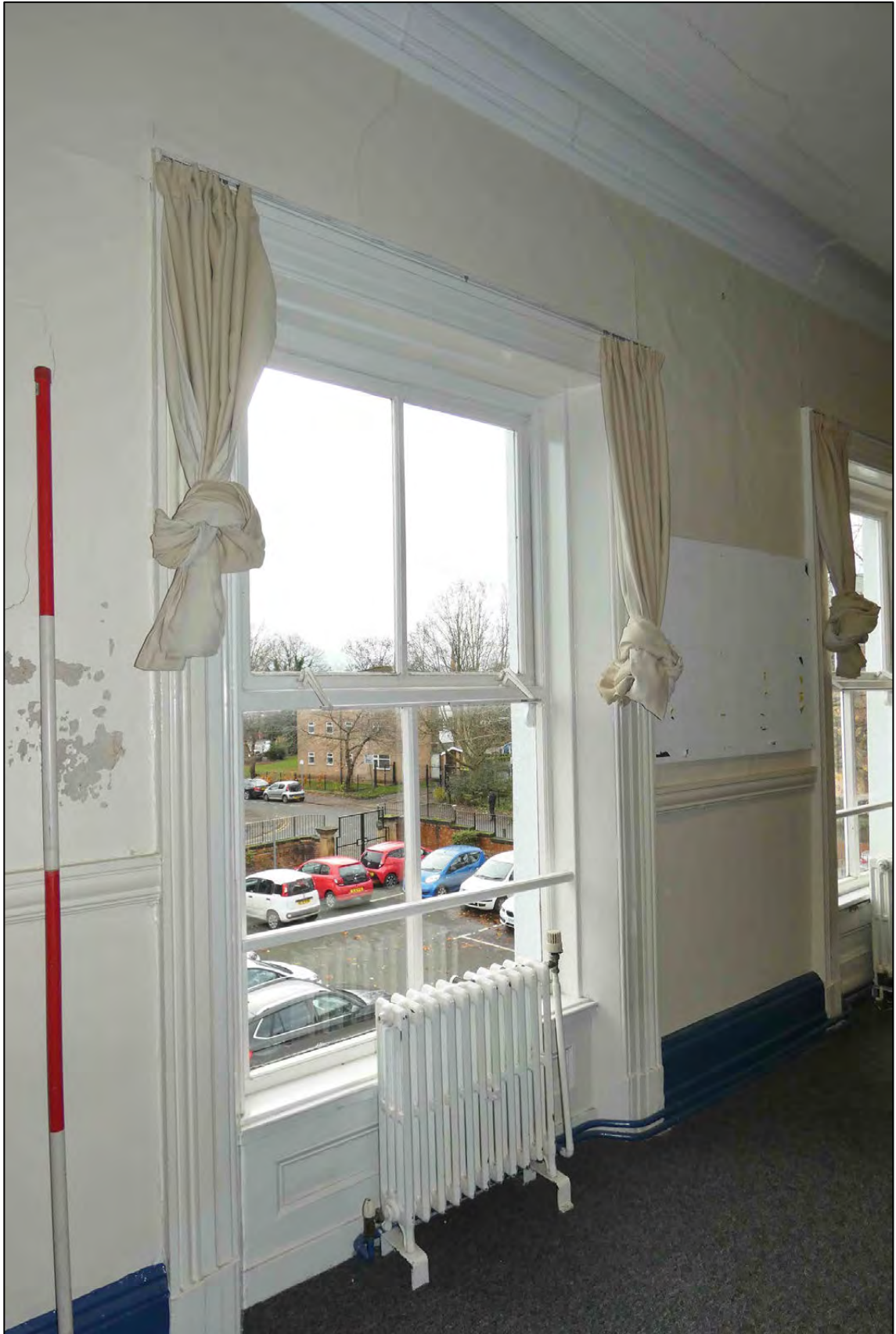
Appendix 2.112: Detail of window in south wall F3 (D63) (Scale 2m)
