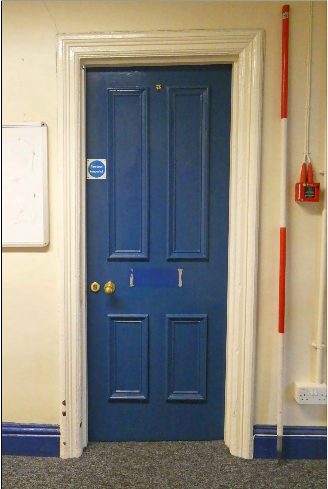
Appendix 2.134: Detail of doorway from F10 to F12 (D32) (Scale 2m)
