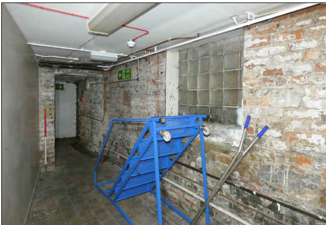
Appendix 2.20: General view B8, looking north(D171) (Scale 1m)
