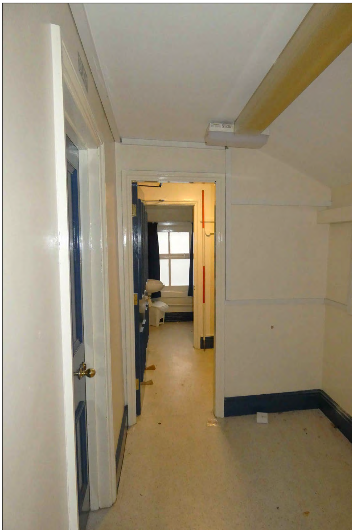
Appendix 2.137: General view looking east into S7 and S8 (D17) (Scale 2m)
