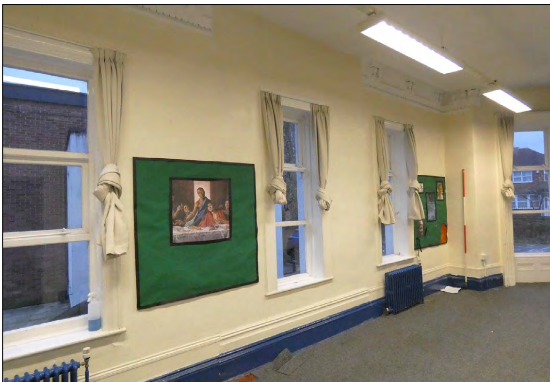
Appendix 2.48: General view of east wall G10 (DI48) (Scale 2m)
