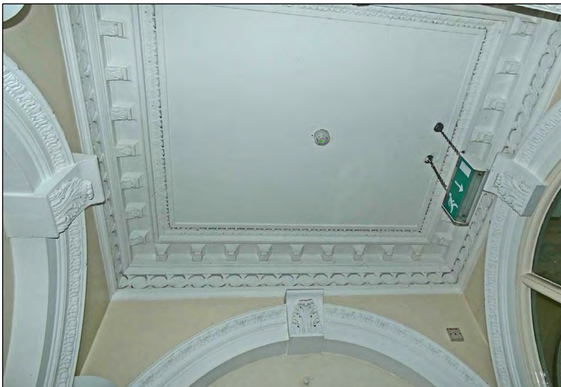
Appendix 2.41: General view of ceiling and arch details in G5, looking south (D126)
