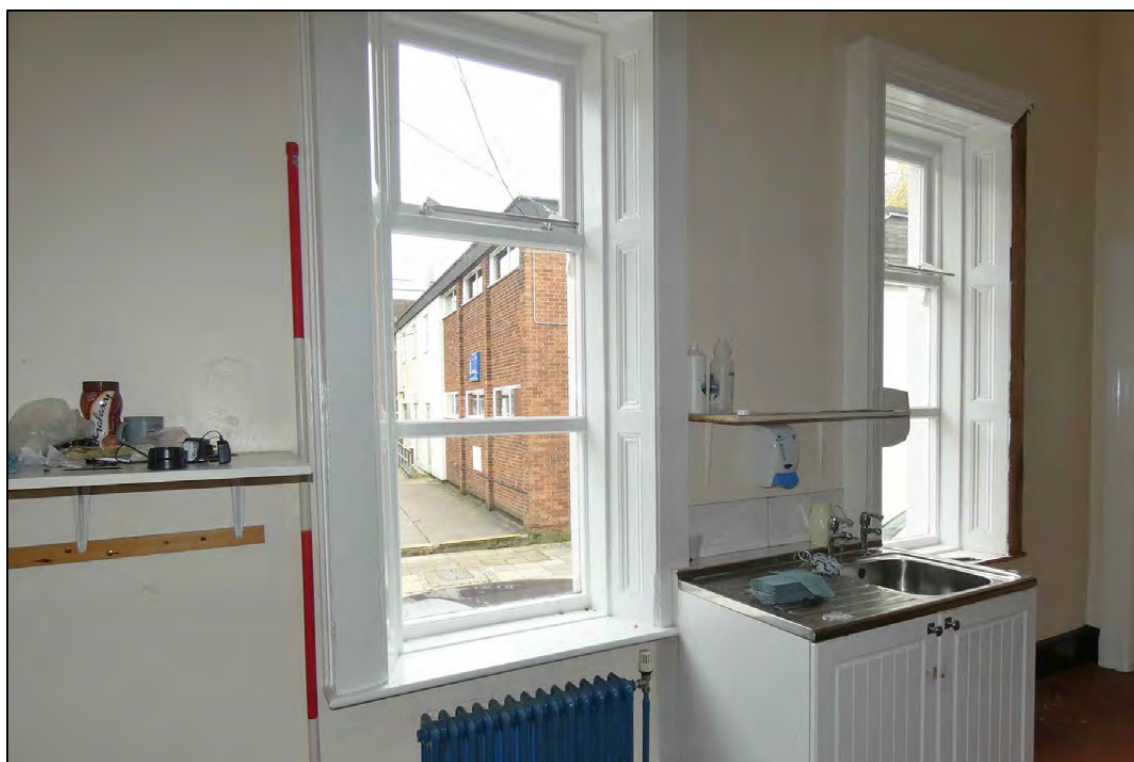
Appendix 2.79: General view of east wall G12 (DI21) (Scale 2m)
