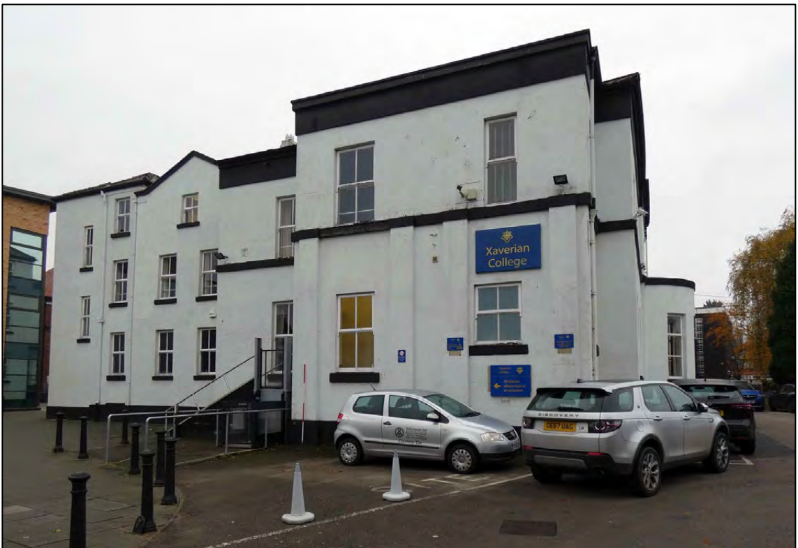
Appendix 2.4: General view of west elevation looking east (D2) (Scale 2m)
