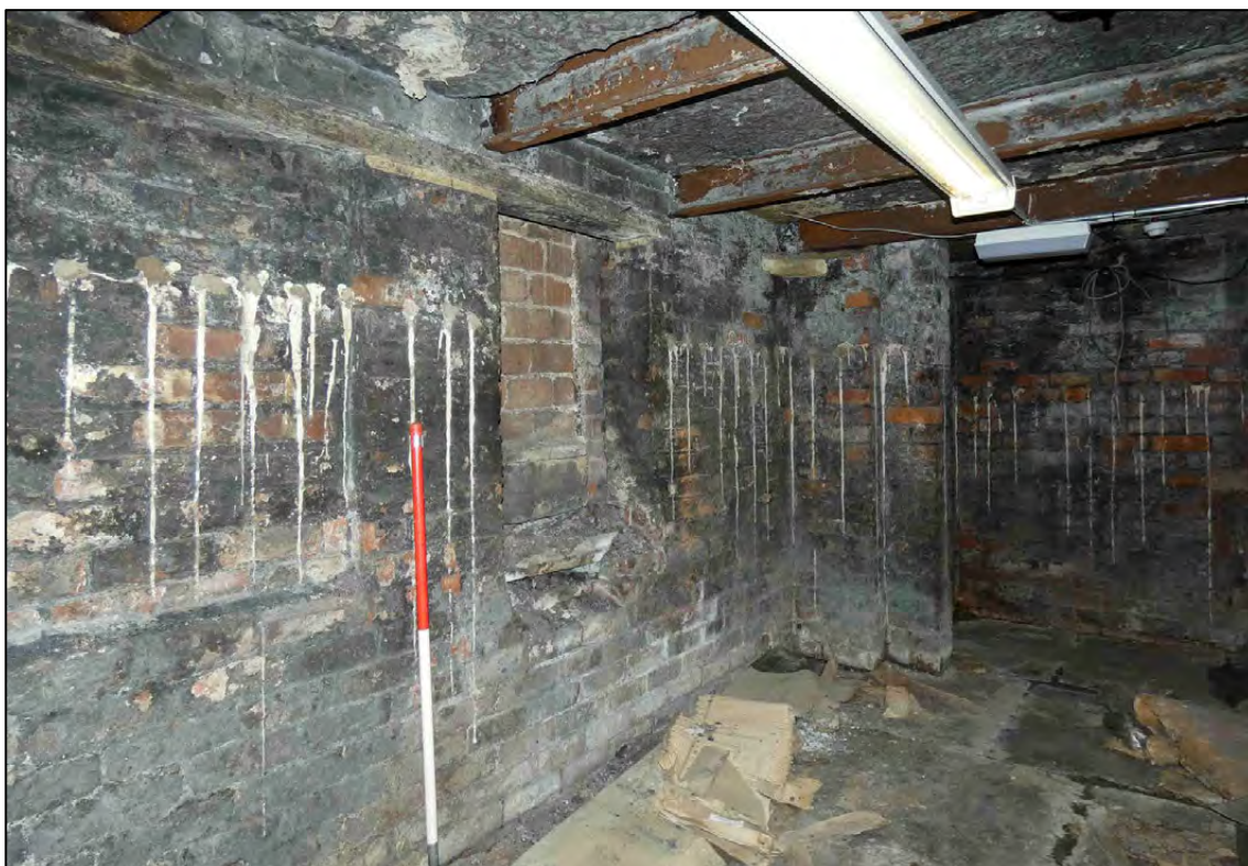
Appendix 2.33: General view of B13 looking east (D180) (Scale 1m)
