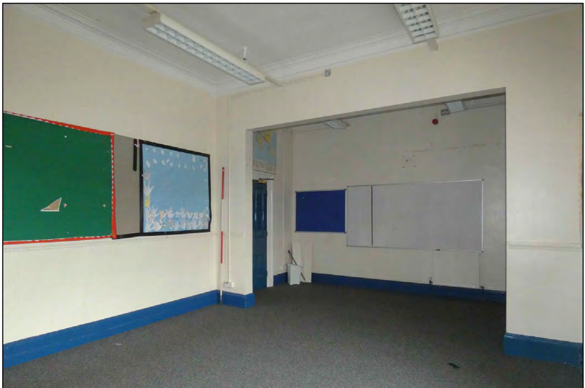
Appendix 2.117: General view of south and east walls F2 (D95) (Scale 2m)
