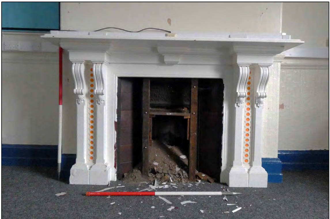
Appendix 2.95: Detail of fireplace in north wall F7 (D54) (Scale 1m)
