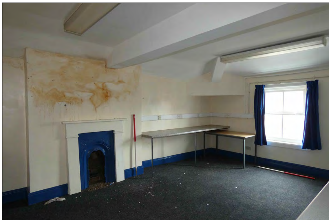
Appendix 2.140: General view of north and east walls S6 (D20) (Scale 1m)
