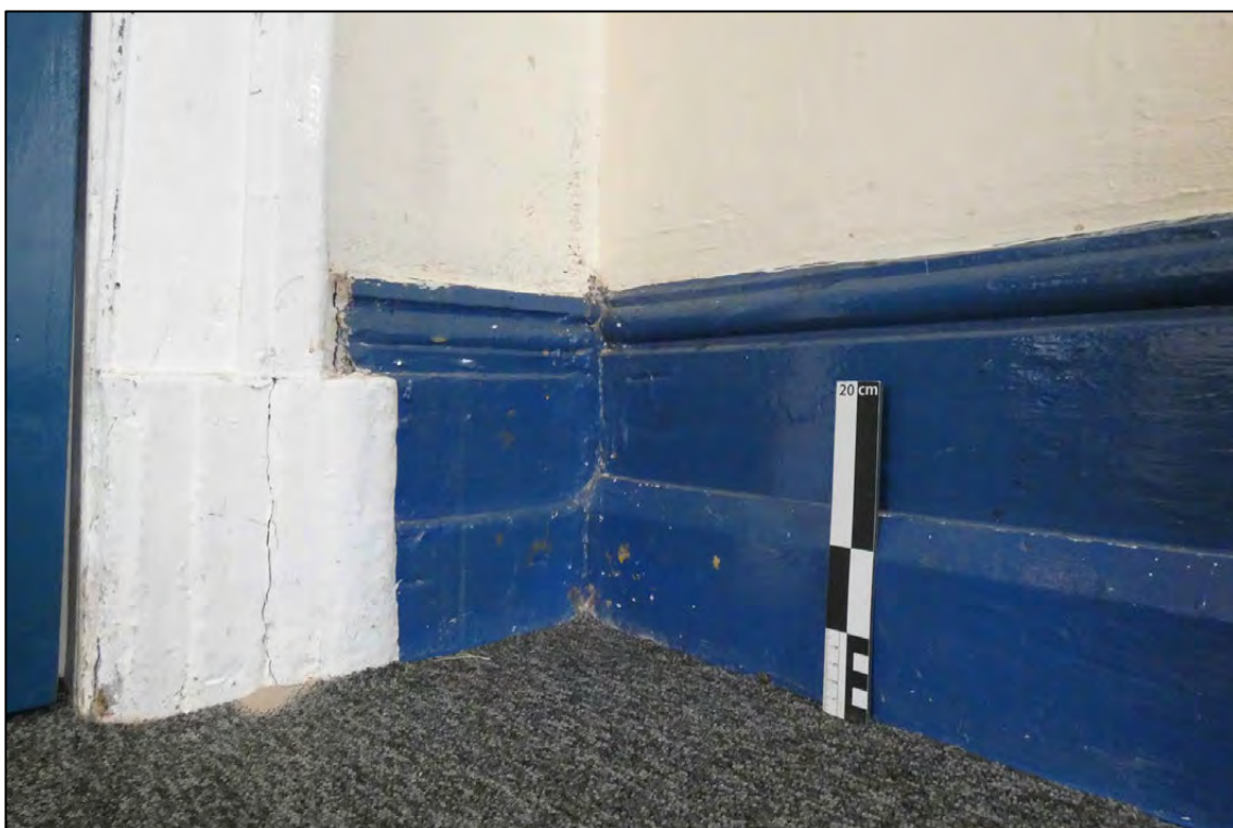
Appendix 2.109: Detail of skirting board in north west corner F4 (D60) (Scale 20cm)
