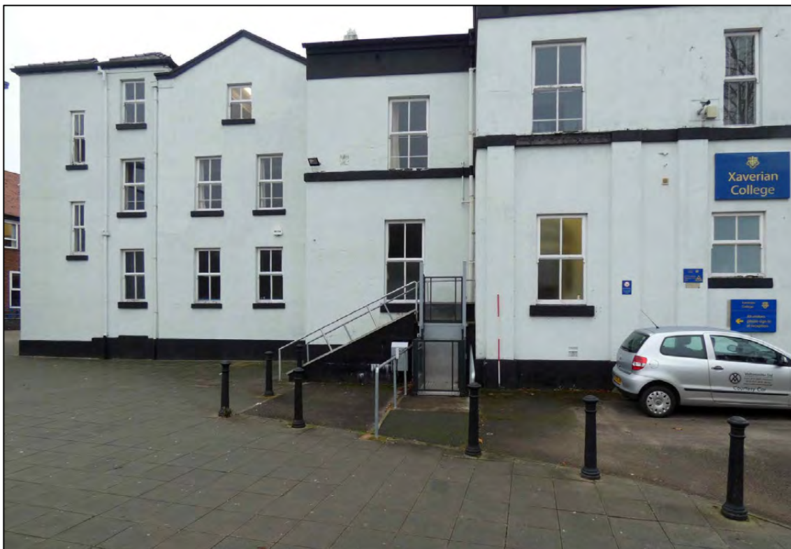
Appendix 2.13: General view of west elevation looking SE (DI5) (Scale 2m)
