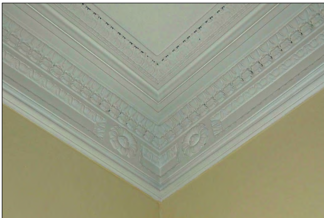
Appendix 2.68: Detail of coving above fireplace G11 (DI39)
