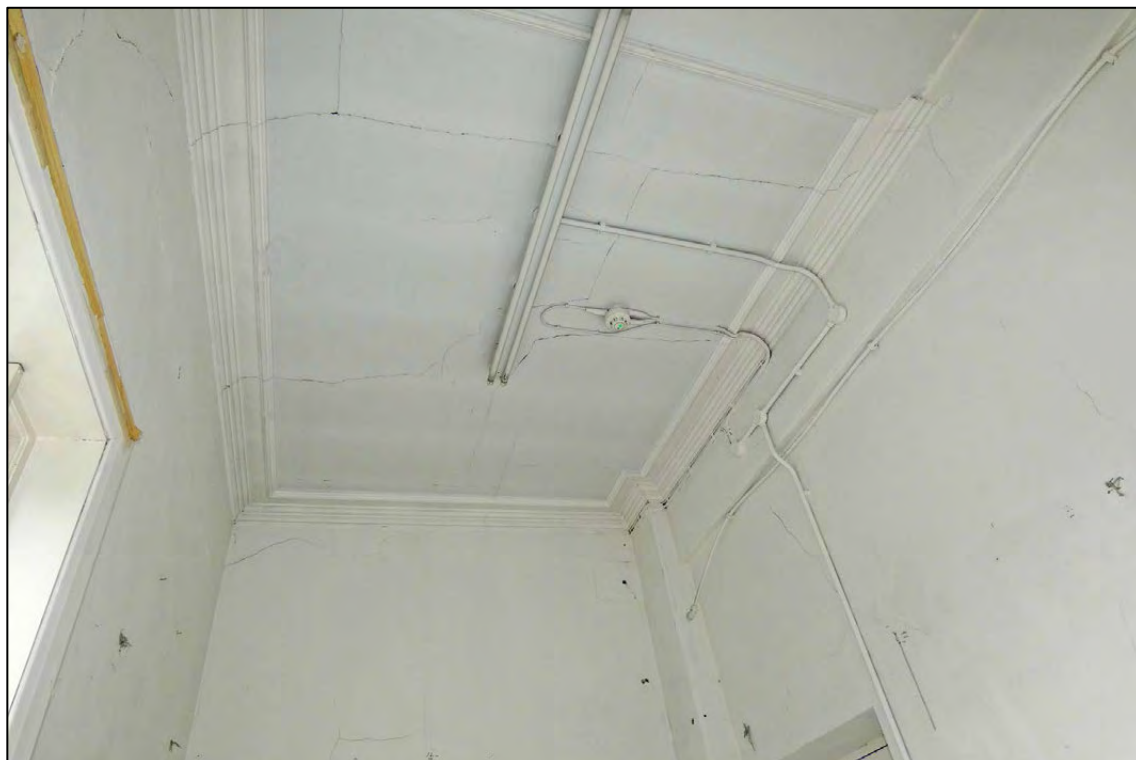
Appendix 2.129: General view of ceiling F5 (D91)
