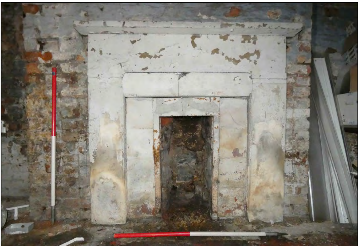
Appendix 2.16: Detail of fireplace B3 (DI60) (Scale 1m)
