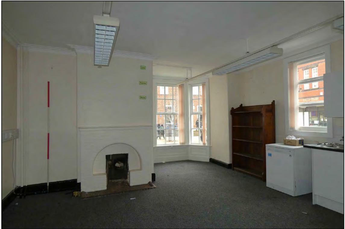
Appendix 2.72: General view of east and north walls of G14 (D109) (Scale 2m)
