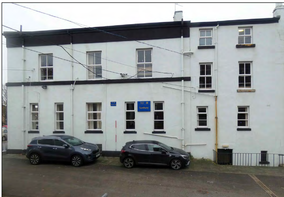
Appendix 2.9: General view of east elevation looking south (D10) (Scale 2m)
