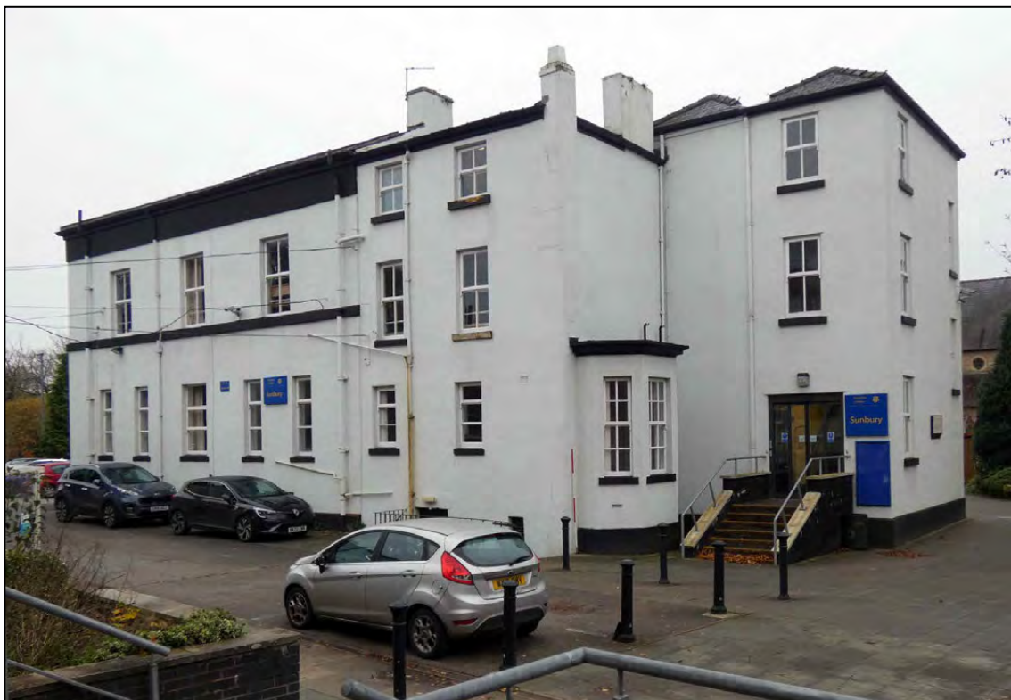
Appendix 2.10: General view of east and north elevation looking south (D12) (Scale 2m)
