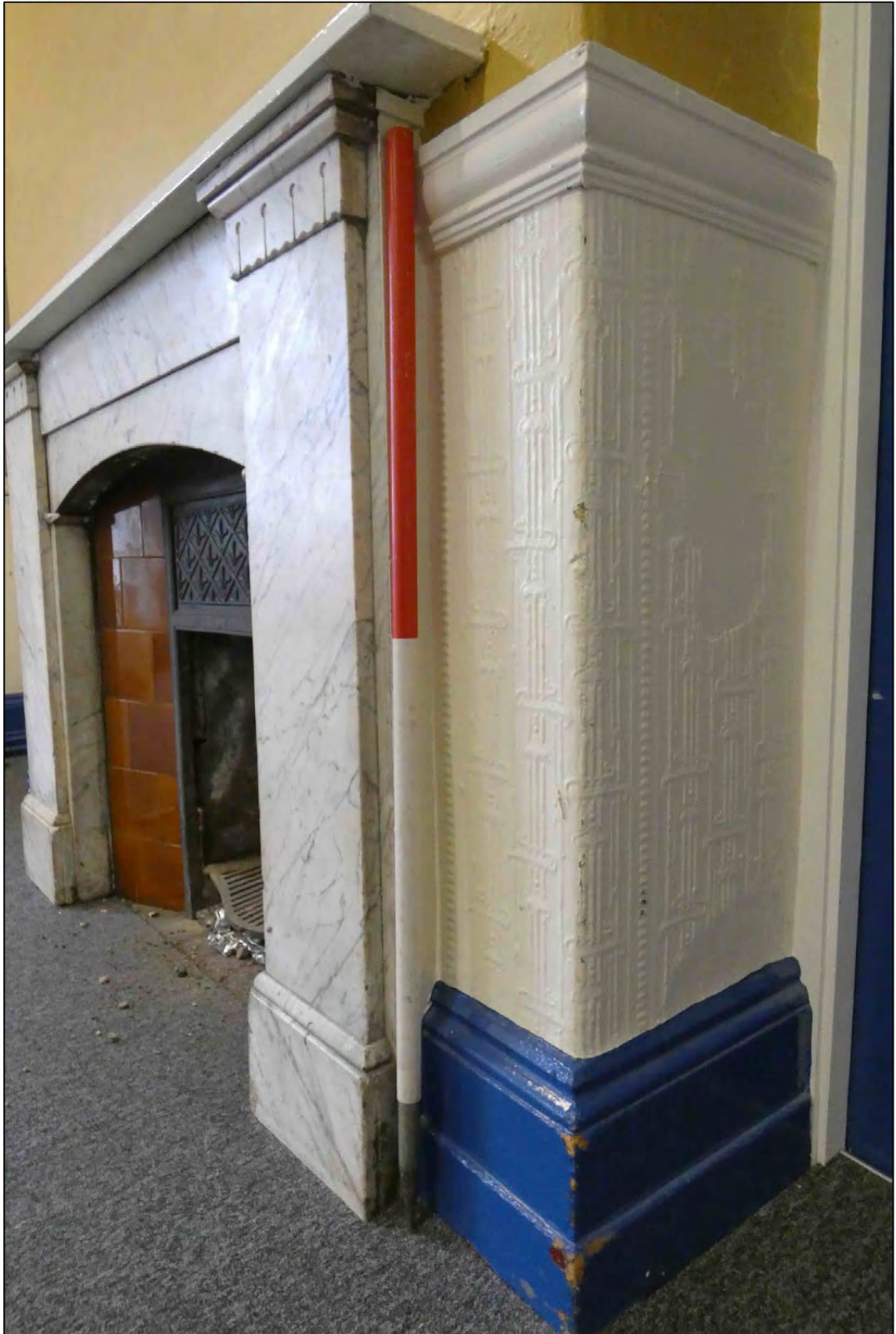
Appendix 2.113: Detail of fireplace in west wall F3 (D68) (Scale 1m)
