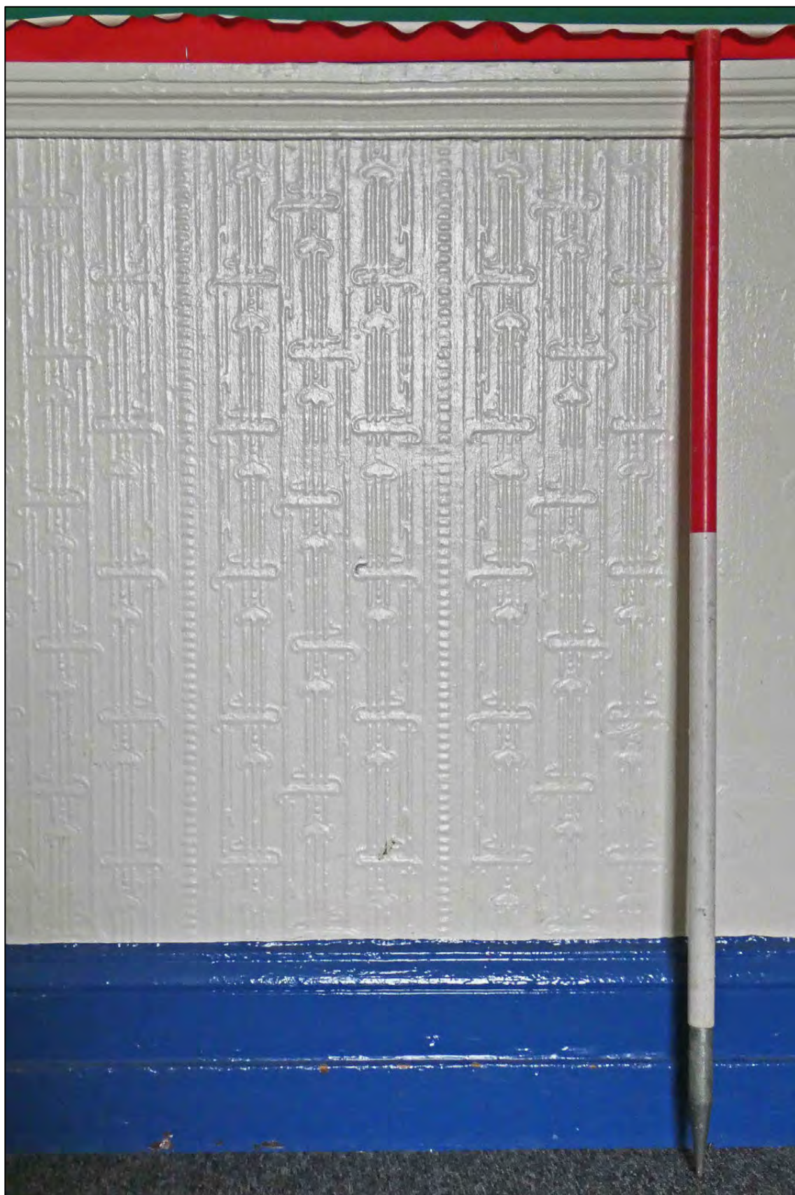
Appendix 2.120: Detail of skirting board and dado rail east wall F2 (D97) (Scale 1m)
