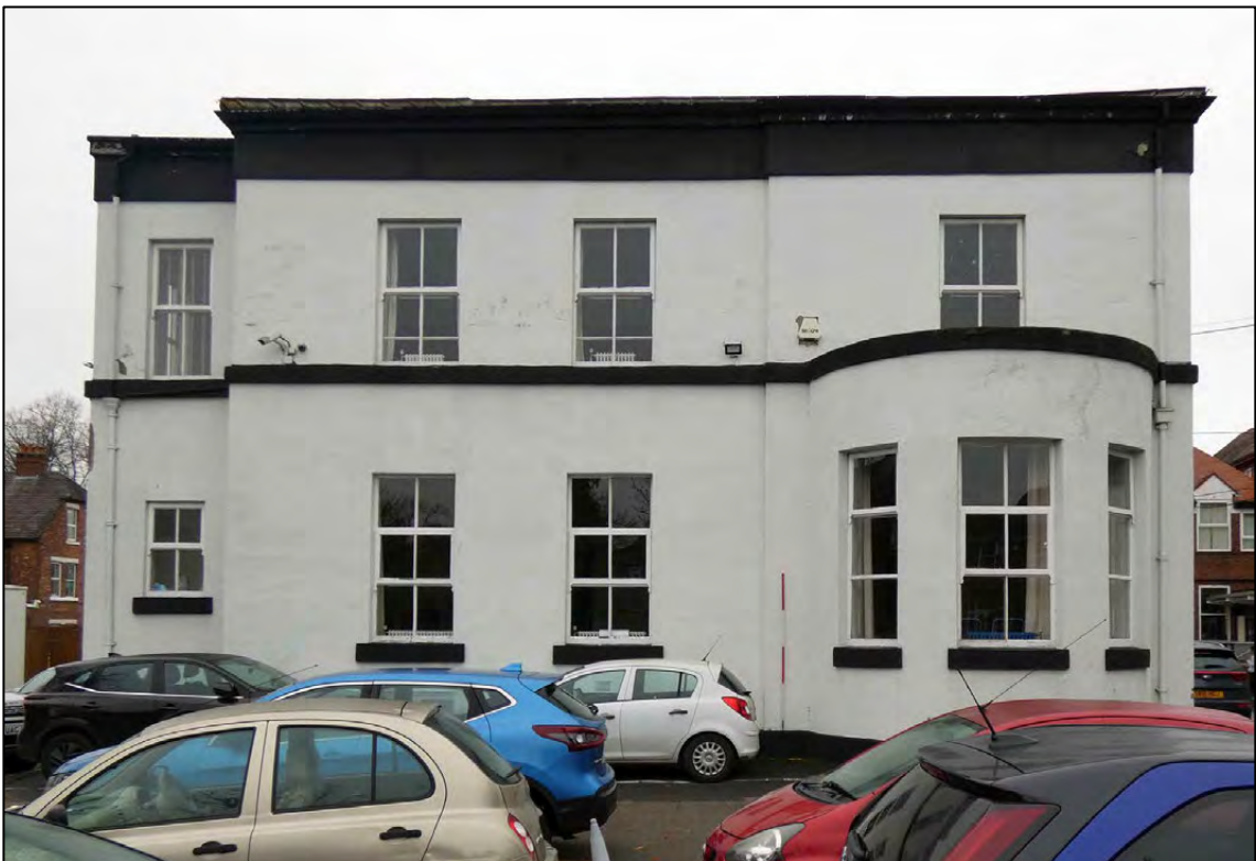
Appendix 2.6: General view of south elevation looking north (D8) (Scale 2m)
