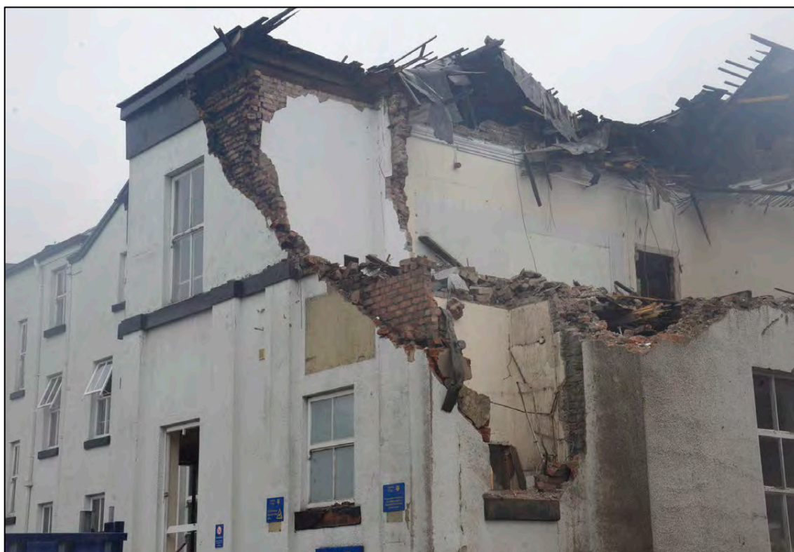
Appendix 2.14: General view of porch during demolition showing straight joint scar and original corner of F6 looking N (DI91) (Scale N/A)
