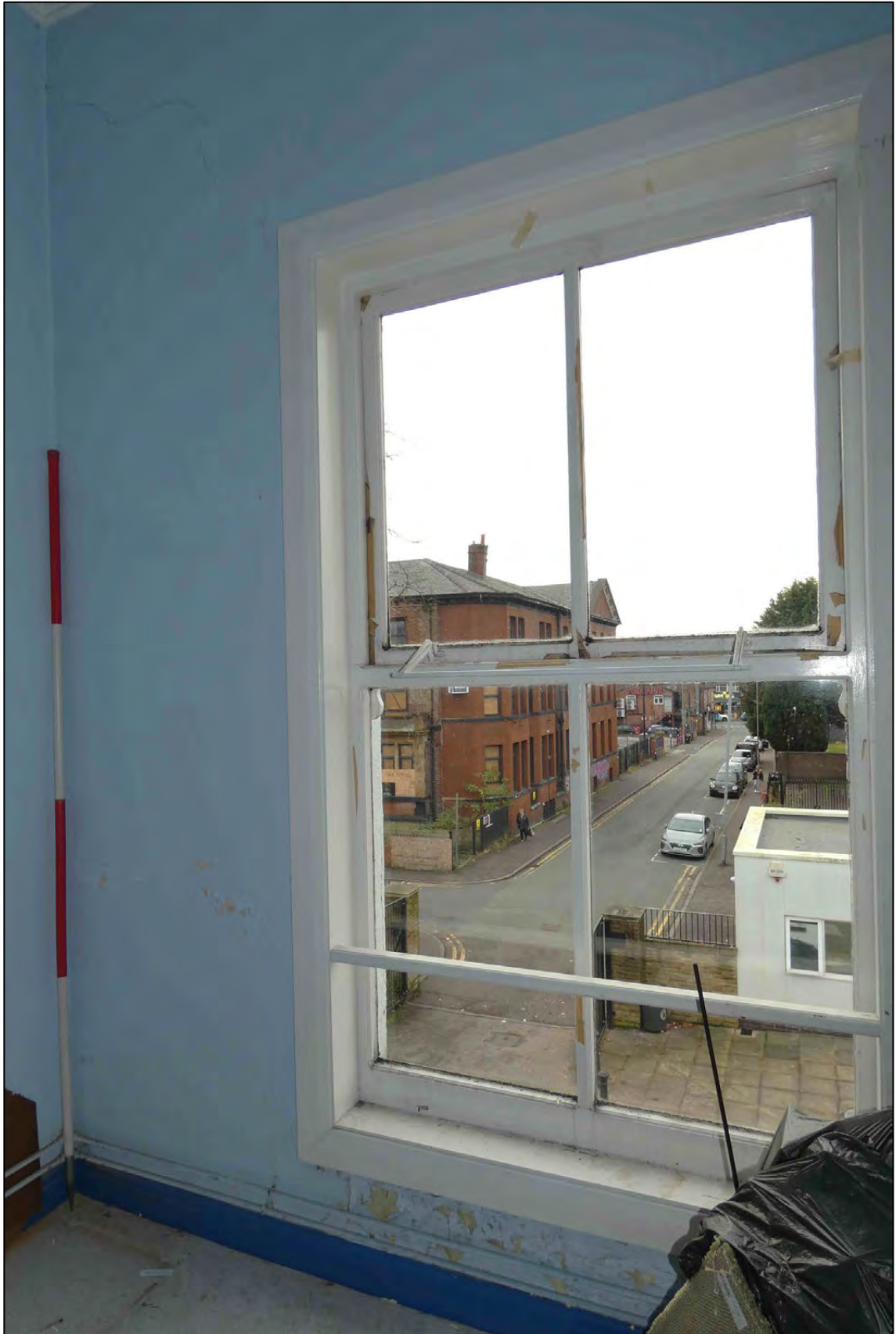
Appendix 2.131: Detail of window F6 (DI00) (Scale 2m)
