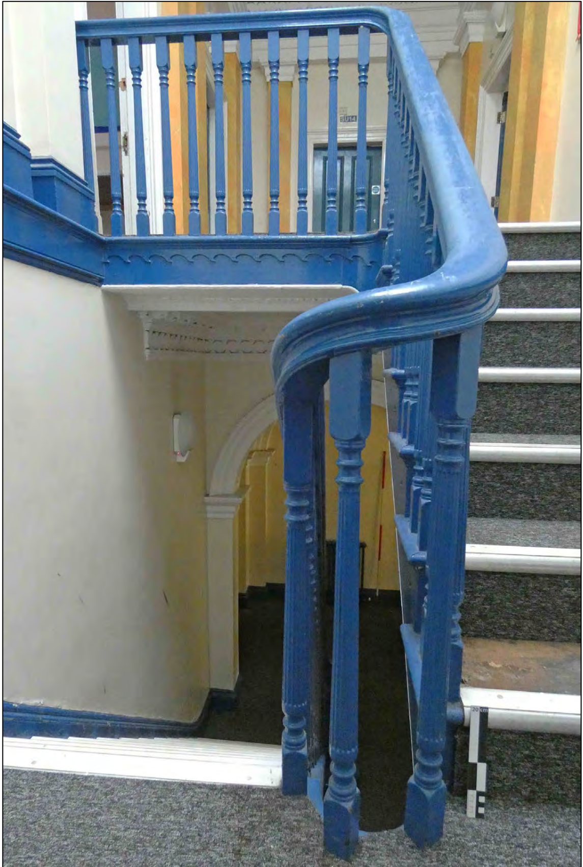
Appendix 2.86: General view of landing F8 (D41) (Scale 20cm/2m)
