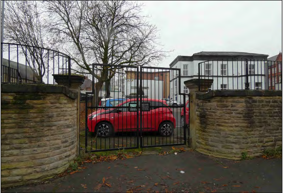
Appendix 2.1: Original front entrance to property looking N (D4)
