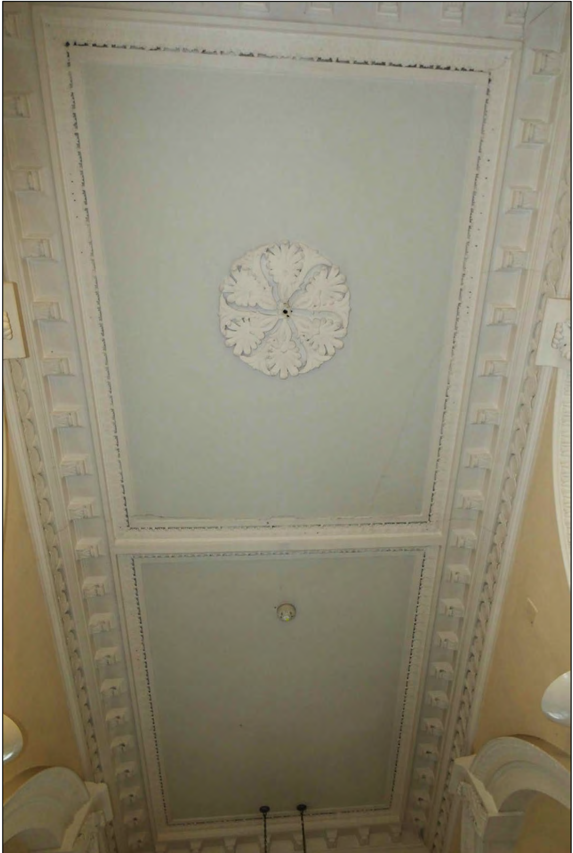
Appendix 2.39: Detail of ceiling G4 looking south-west (D128)
