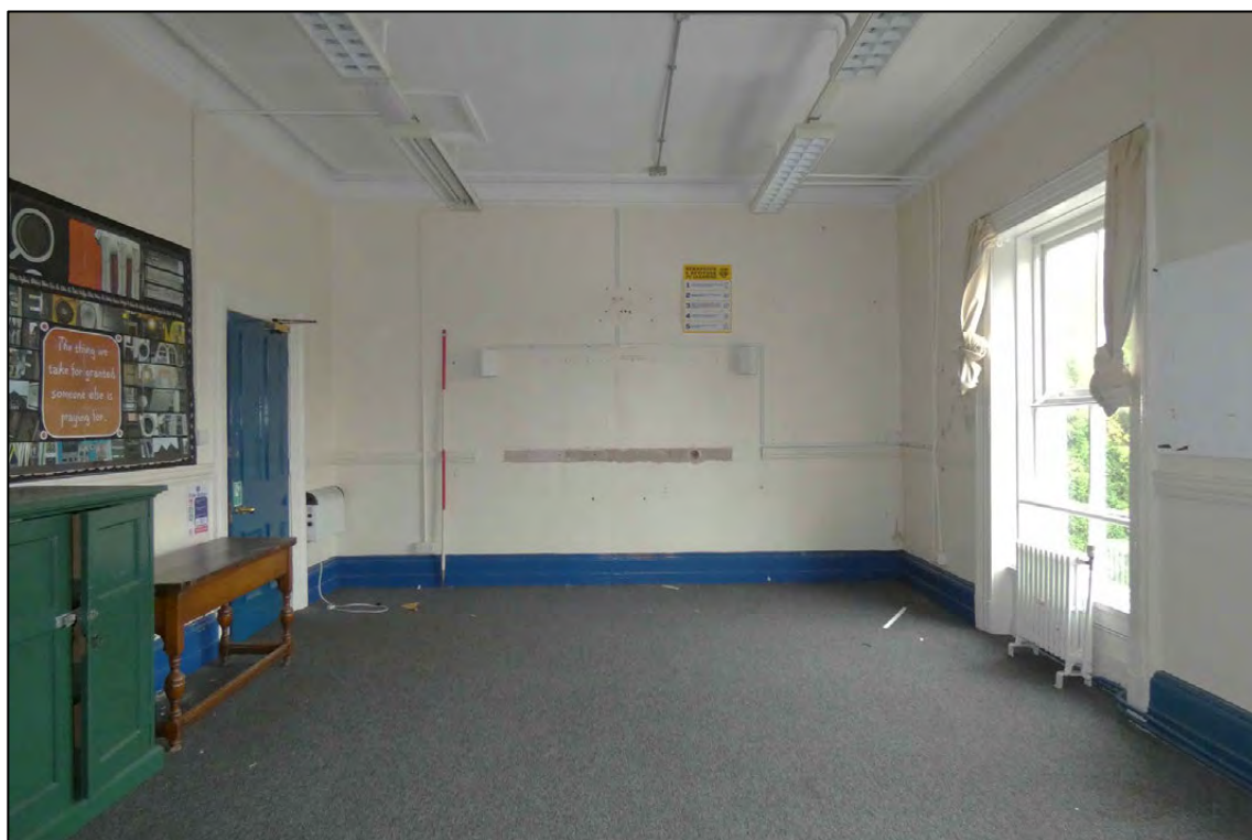
Appendix 2.III: General view looking east of F3 (D69) (Scale 2m)
