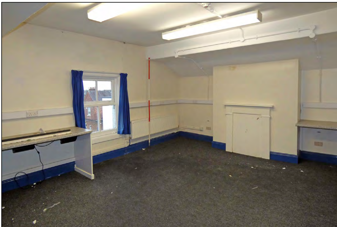
Appendix 2.142: General view of north and west walls S4 (D22) (Scale 2m)
