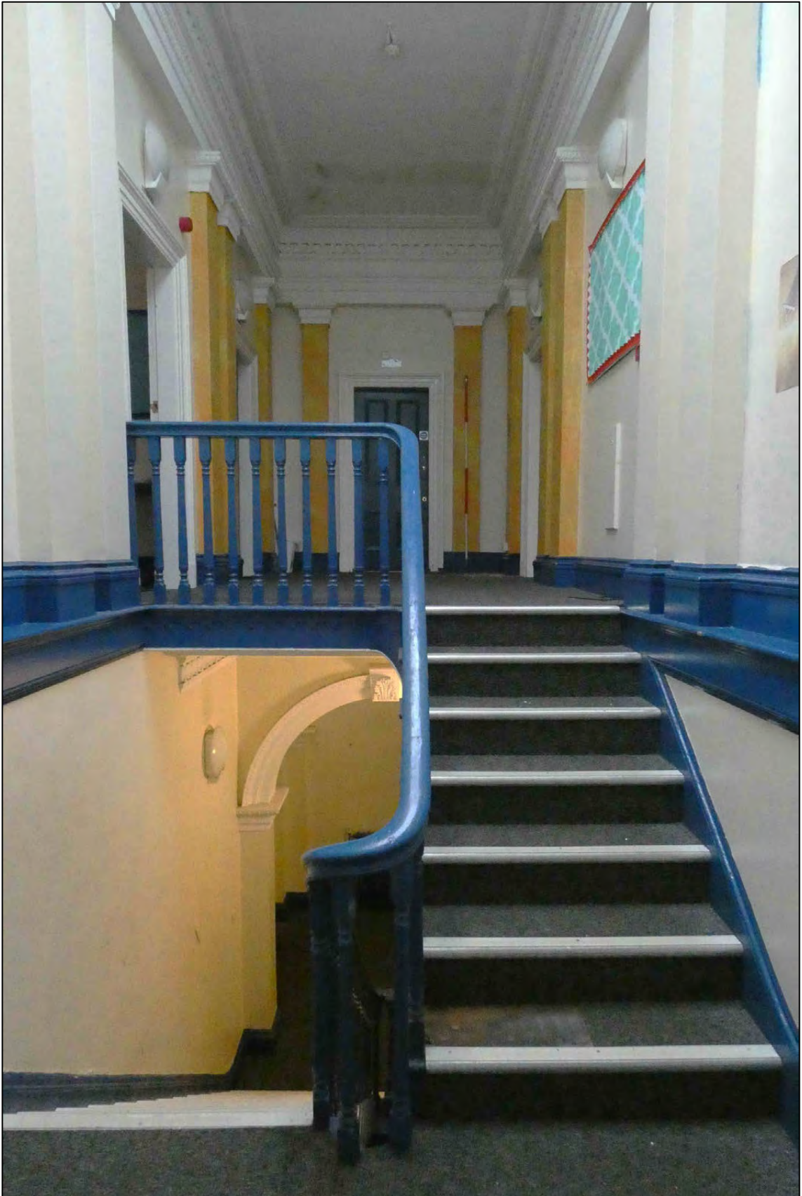
Appendix 2.85: General view of staircase F8 (D39) (Scale 2m)
