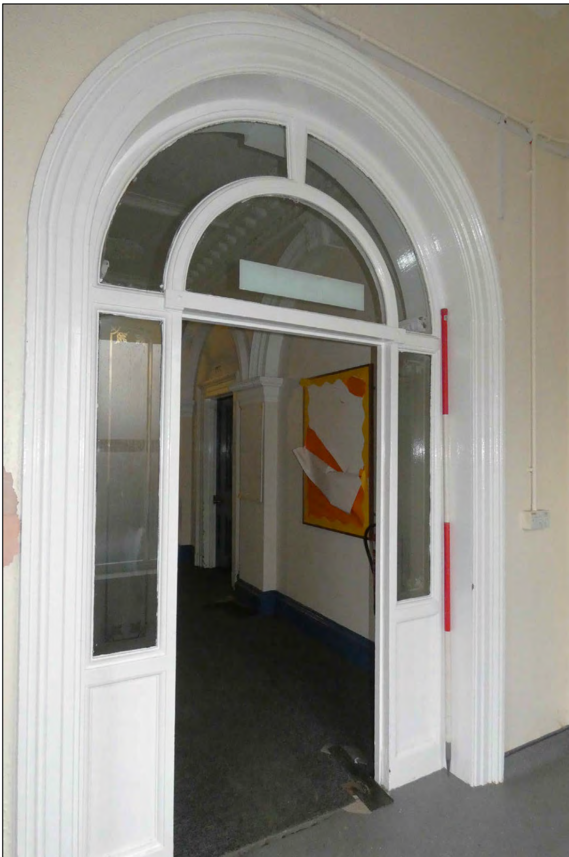
Appendix 2.34: General view of doorway G1 (D131) (Scale 2m)
