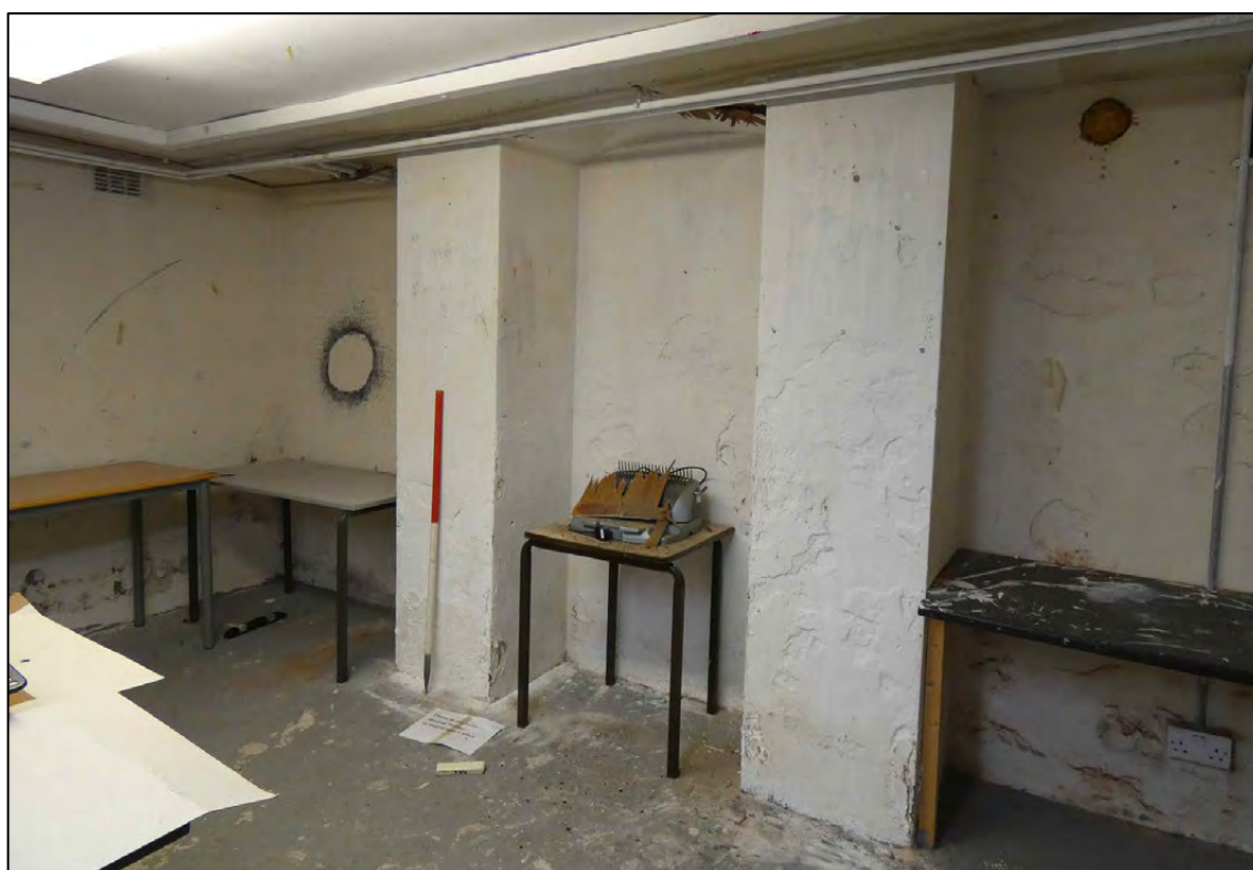
Appendix 2.24: Detail of removed fireplace B5 (DI67) (Scale 1m)
