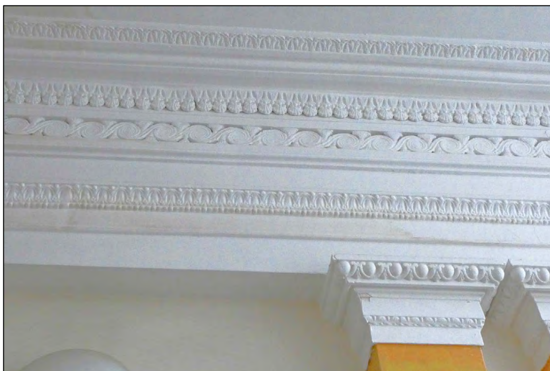
Appendix 2.91: Detail of deep coving F1 on west wall(D50)
