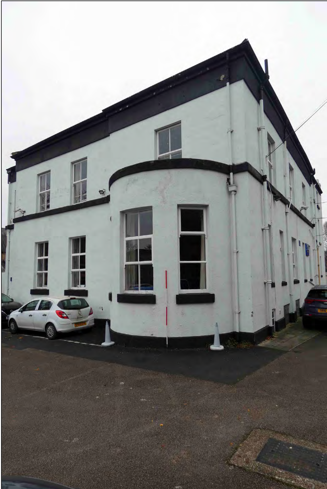
Appendix 2.7: General view of bay window on south elevation looking NW (D7) (Scale 2m)
