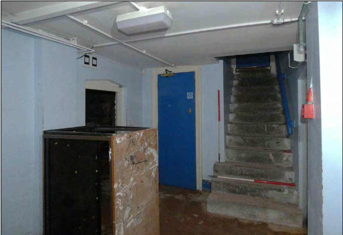
Appendix 2.17: General view of staircase B1 (DI63) (Scale 1m)
