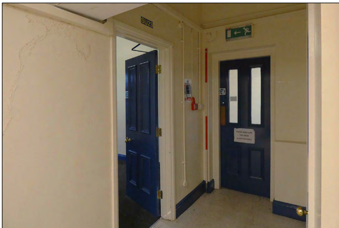
Appendix 2.144: Detail looking north in corridor S5 towards S1 and open doorway to S3 (D25) (Scale 2m)
