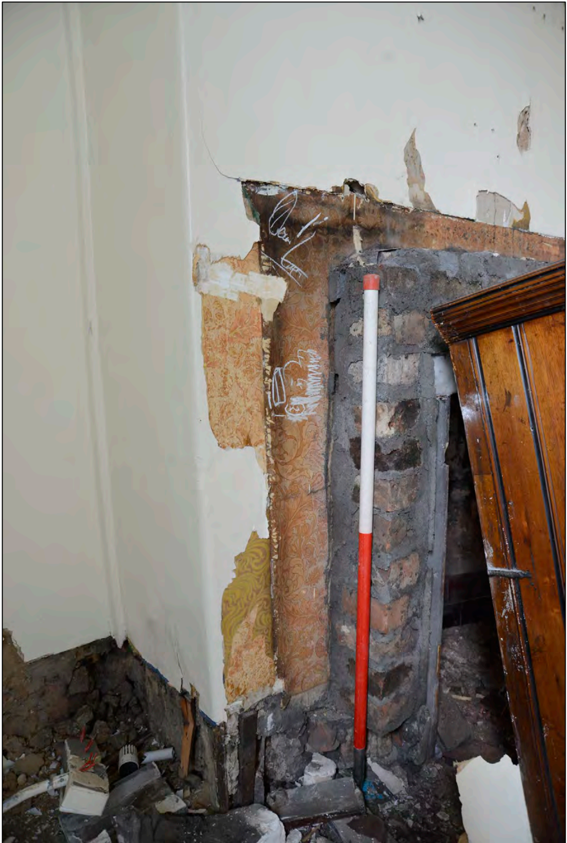
Appendix 2.69: G11 General view of wallpaper revealed behind chimneypiece during SWB looking N (Scale 1m)
