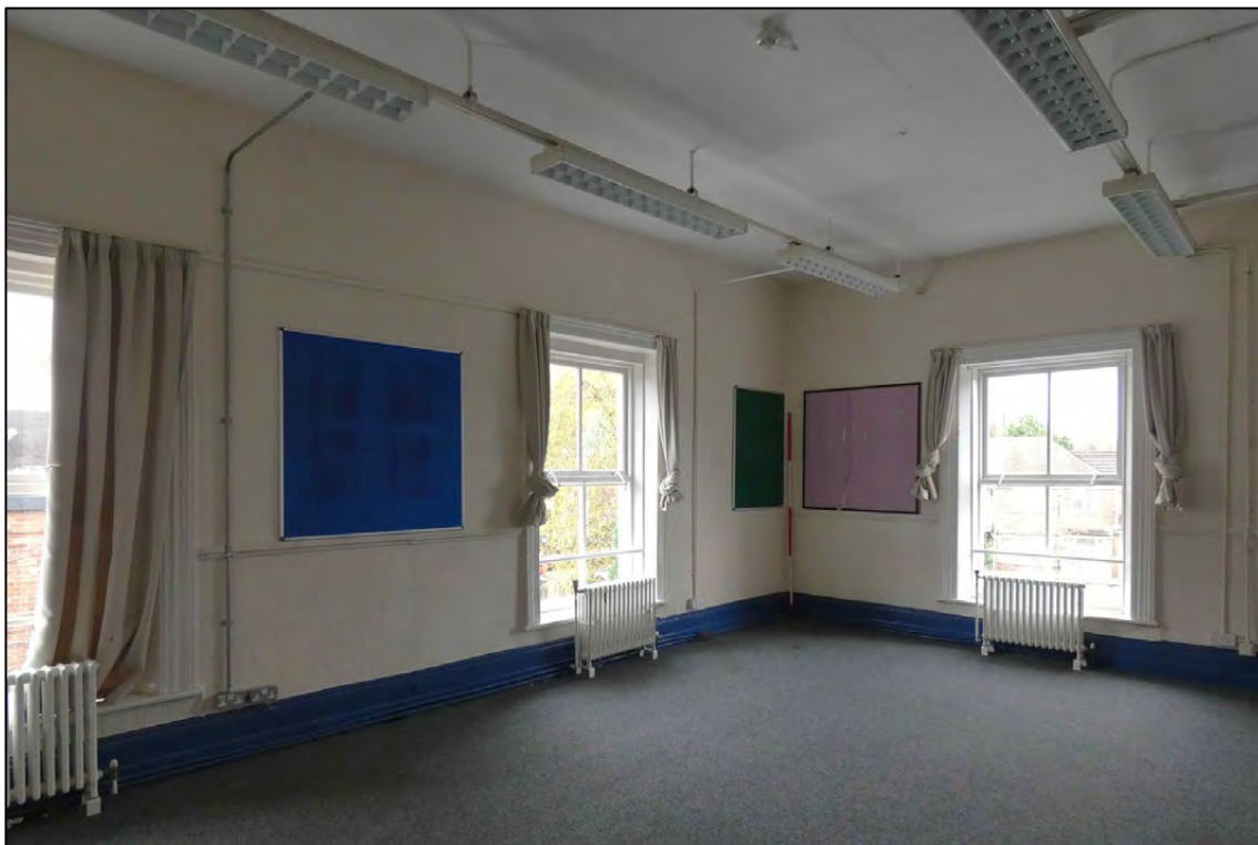
Appendix 2.100: General view of east and south walls F4 (D57) (Scale 2m)
