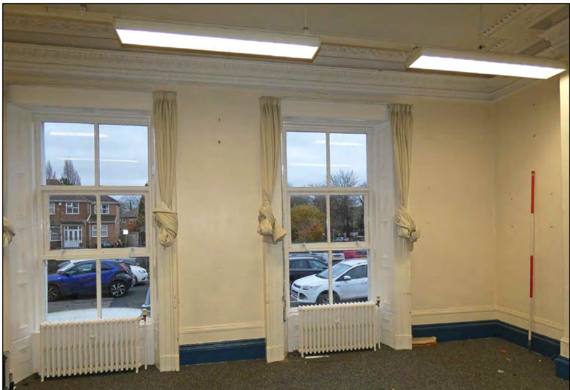
Appendix 2.58: General view of windows in south wall of G9 (D141) (Scale 2m)
