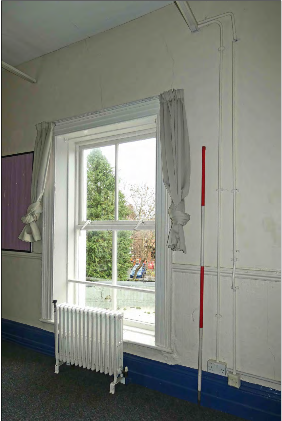
Appendix 2.102: Detail of window in south wall F4 (D59) (Scale 2m)
