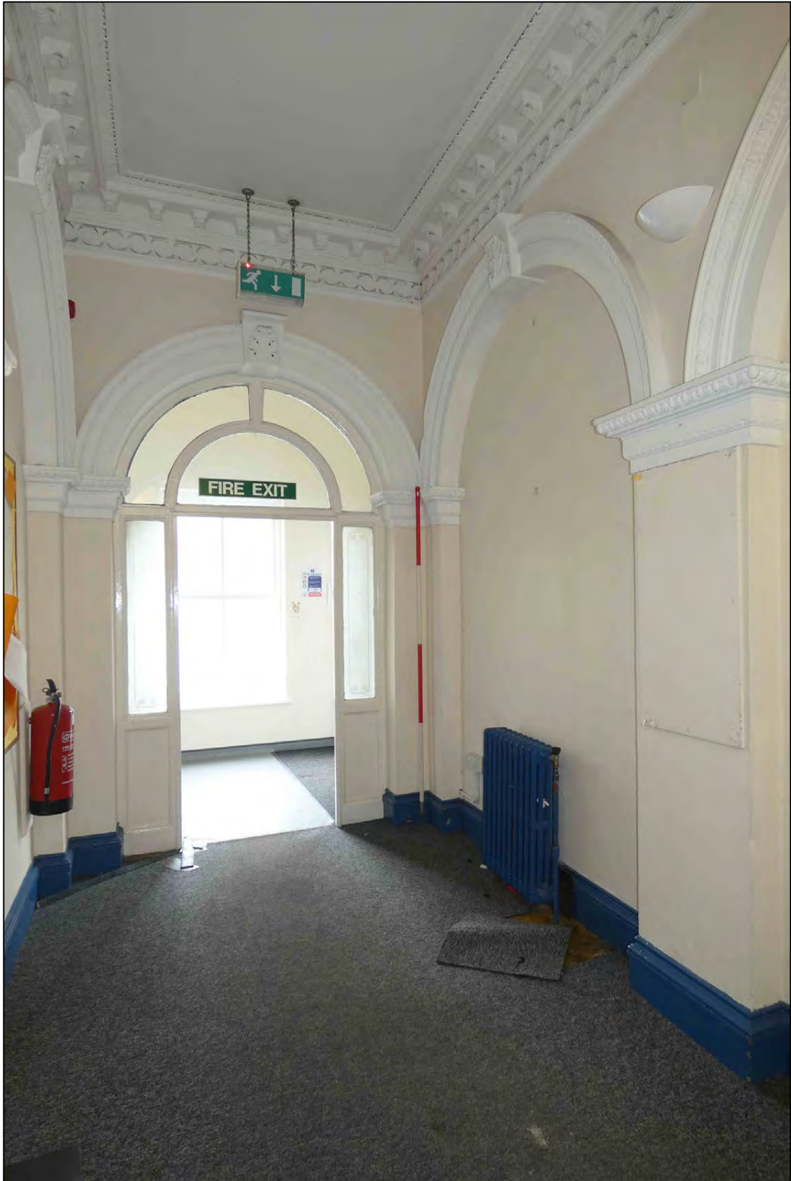
Appendix 2.36: General view G4 looking west (D127) (Scale 2m)
