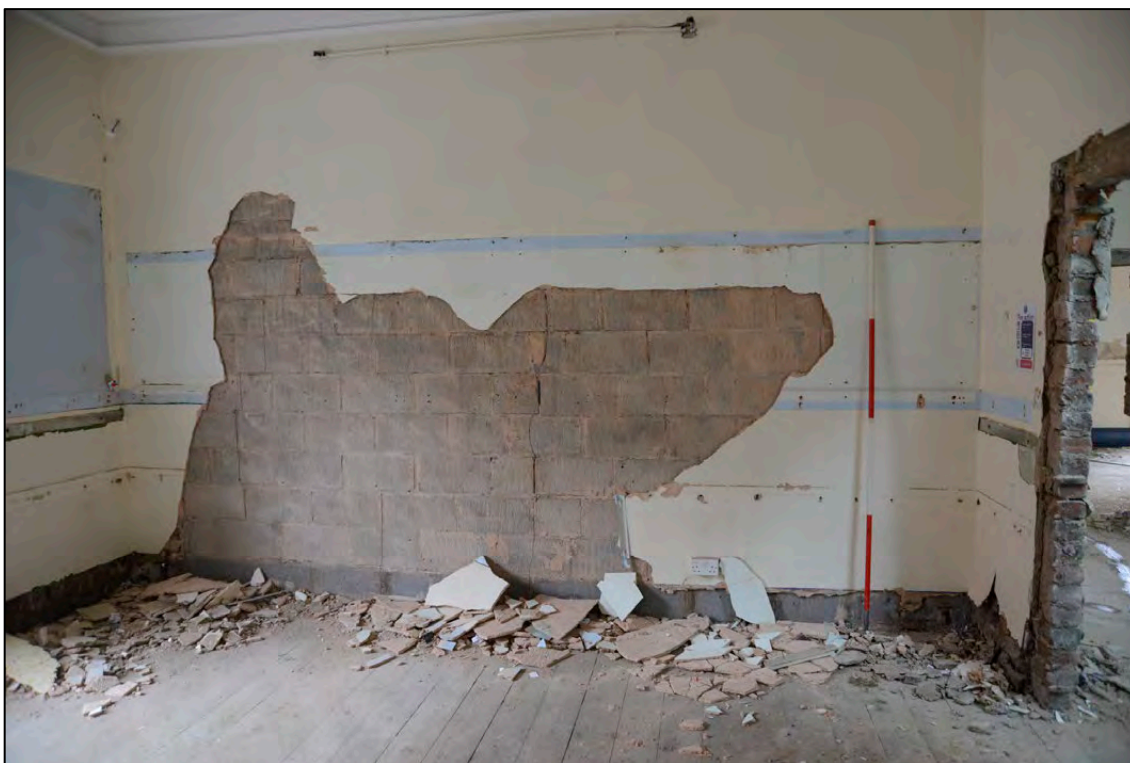
Appendix 2.98: F7 General view of blockwork partition in south wall during SWB looking SE (D182) (Scale 2m)
