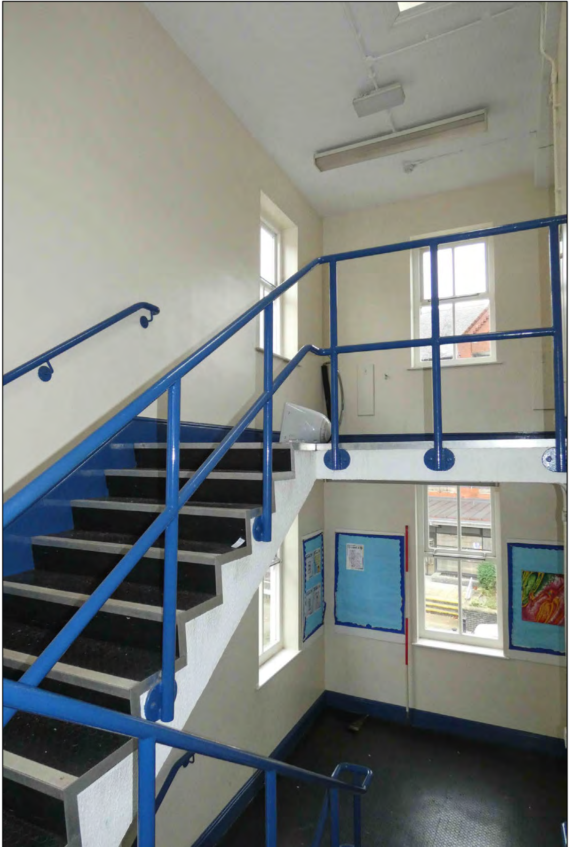
Appendix 2.146: General view of stairwell S1, looking north-east (D28) (Scale 2m)
