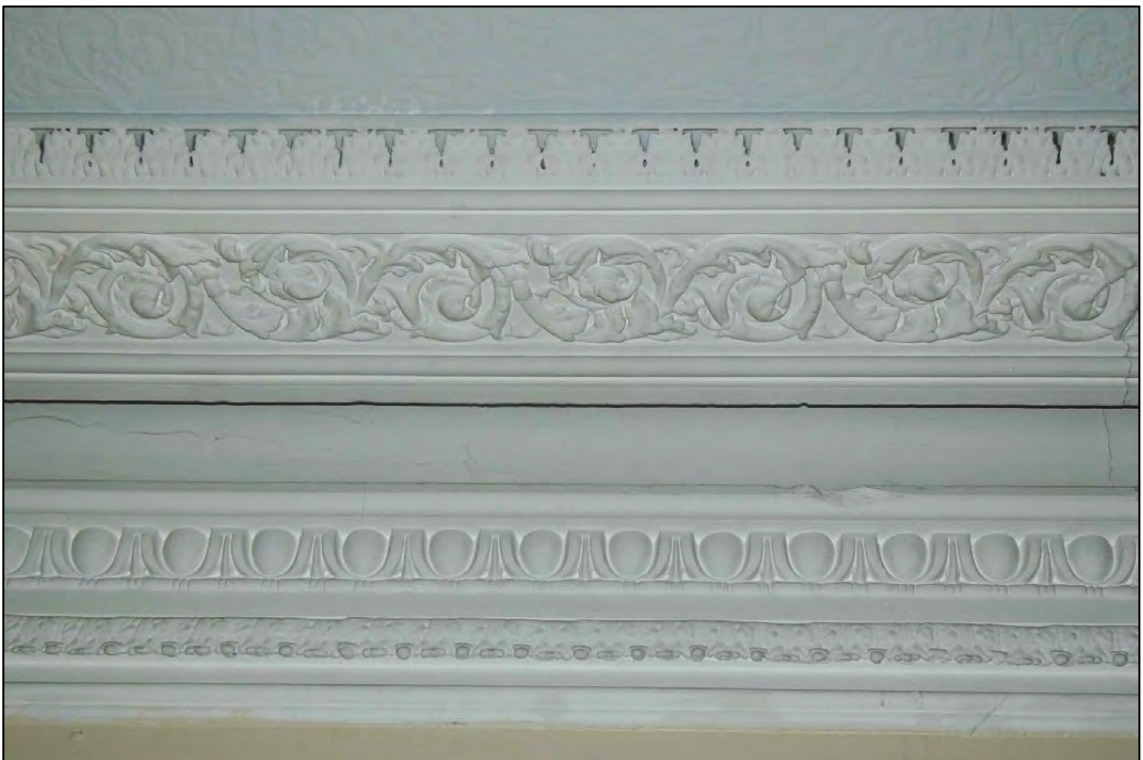
Appendix 2.63: Detail of coving on north wall G9 (DI46)
