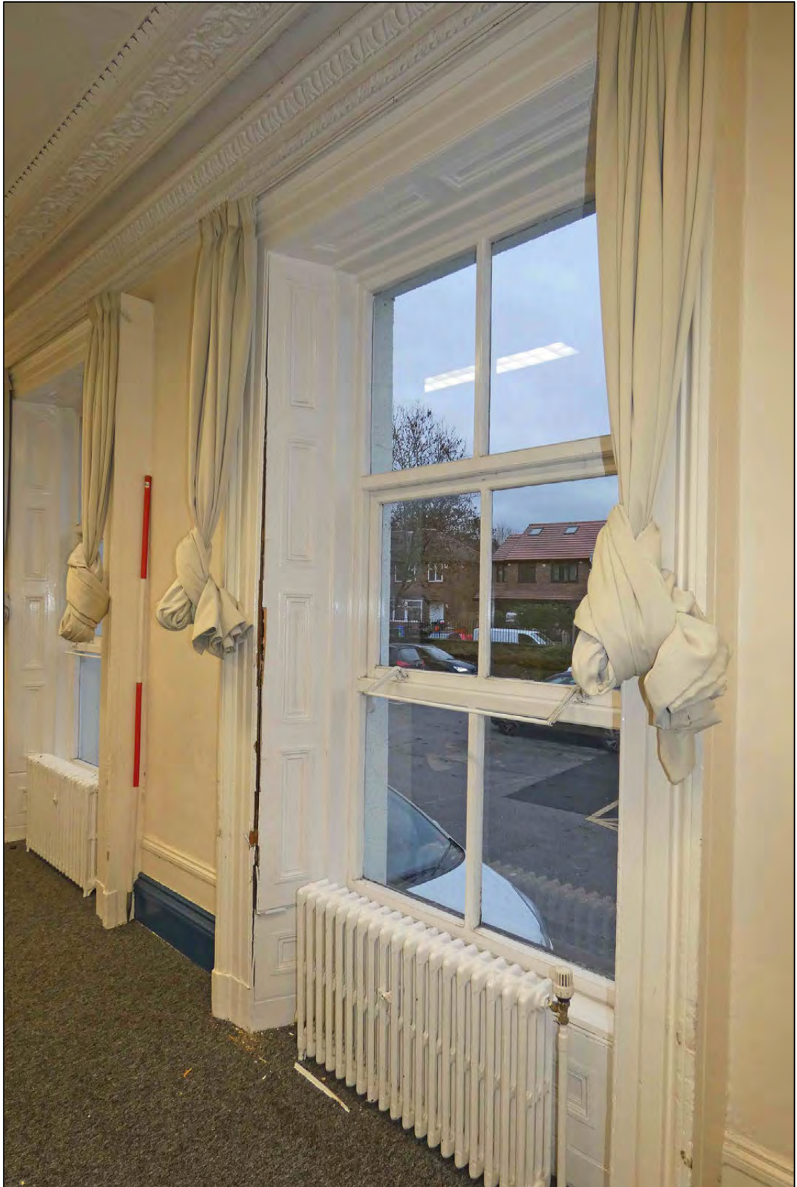
Appendix 2.59: Detail of windows G9 (DI43) (Scale 2m)
