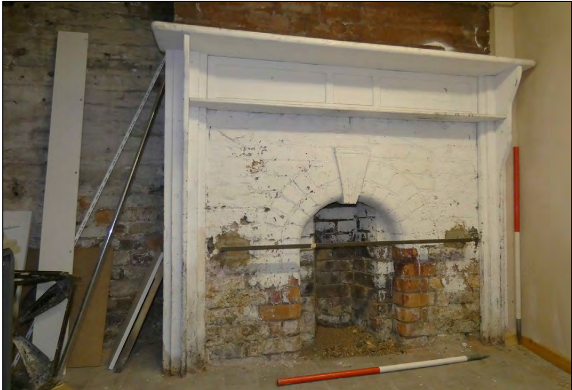
Appendix 2.21: Detail of fireplace B7 (DI65) (Scale 1m)
