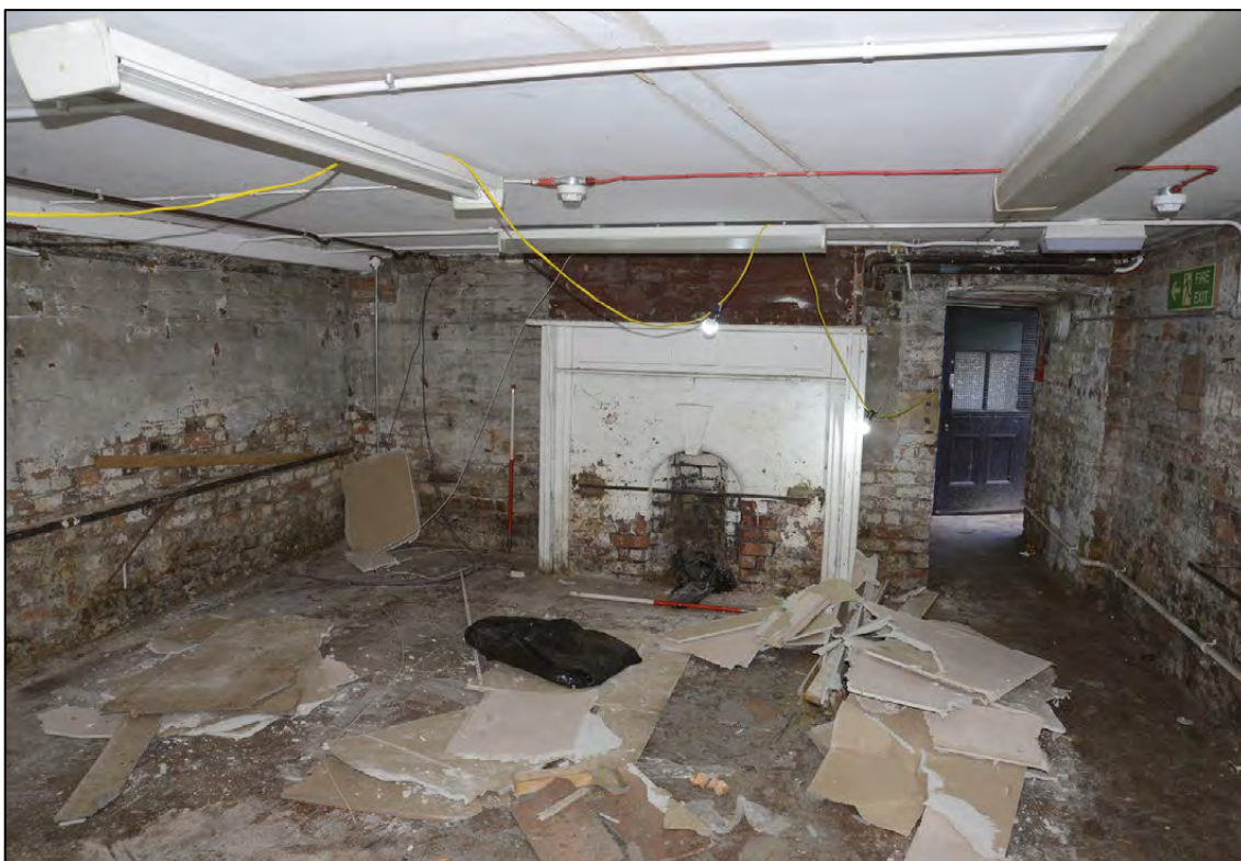
Appendix 2.19: General view of B7, following removal of partition looking north (D164) (Scale 1m)
