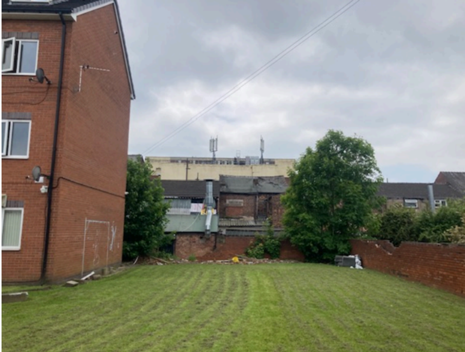
View of application site showing the gable of the existing building
