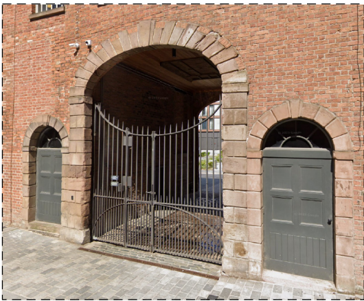
Examples of gates in similar contexts: top – Royal Mill, Ancoats, bottom – Murray's Mill, Ancoats
