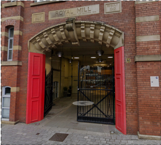
Original gates refinished and pinned back, ie. A retained but non-functioning heritage element.
