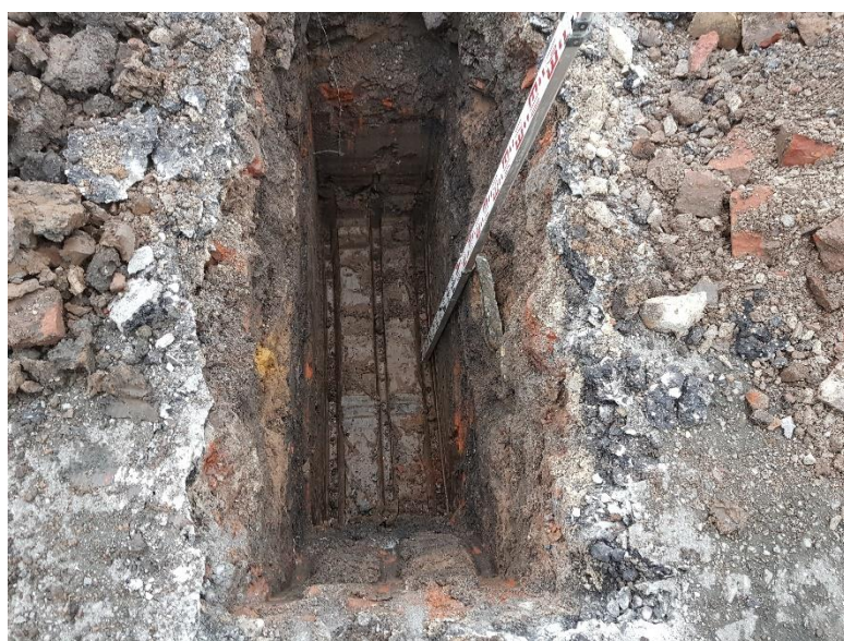
TP101: Internal view of excavation.
