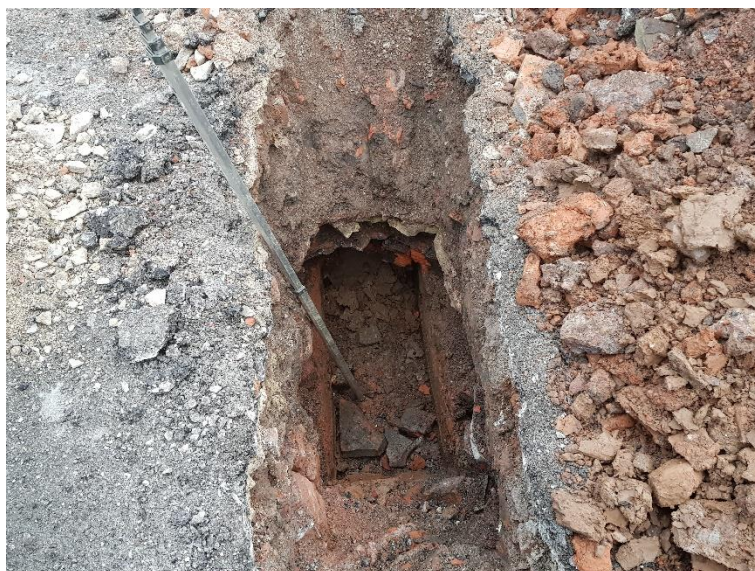
TP104: Internal view of excavation.
