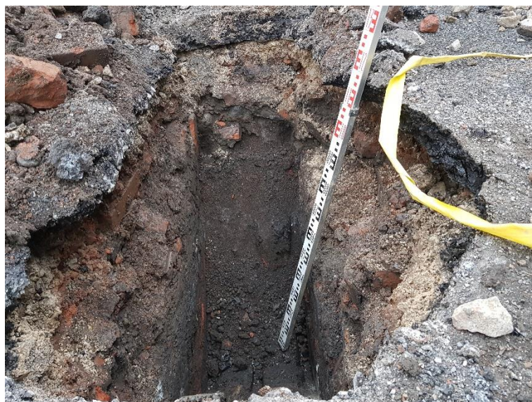
TP103: Internal view of excavation.
