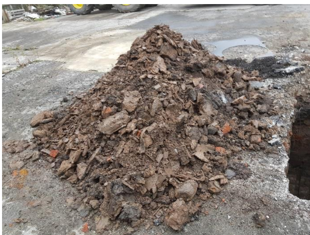
TP101: Excavation spoil
