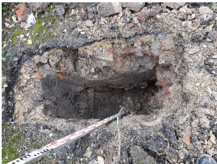
TP102: Internal view of excavation.
