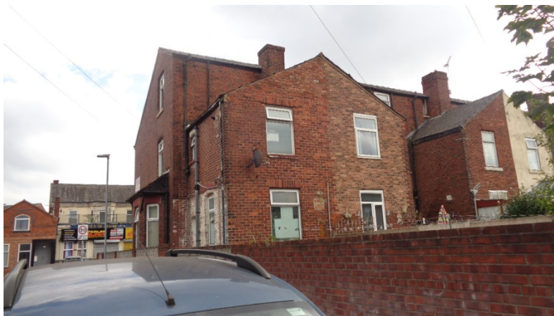
Rear Elevation of Application Property.
