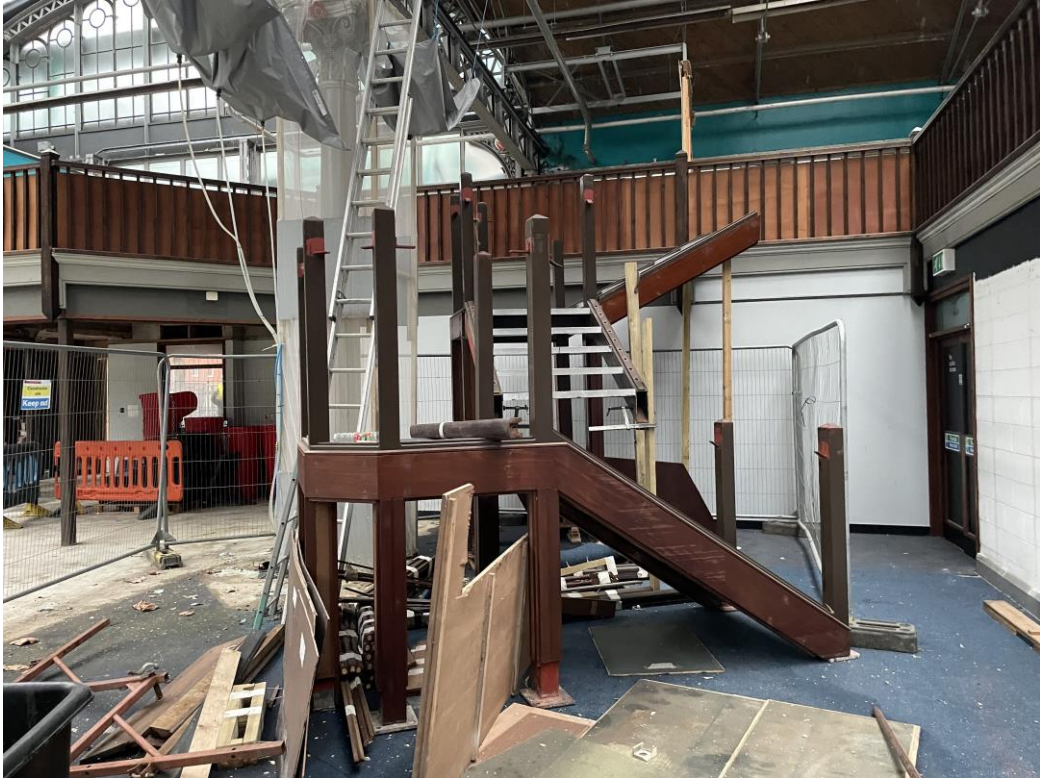
Figure 117: A view of the 1980s balcony staircase that was located to the centre of the east elevation showing it here recently moved into the south-east corner.
