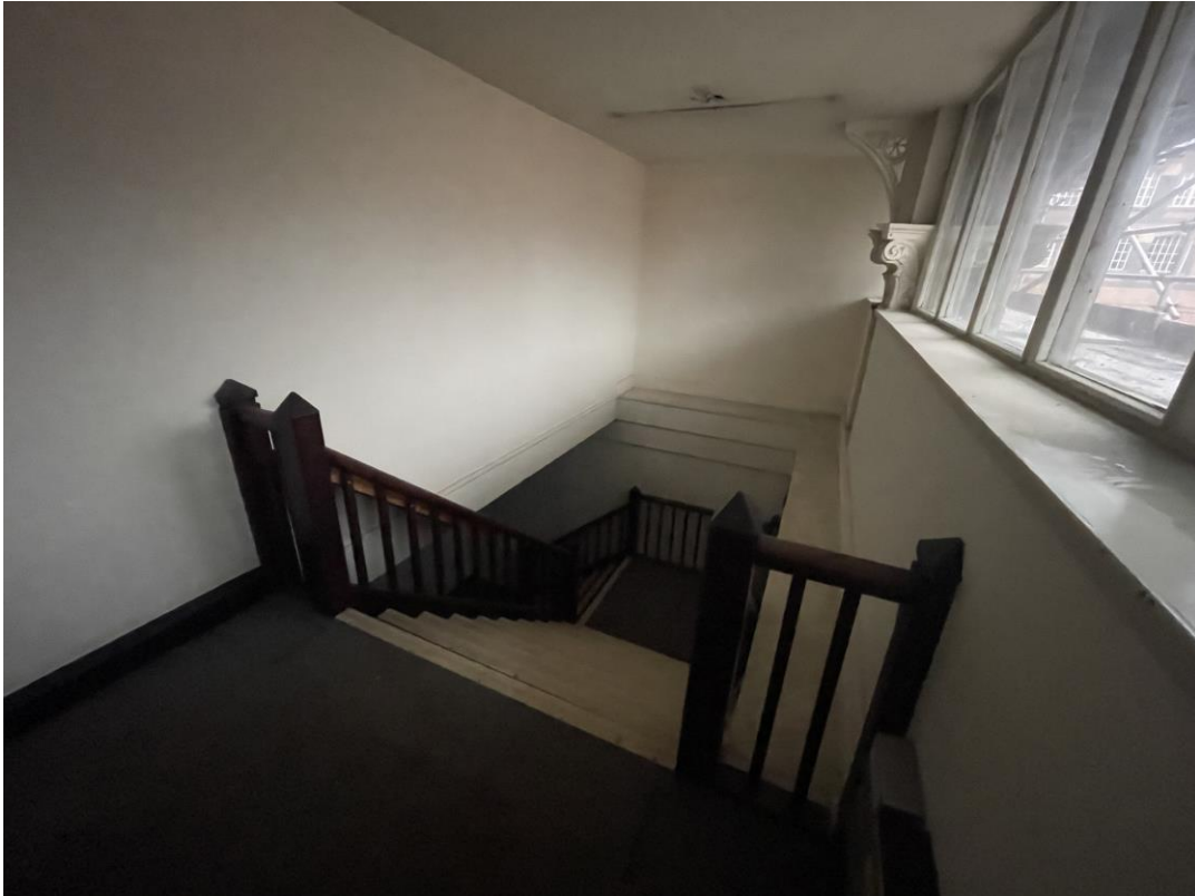
Figure 153: Looking into the 1980s north-west corner staircase to the ground floor.
