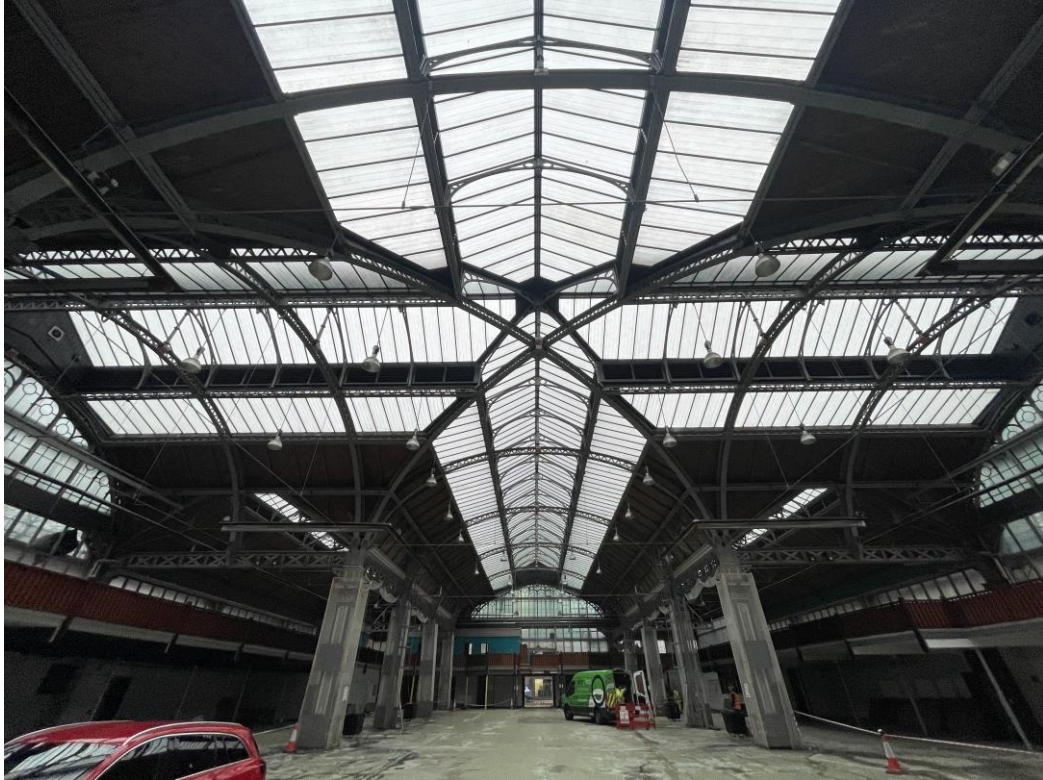
Figure 122: Looking up at the roof.
