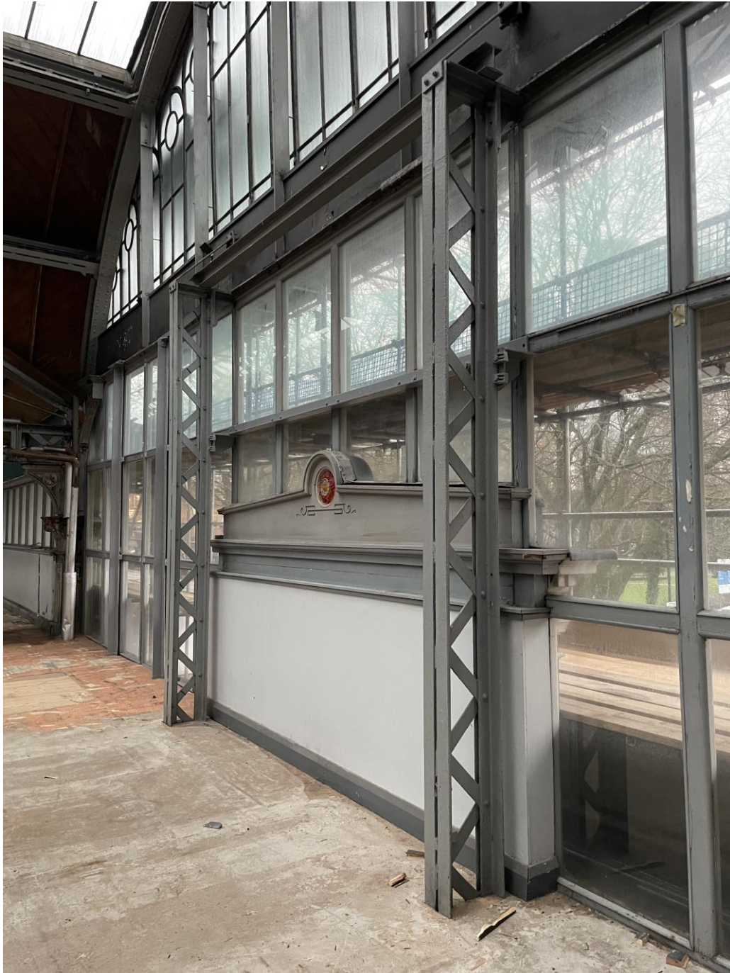
Figure 141: A closer view of the original lattice iron gate supports.
