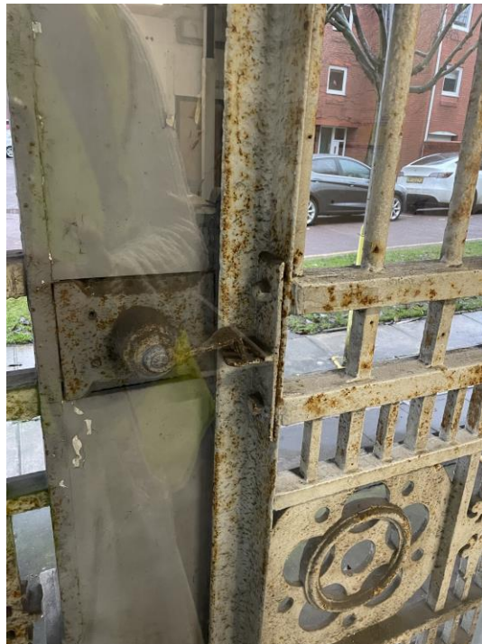
Figure 91 & 92: View of the rear of the original sliding gate as seen from the interior of the north-west room, showing the base sliding casing and lock. (2024)
