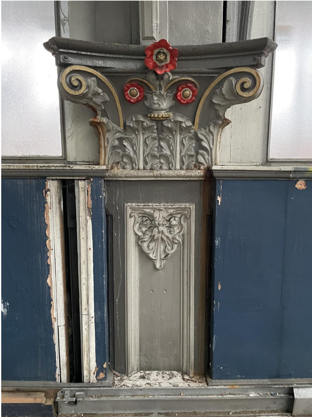
Figure 150: Detailed view of one of the external cast iron Corinthian columns to the west elevation, again featuring the “Lancashire rose” motif.
