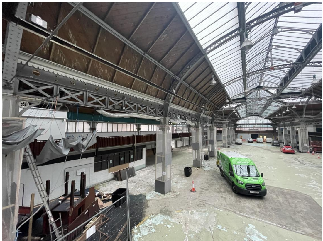
Figure 125: Looking along the southern balcony from the eastern balcony.
