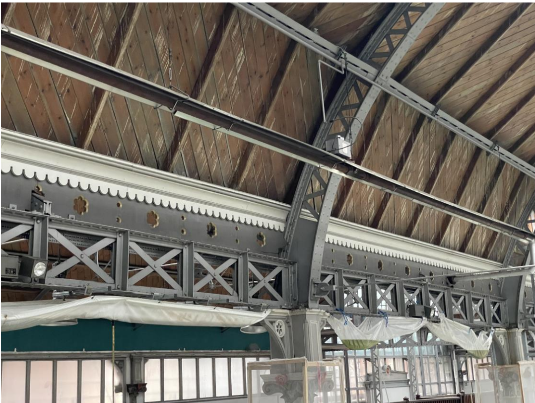
Figure 127: A detail of the original roof structure and 198-s replacement timber boarding above the southern balcony.
