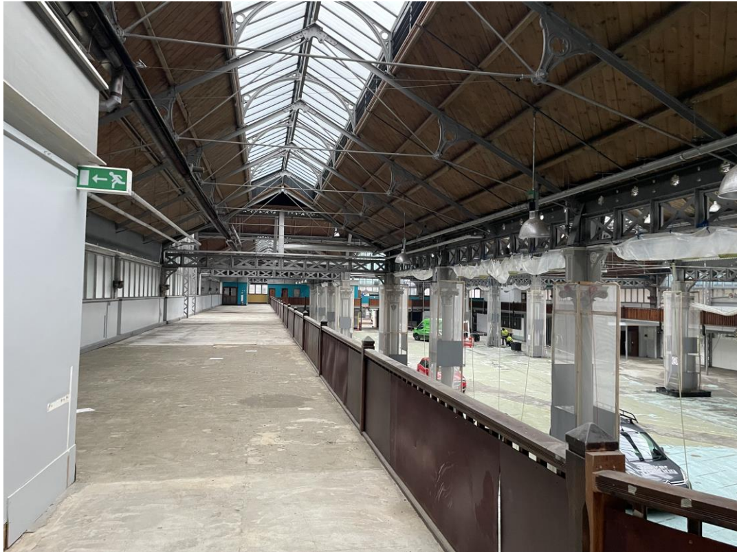
Figure 152: Looking east along the length of the northern balcony. The wall to the left forms the north-west staircase.
