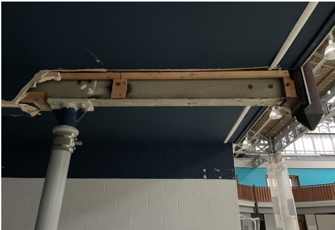
Figure 105: A detail of one of the existing columns and its connection to the cantilevered I beam
