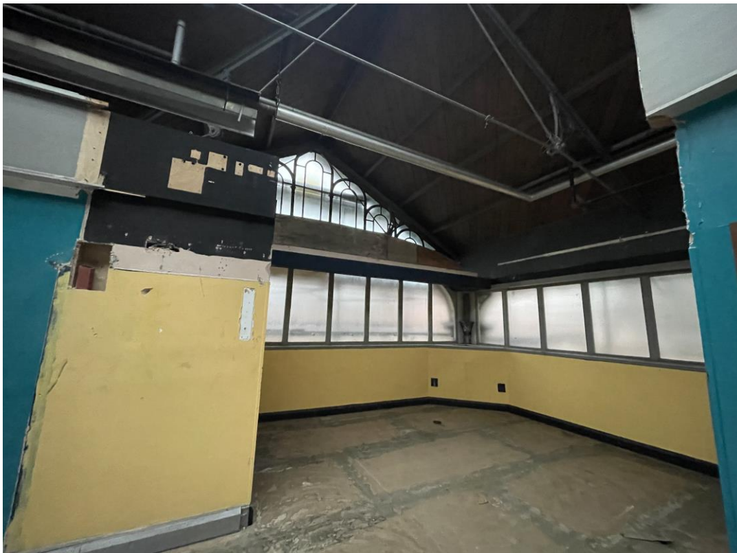
Figure 133: The north-east corner of the balcony as seen following the removal of 1980s partition walls.
