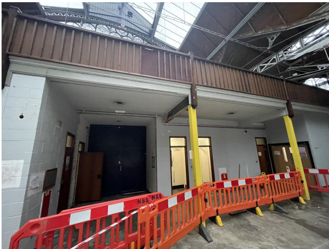
Figure 120: Looking west towards the current entrance in the centre of the west elevation.
