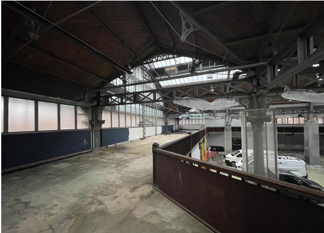
Figure 145: Looking north along the western balcony from the south-west corner.
