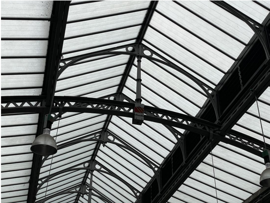
Figure 128: A view of the central, raised section of the roof, showing its recent refurbishment, which included new glazing and redecoration.
