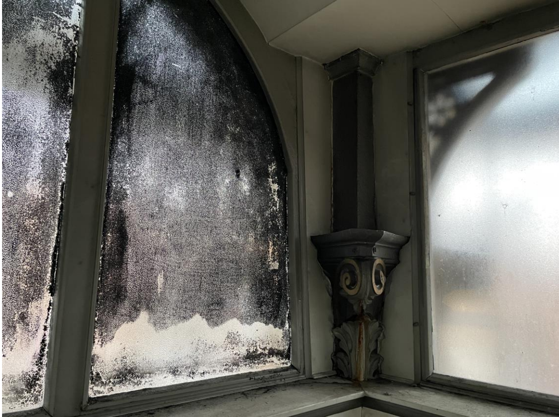
Figure 147: Detailed view of the corner of the original cast iron frame in the former cleaner's room.
