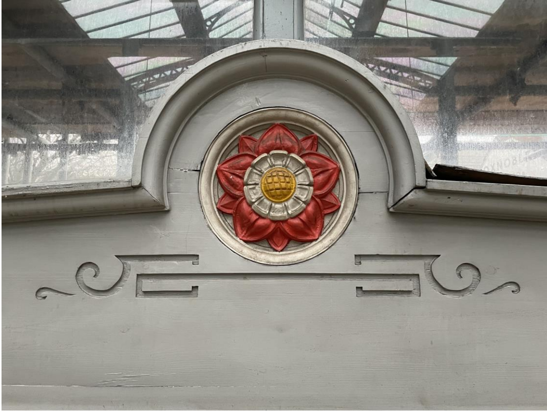
Figure 143: Close up view of the cast iron “Lancashire rose” decoration above the original south entrance.
