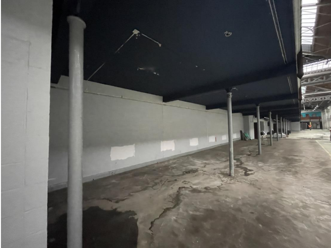
Figure 104: Looking north-east along the underside of the north balcony, showing the remaining, simple cast iron columns.
