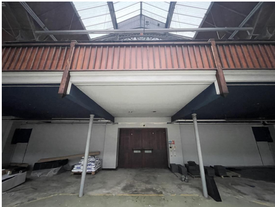
Figure 103: The original central entranceway to the centre of the north elevation.
