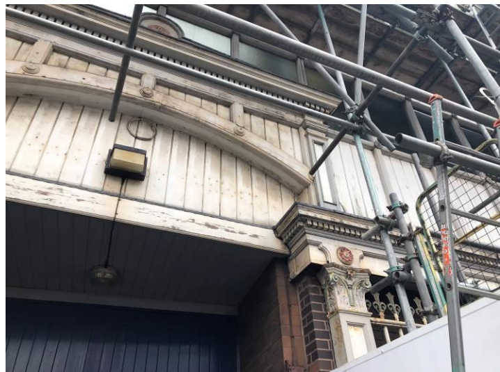
Figure 95: The lower parts of the west elevation. (2023)
