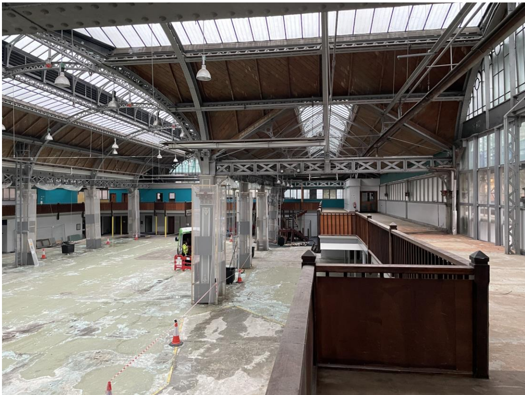
Figure 144: A view looking south along the western balcony.
