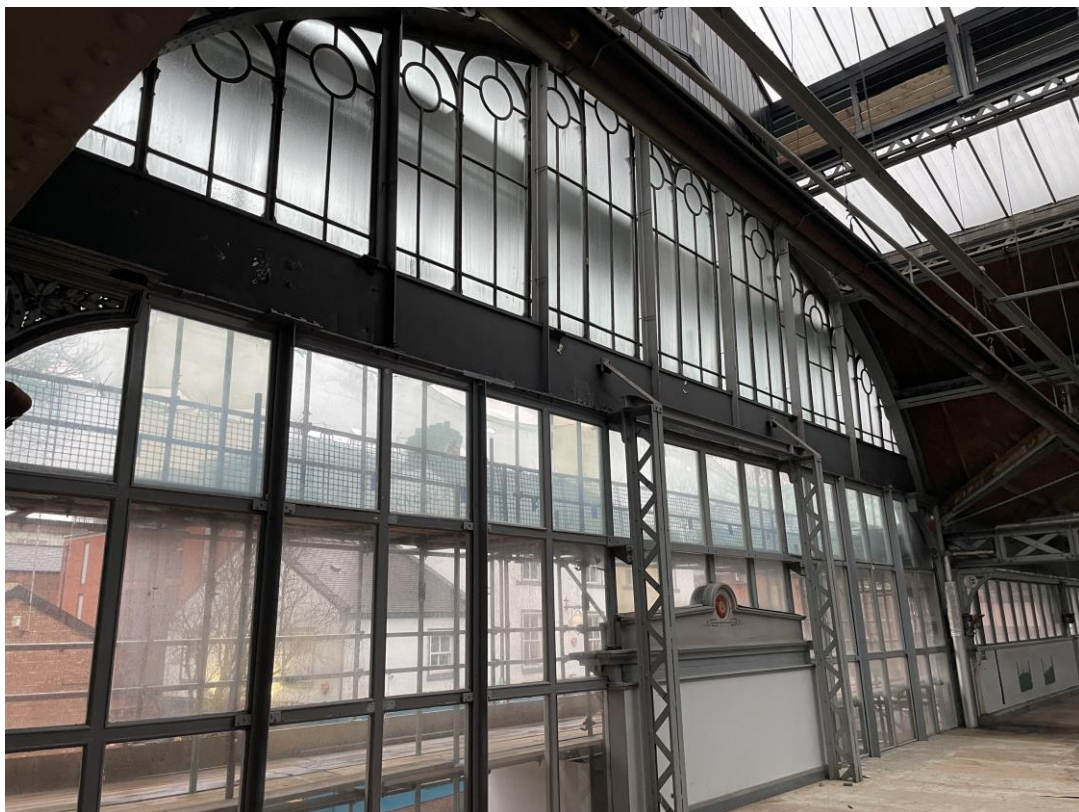
Figure 140: A view of the central glazed gable to the south elevation (Liverpool Road, showing the iron lattice supports for the original iron gates (since removed)).
