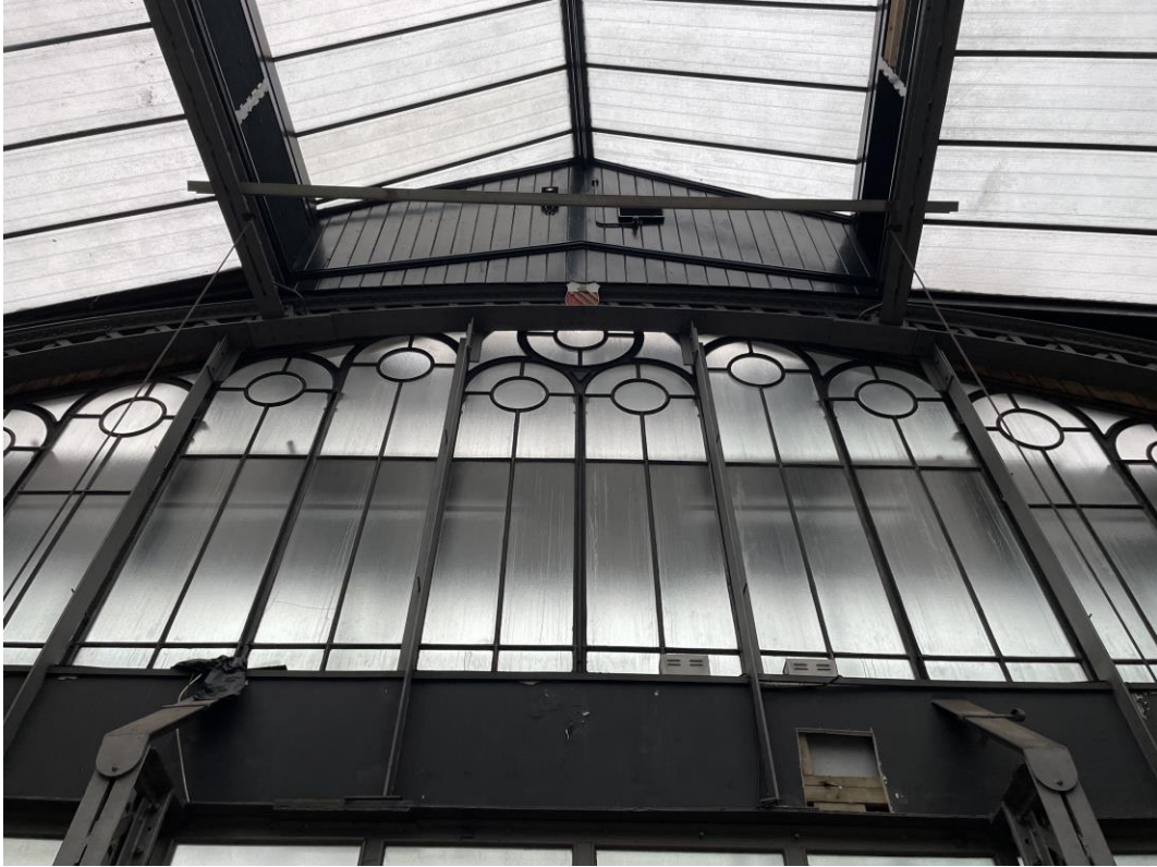
Figure 149: A view looking up at the glazed gable to the middle of the west elevation, showing the tops of the two original lattice gate supports to the bottom.
