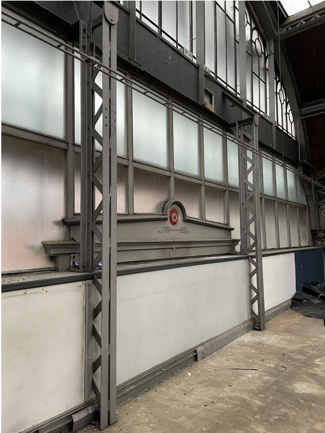
Figure 151: The central west glazed gable and former gate supports.
