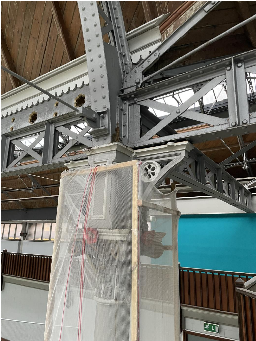
Figure 137: Detail of one of the original cast iron Corinthian columns to the north-east corner.
