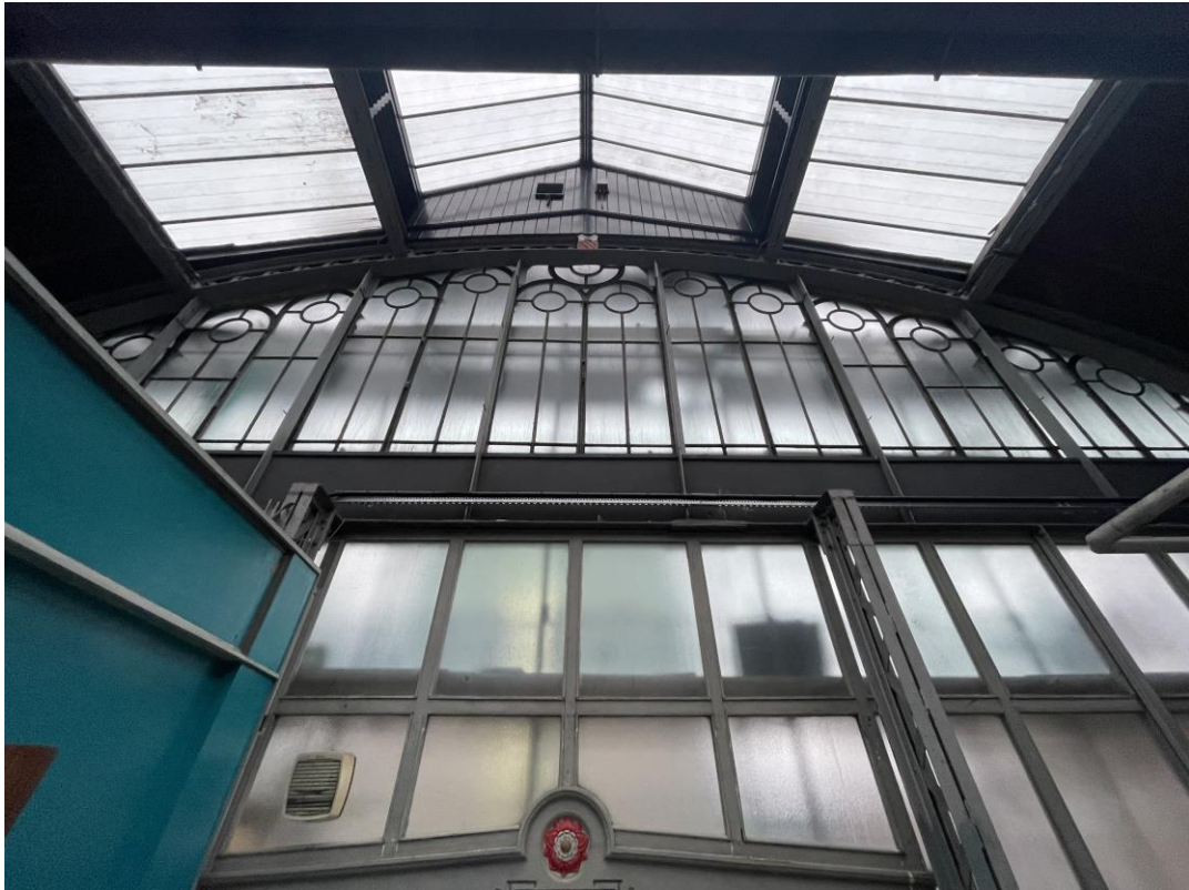
Figure 130: The central glazed gable to the east elevation. This area of the balcony was used during the c1930s-50s (and possibly before and after) as the Hall's restaurant.
