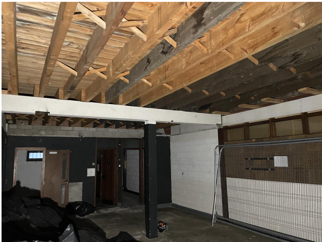
Figure 111: A view looking south into the 1980s rooms to the south-east corner of the building, showing a number of earlier joists/floorboards that formed part of the earlier balcony.
