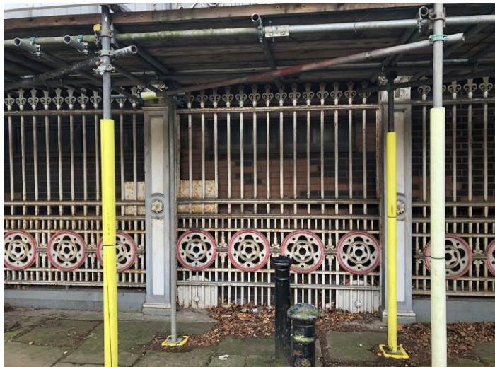
Figure 83-84: Examples of the original sliding gates to the north elevation. Note the wheels (bottom) and lock protection plates (centre) (2023).
