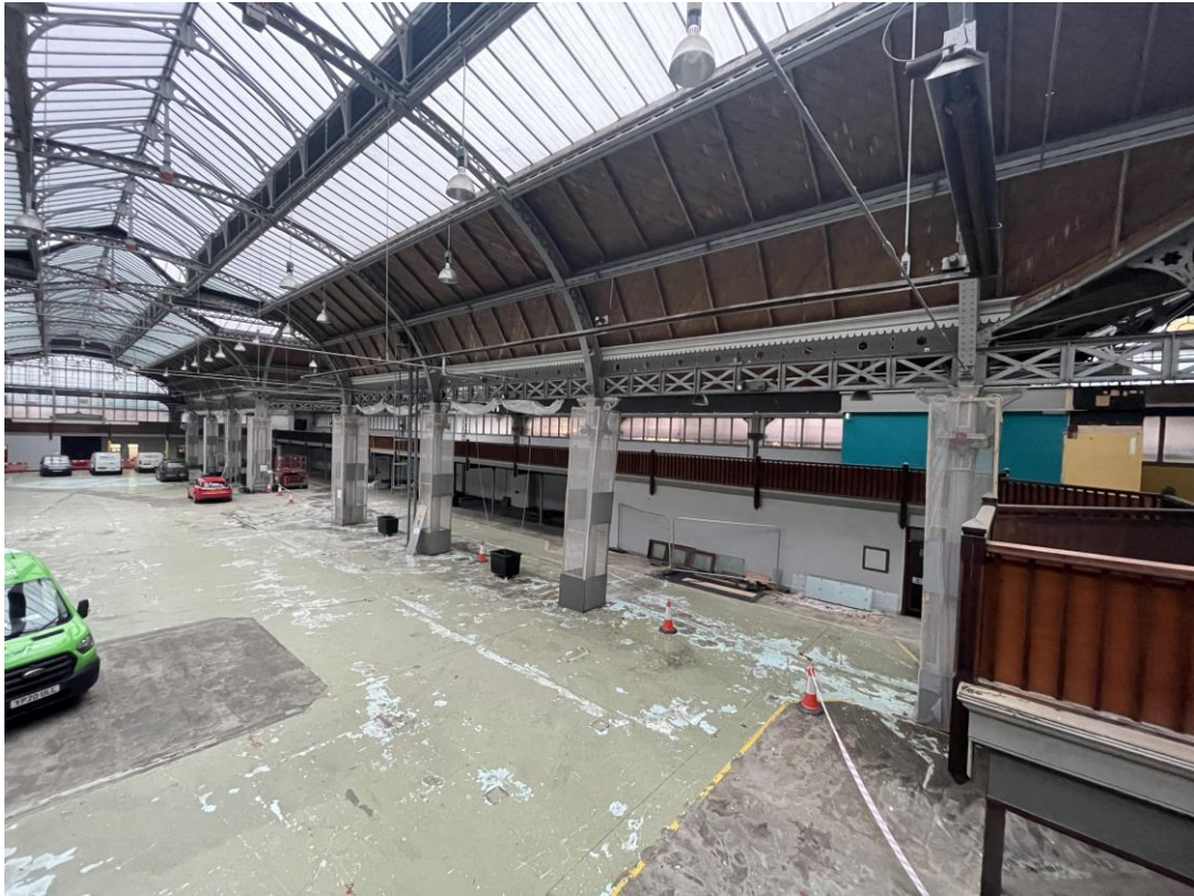
Figure 126: Looking along the northern balcony from the eastern balcony.
