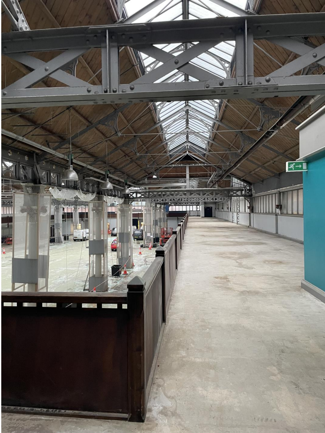
Figure 136: A view looking west along the northern balcony from the eastern end, showing the 1980s varnished timber balustrading. .
