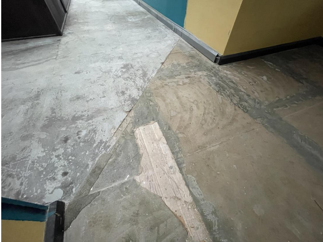
Figure 134: Looking down at the floor in the north-east corner, showing the modern screed and floorboards underneath.
