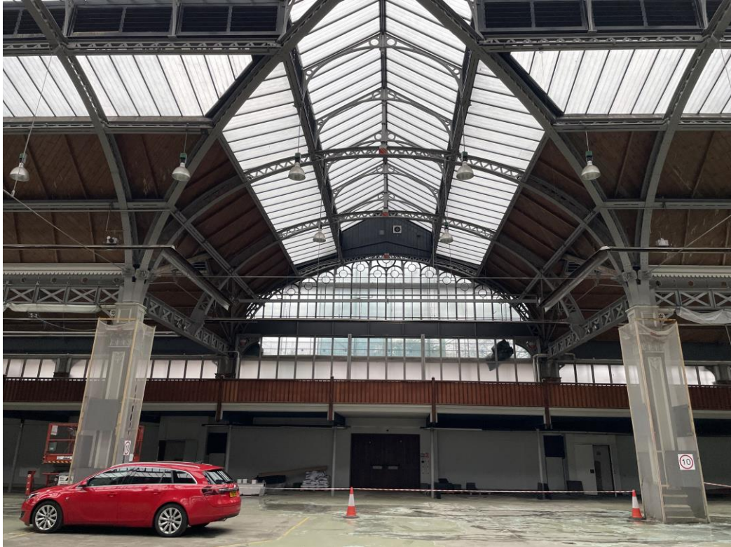
Figure 119: Looking north towards the centre of the north elevation.
