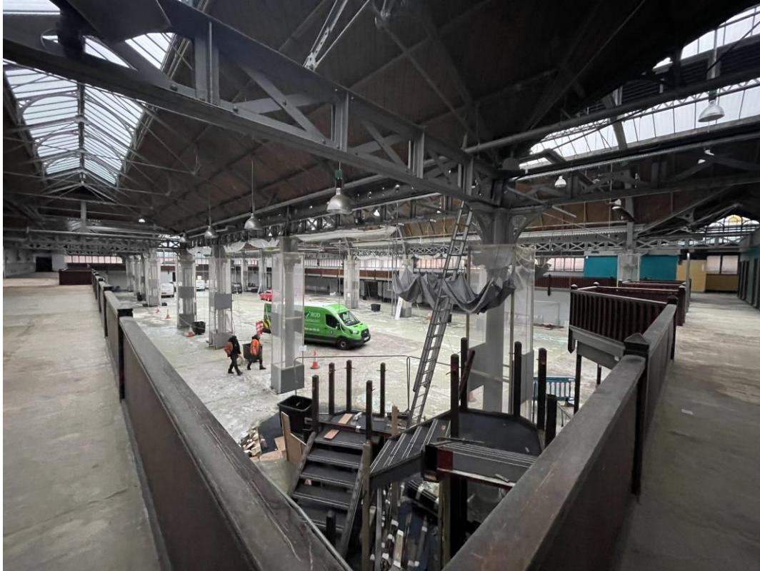
Figure 139: Looking diagonally north-west across the building from the south-east corner of the balcony.
