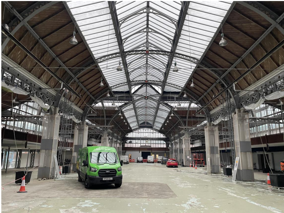
Figure 100: Looking west across the centre of the building.
