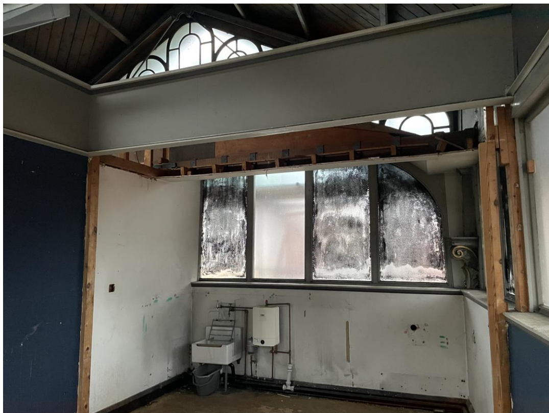
Figure 146: Looking into the south-west corner of the balcony, which as part of the 1980s scheme was used as a cleaner's room.
