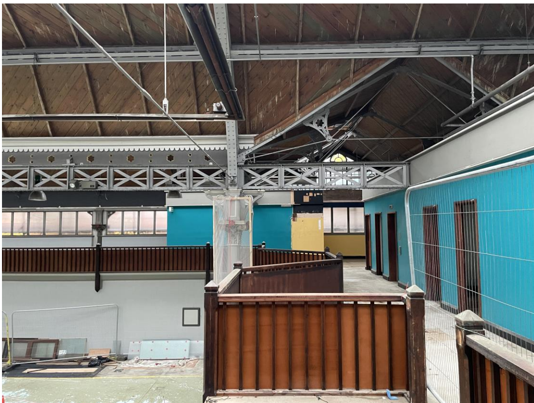
Figure 129: Looking north along the eastern balcony, showing the 1980s rooms to the right.
