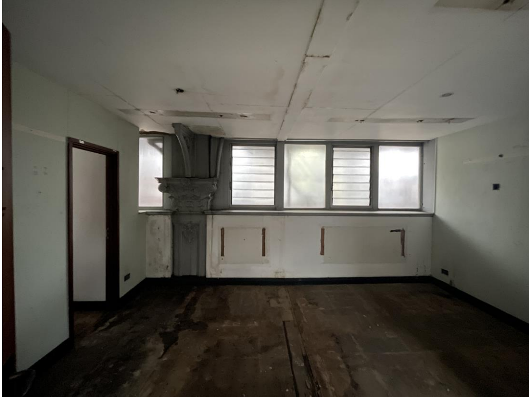
Figure 132: Looking into one of the 1980s rooms to the north-east corner of the east balcony.
