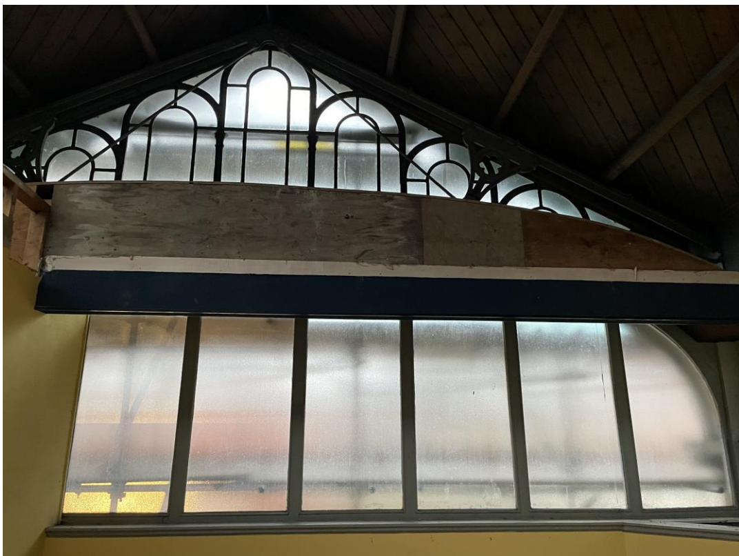
Figure 135: A closer view of the glazed gable to the north-east corner, overlooking Tonman Street.
