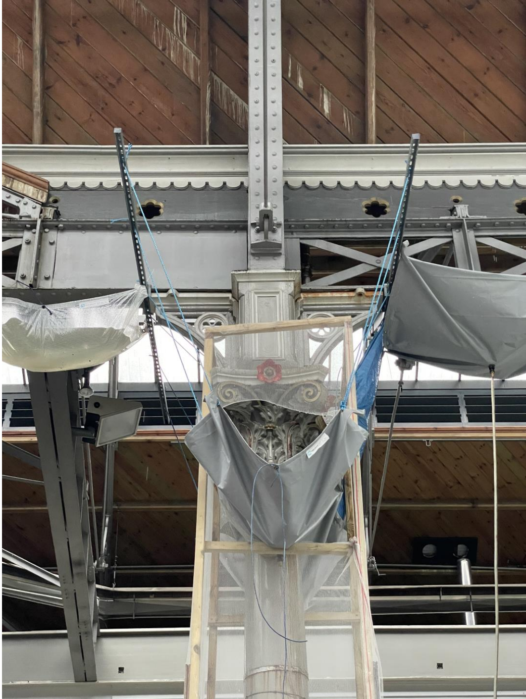
Figure 121: Detail of one of the Corinthian cast iron columns.
