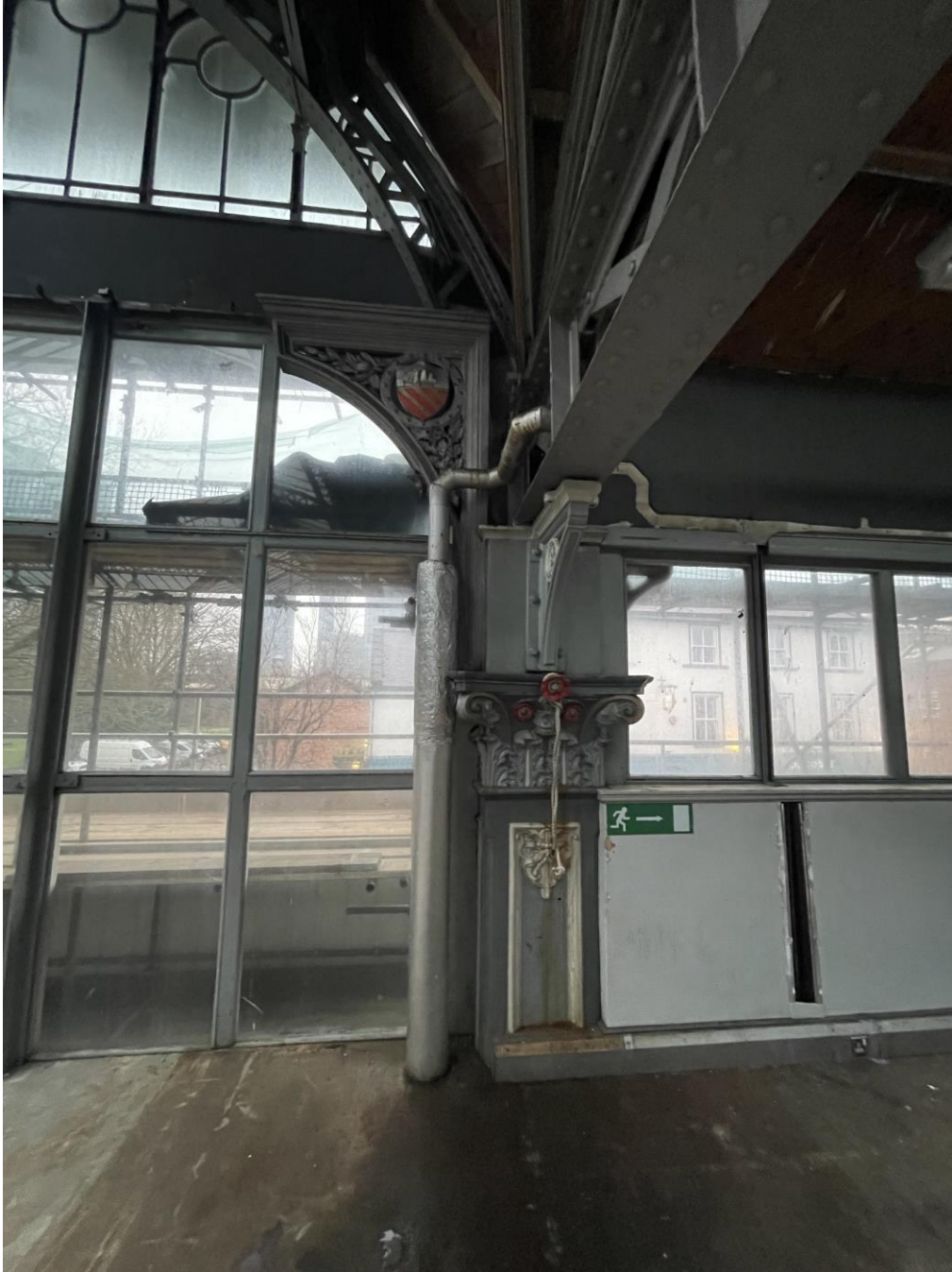
Figure 142: Detail of the external cast iron column to the west of the gable.
