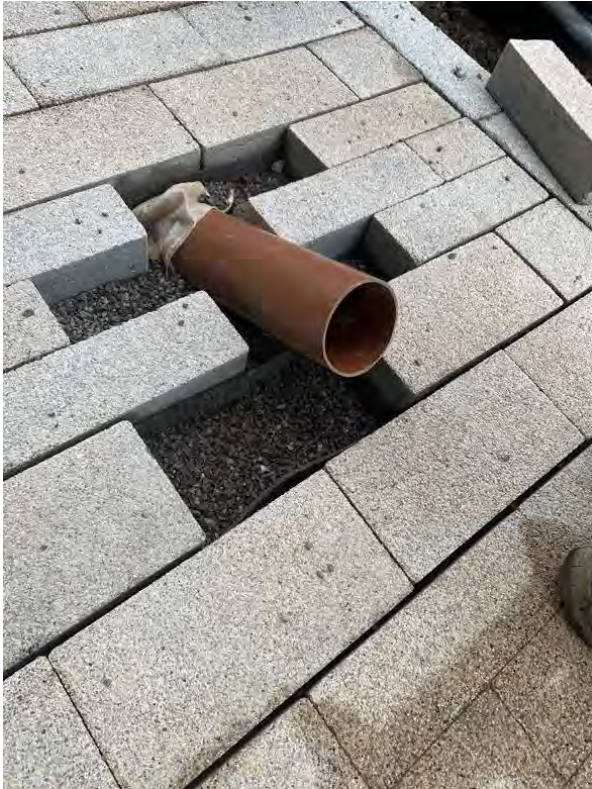
Figure 7 – Permeable Paving Installation
