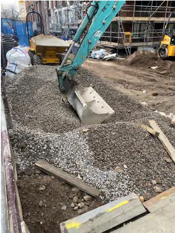
Figure 8 – Permeable Paving Installation
