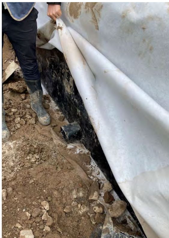
Figure 3 – Attenuation Tank Installation
