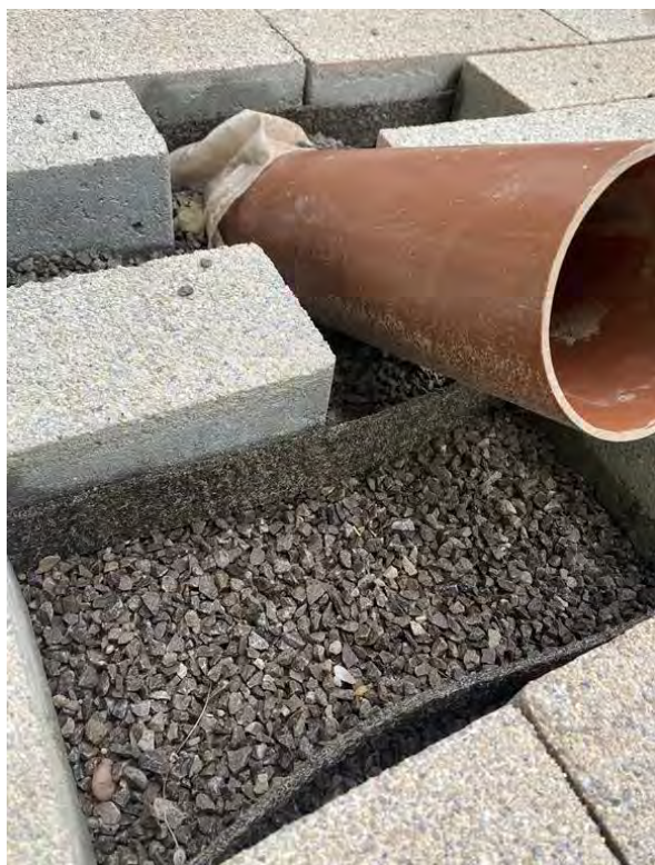
Figure 7 – Permeable Paving Installation
