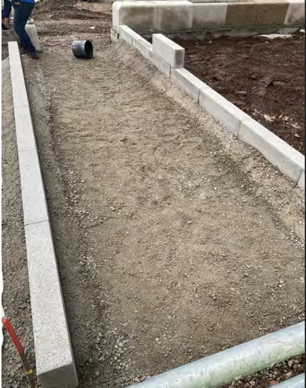
Figure 5 – Permeable Paving Installation
