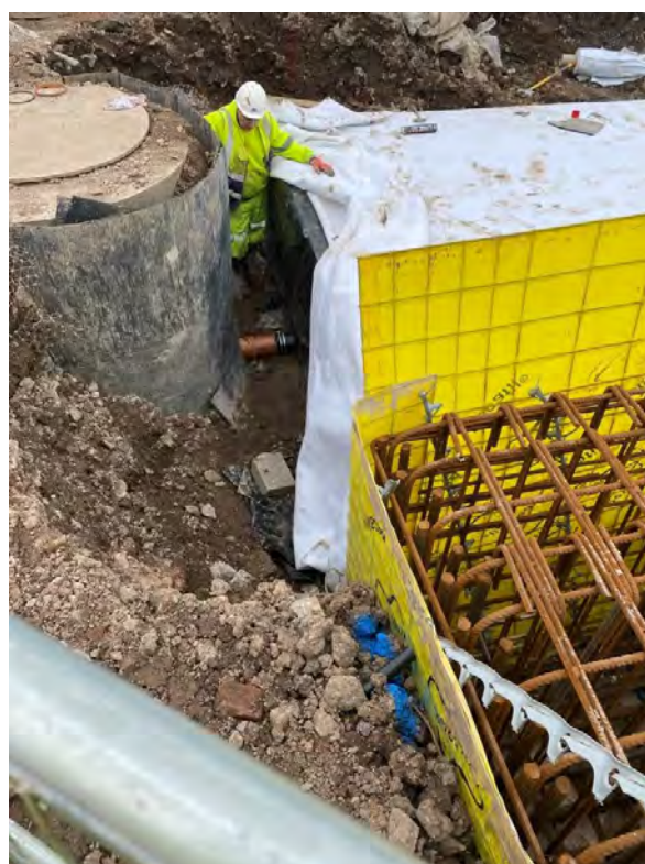
Figure 2 – Attenuation Tank Installation
