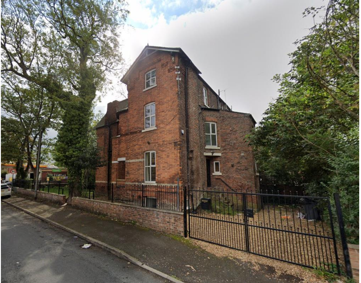
Fig.3– Imagery - The north and west elevations of the property (Source: Google Maps)
