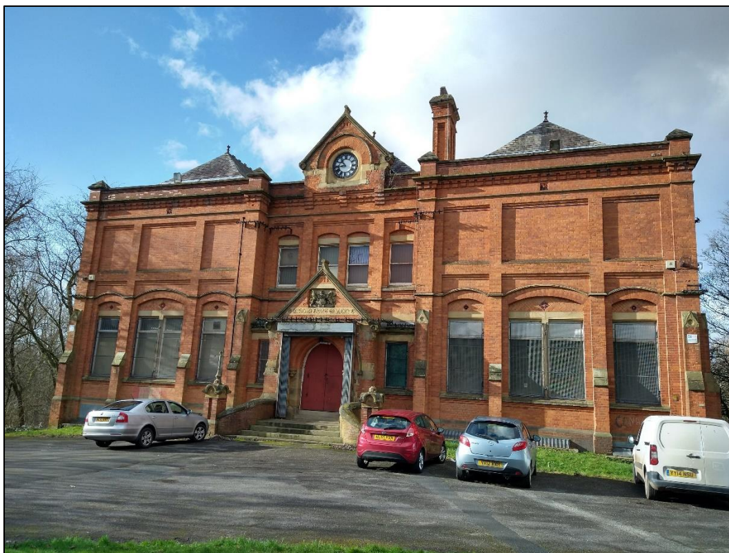
Plate 3: East façade of building.
