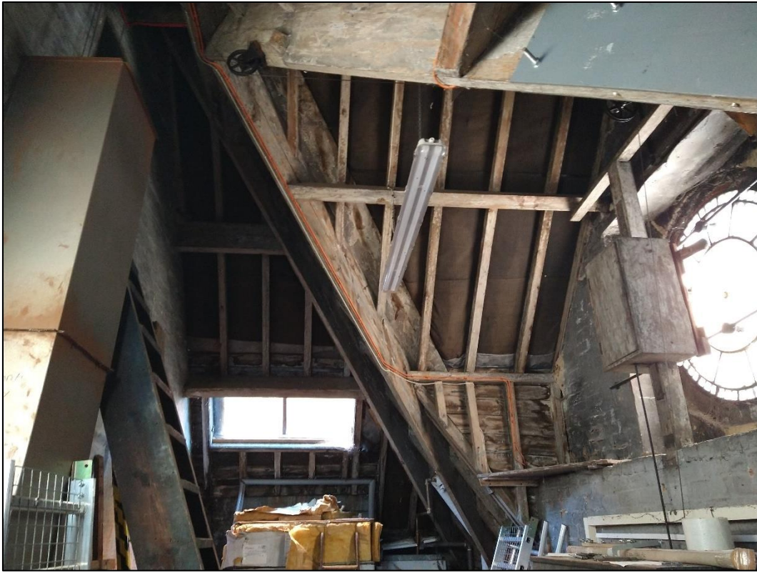
Plate 16: Interior of the clock tower, showing intact bitumen roofing felt beneath tiles, and multiple windows and the clock face creating a well-lit space.
