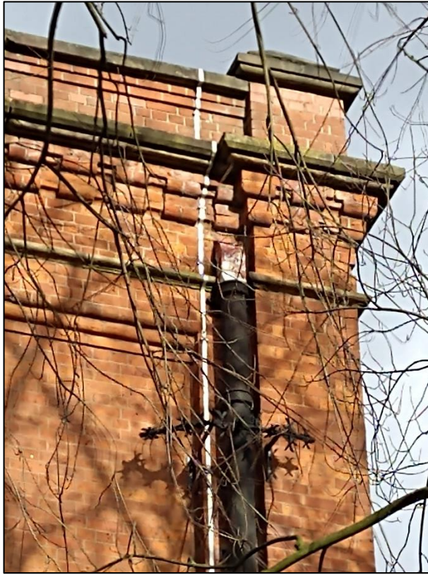
Plate 10: Location of possible bird nest in a gap by the top of a drainpipe, on the south-east elevation.
