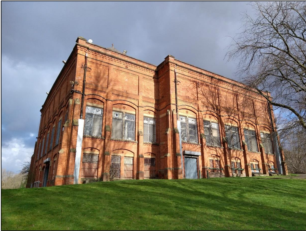
Plate 4: South façade of building.
