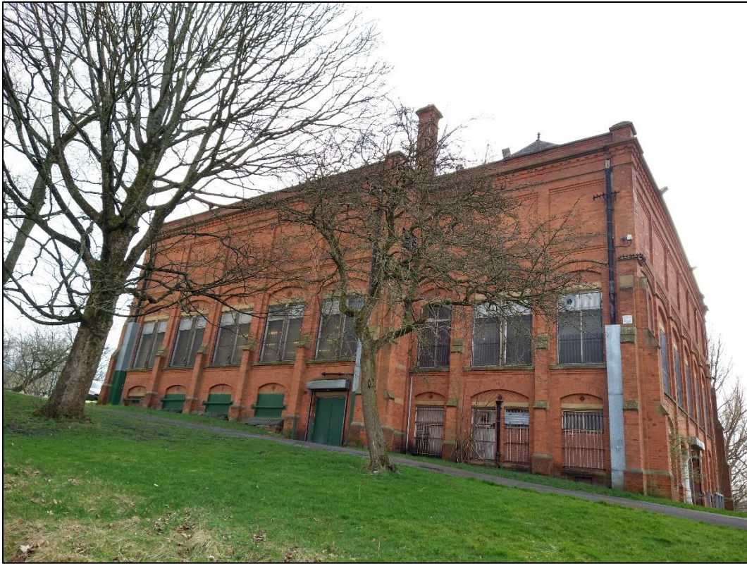
Plate 6: Northern façade of building, showing semi-sunken basement level and sloping footprint.
