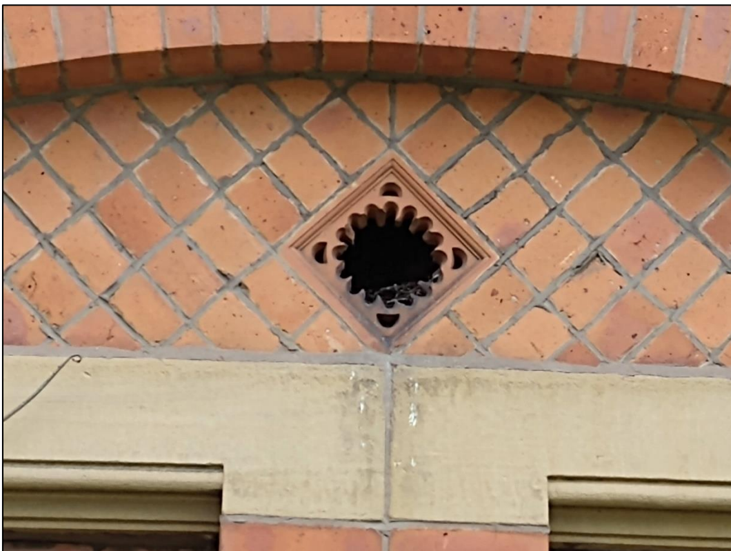
Plate 9: Decorative air vent with broken spokes. An old birds nest is observable within the hole.
