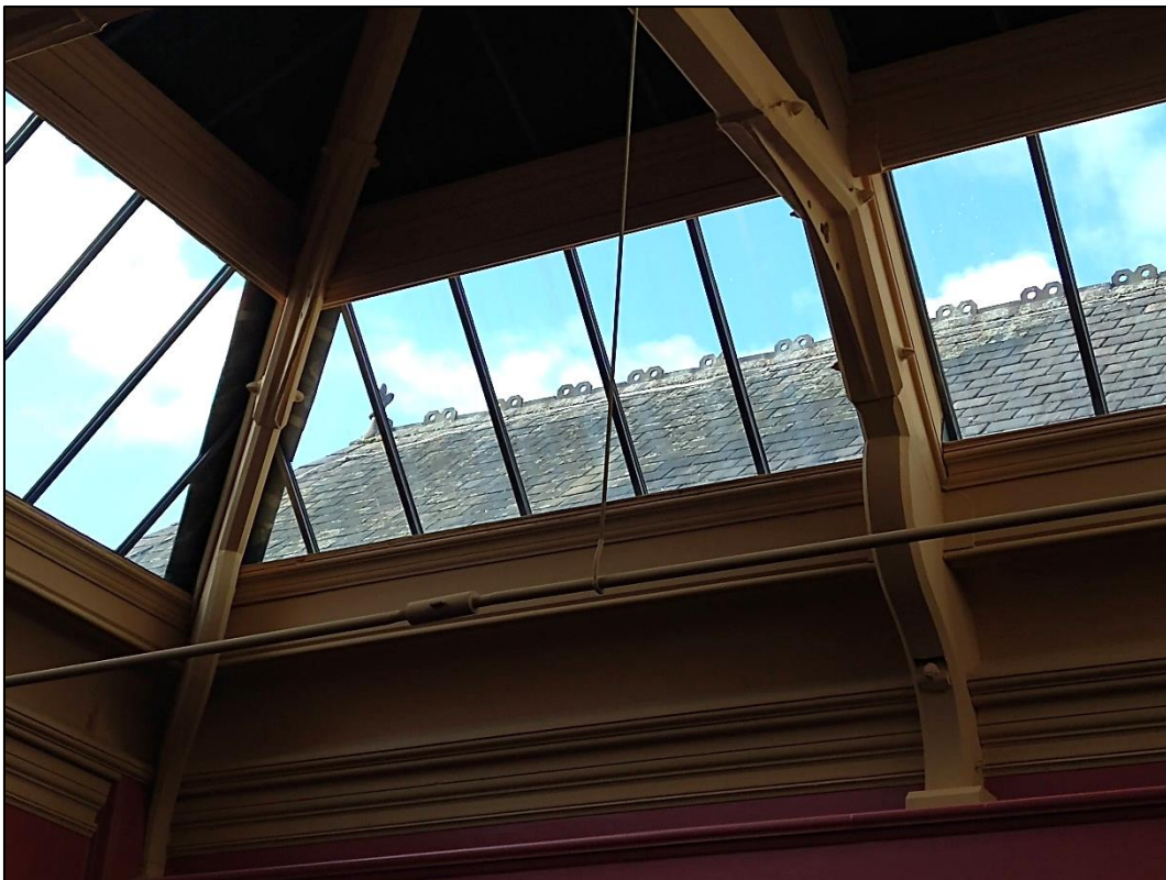
Plate 23: View through internal glass roof structure, toward internal ridgeline, with tiles well-fitting and in generally good condition.
