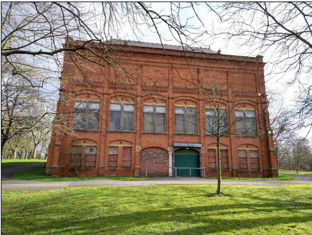
Plate 5: West façade of building, showing loading entrance into the cellar.
