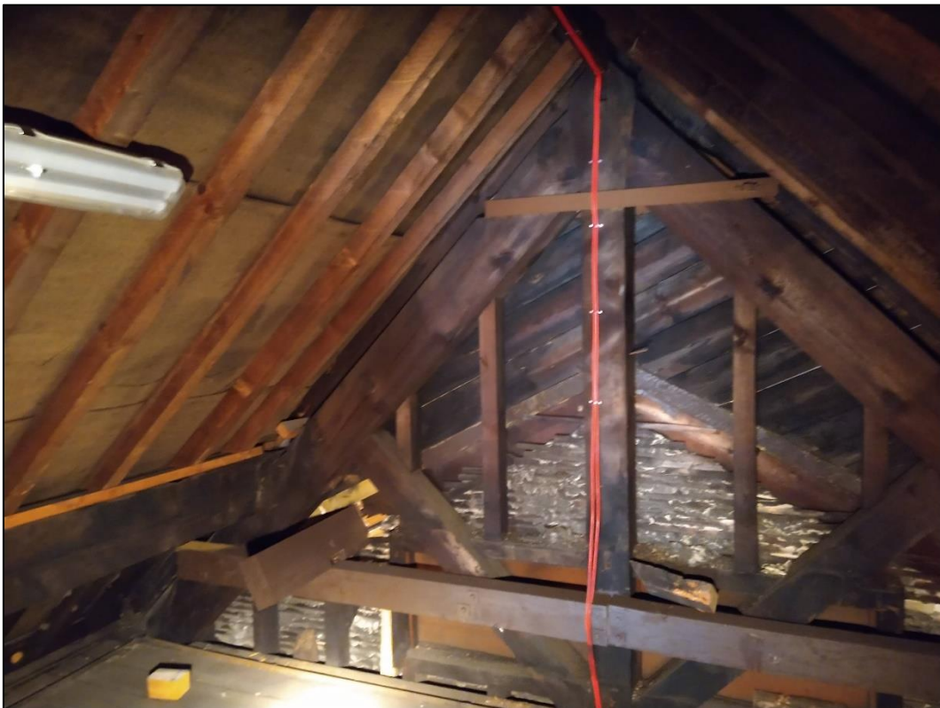
Plate 19: Interior of the central internal loft void, above the main hall, which was lined with plywood and well-sealed.
