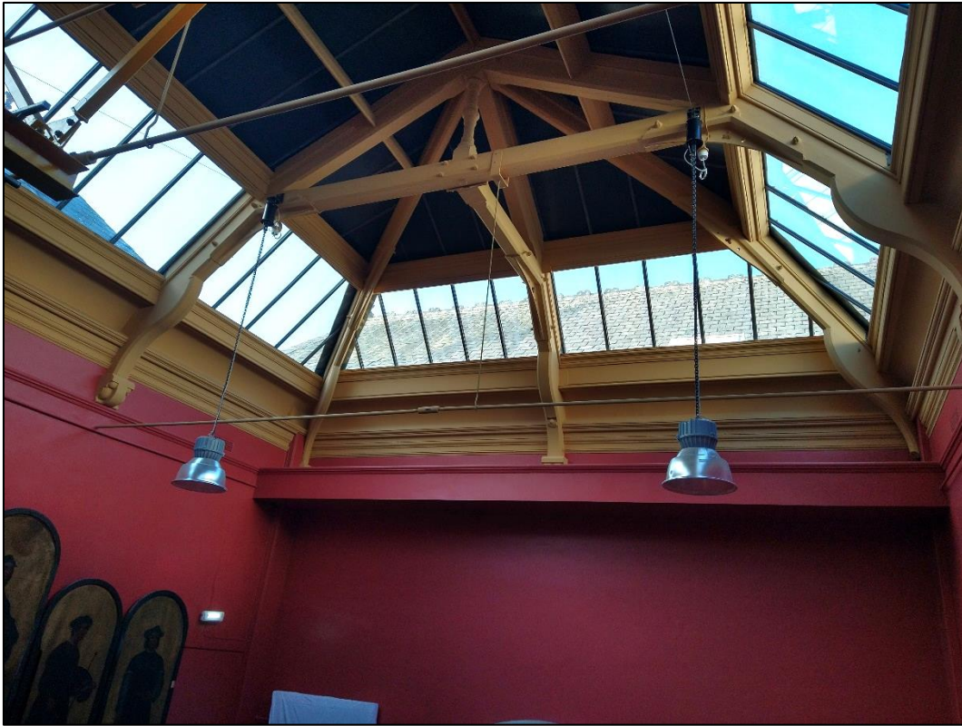
Plate 22: Main hallway within the building, with internal roof ridges visible through the glass roof.
