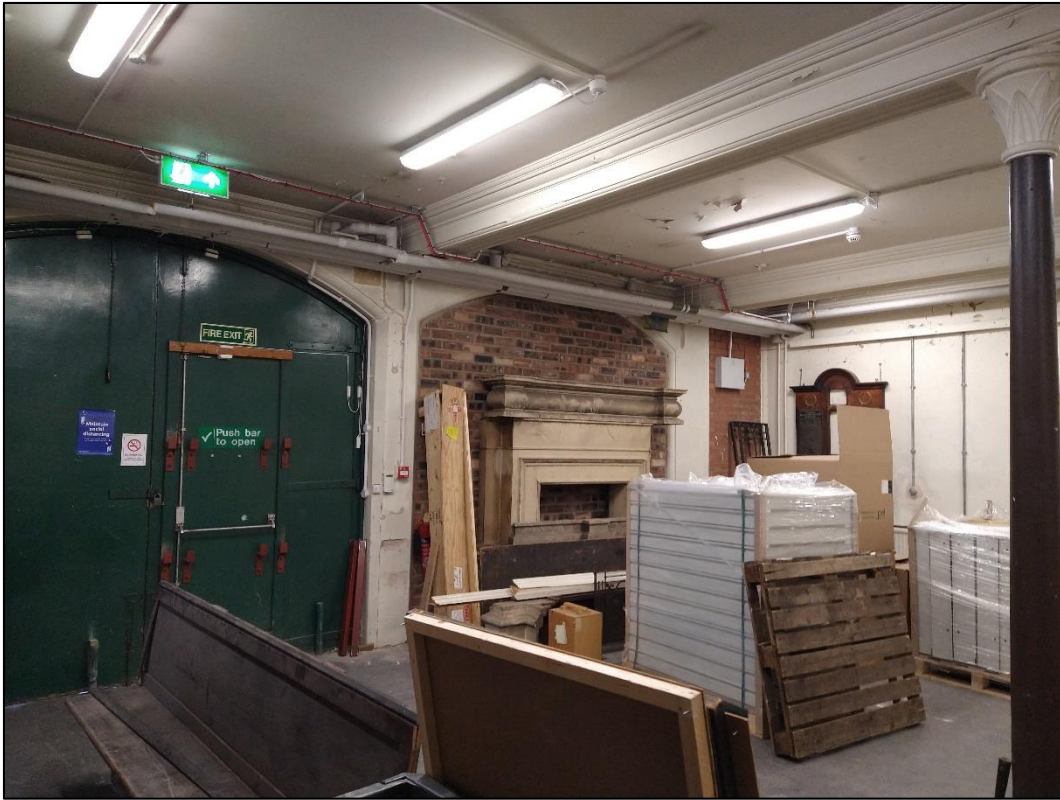
Plate 26: Example of internal basement space, showing the large loading bay doors on the western side of the building, which were well sealed around the frame.
