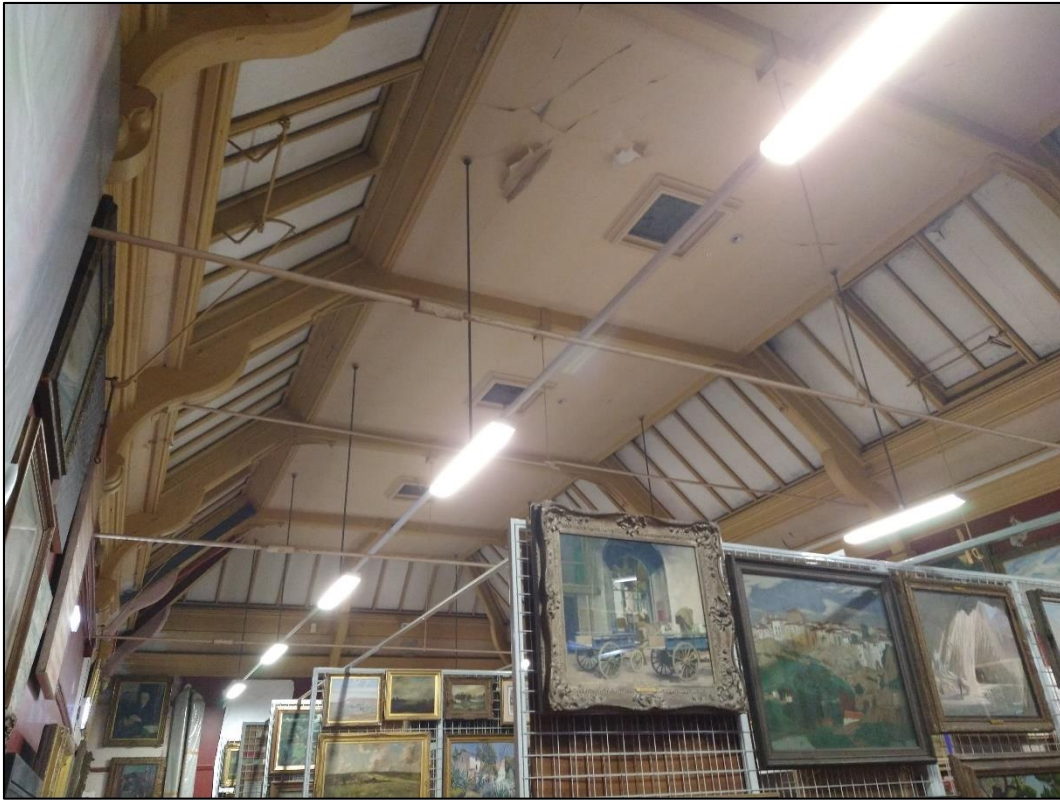
Plate 14: Example of Internal roof structure, showing the south wing, with an inaccessible internal roof void, with metal shuttered skylights around the edges.
