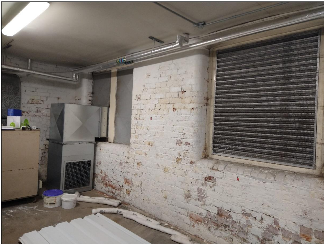
Plate 25: View of shutters present within the plant roof, which were well sealed and in good condition, with no gaps large enough for bats to gain entry.
