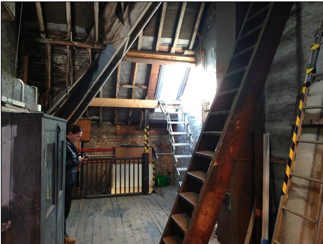
Plate 17: Alternative view of interior of the clock tower, showing wooden access stairs to the roof void above the main hall to the right, and metal stairs to the roof access straight ahead.
