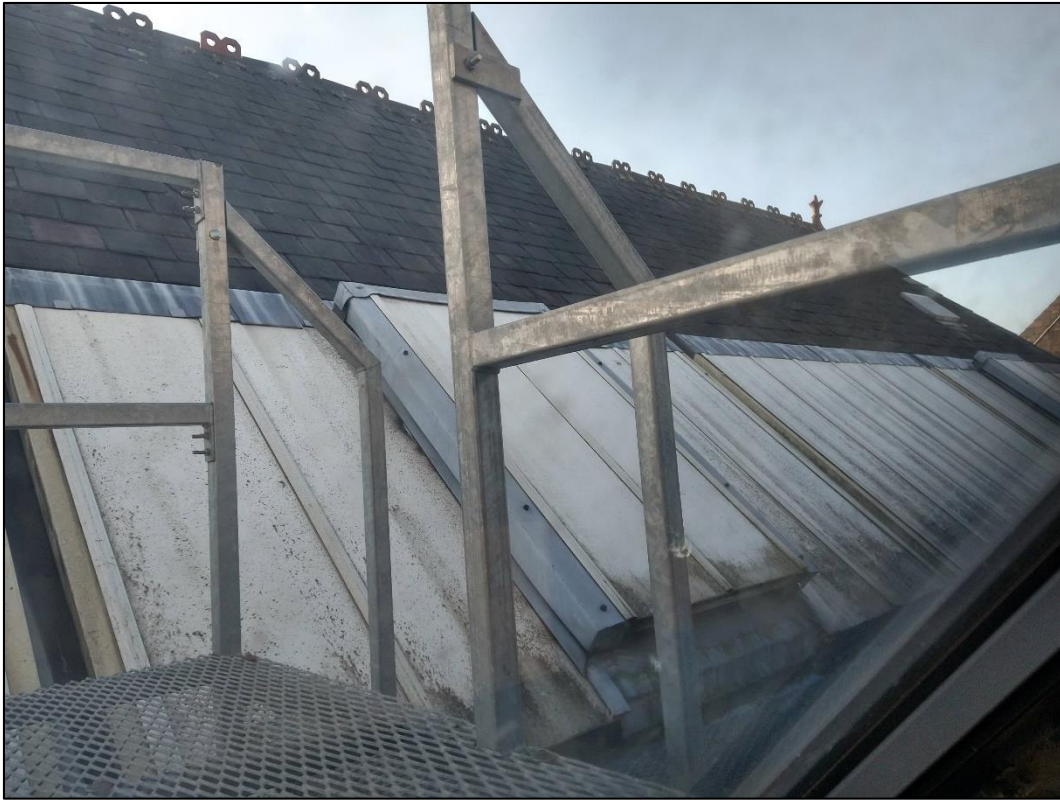
Plate 18: View through the roof access hatch, showing metal covered skylights with lead flashing on the interior of the southern ridge line. The roof could not be accessed during the survey.
