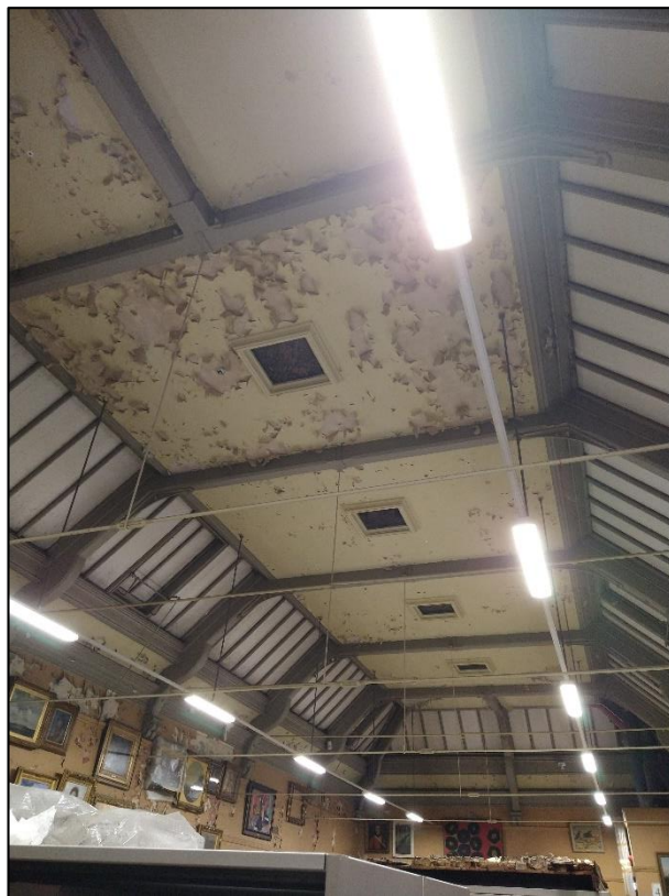
Plate 15: Example of internal roof structure, with inaccessible roof void and metal shuttered skylights, within the west wing.
