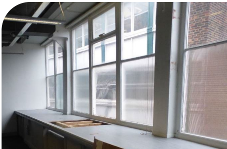
Fig 2. Single glazing to East elevation
