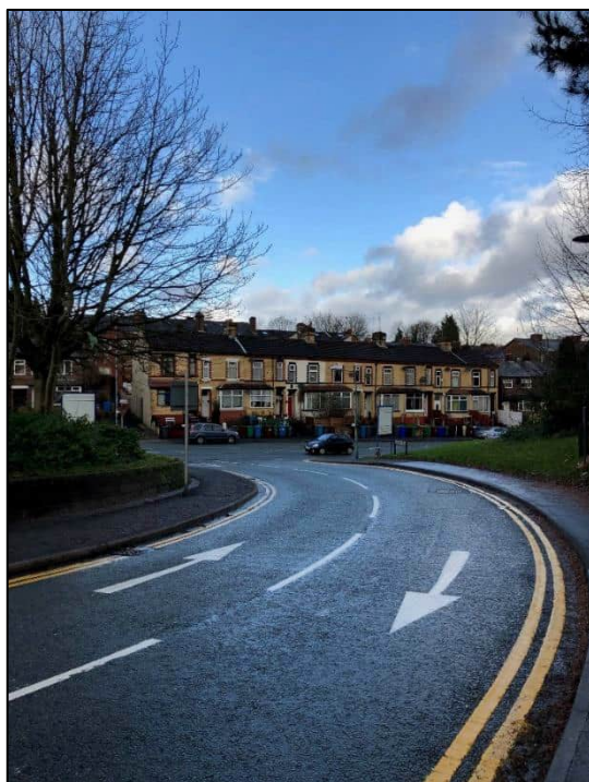
Figure 3.6 (left) – Site Access off Delaunays Road (Crumpsall Way)
